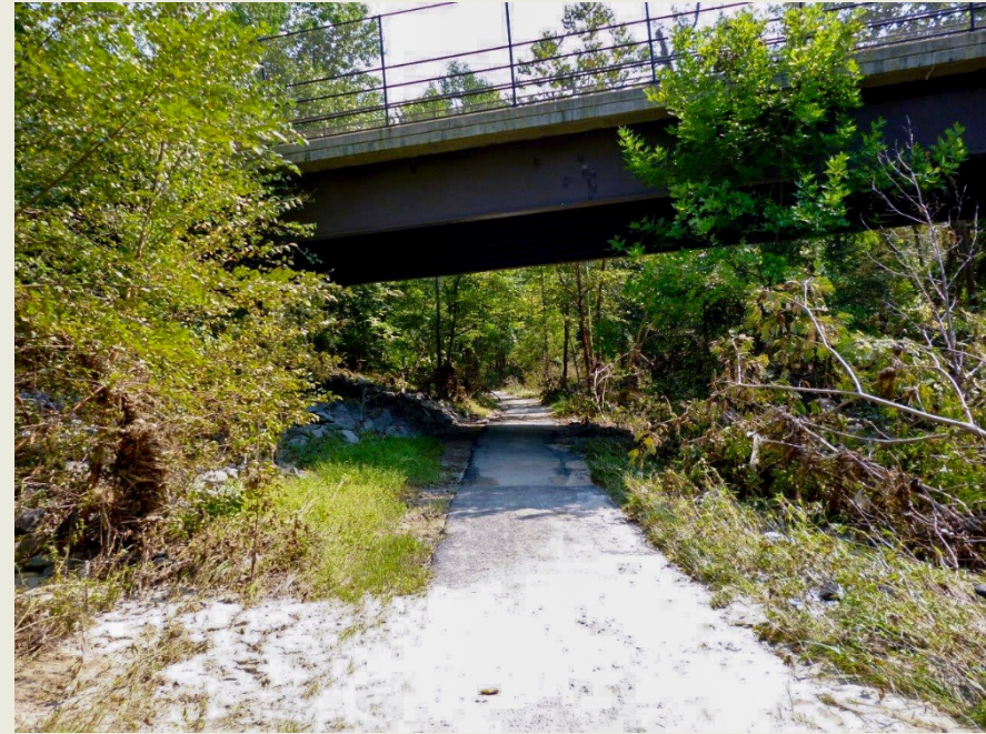
Undamaged Asphalt Section Of Same Trail
