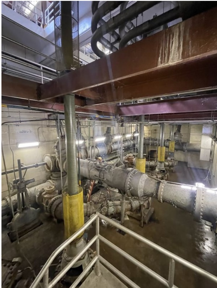
Figure 2-7: Accotink Pumping Station General Condition
