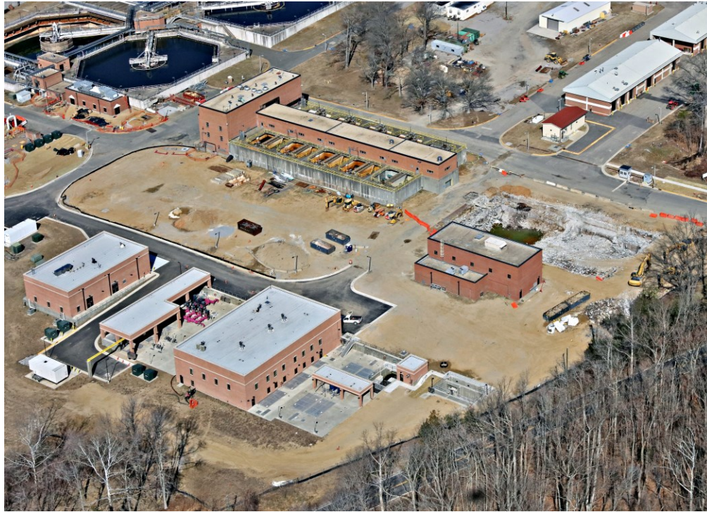
Figure 2-27: Aerial Photo of UV Disinfection Project Completed Facilities
