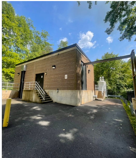
Figure 2-9: 50/66 Main Pump Station External Appearance
