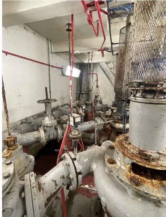
Figure 2-5: Rivertowers Pumping Station General Condition
