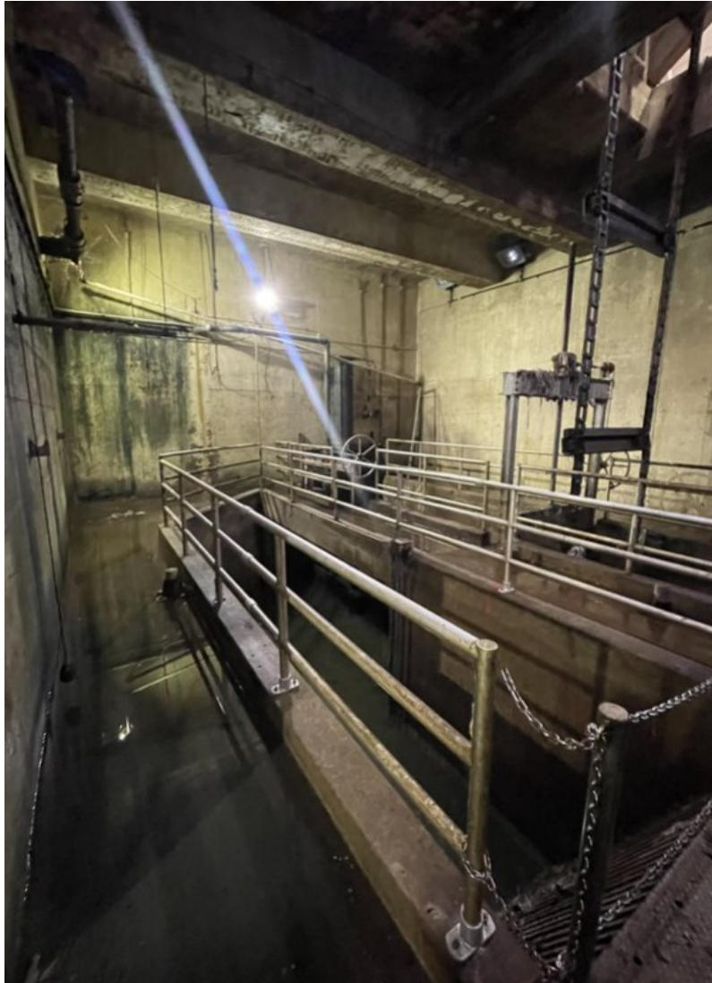
Figure 2-6: Accotink Pumping Station Wet Well General Condition
