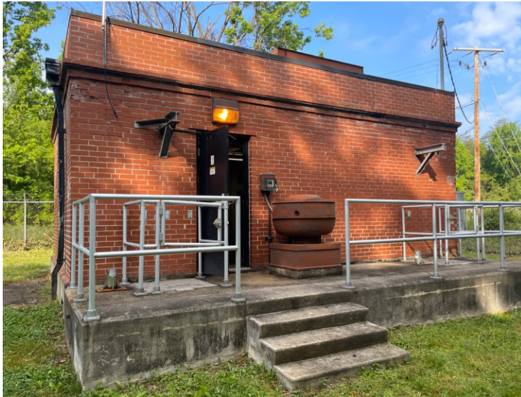
Figure 2-4: Rivertowers Pumping Station External Appearance
