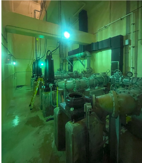
Figure 2-8: 50/66 Main Pump Station General Condition
