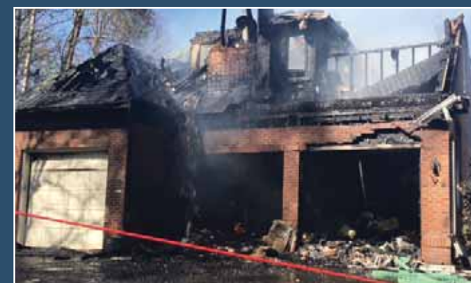
This accidental house fire in the Oakton area on March 30, 2016, was started by rags that were soaked with linseed oil that were left in a pile outside of the home. The rags spontaneously combusted and caused the fire to spread to the home. The home sustained approximately $652,500 in damages. (Top two and bottom left photos provided by Dereck Welsh, Northern Virginia Fire Buffs. Bottom right photo by Battalion Chief Willie Bailey.)
