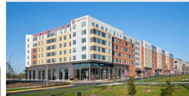
Ovation at Arrowbrook 274 Multifamily Units Dranesville District
