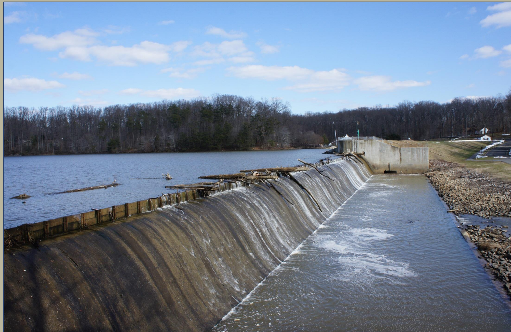
Existing Dam Spillway
