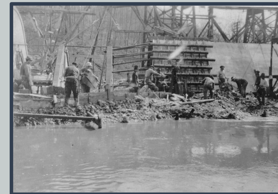
Mid-construction of the 1943 dam
