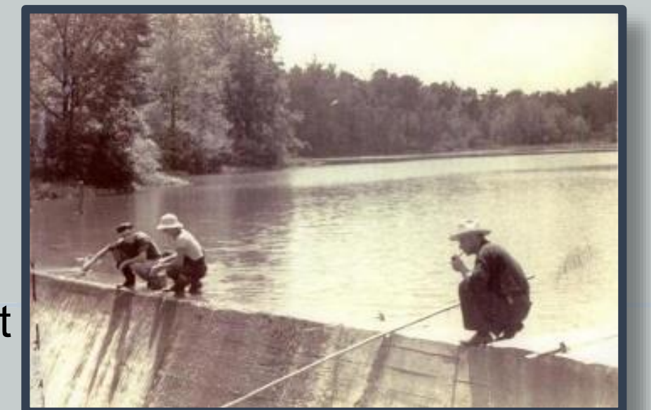
Picture of the original 1918 dam
