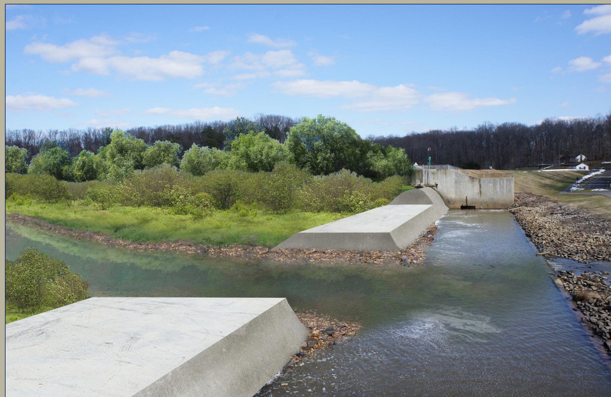
Conceptual Image of Lowered and Notched Spillway with Reclaimed, Vegetated Land Area
