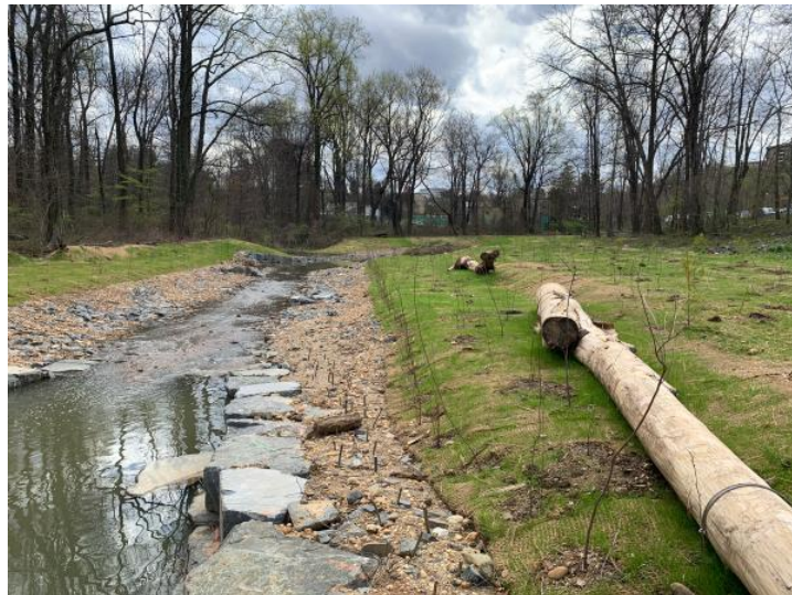
Restored Scotts Run stream channel (Picture Credit: Fairfax County Staff, April 2022)
