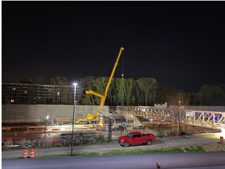
Pedestrian and bicycle bridge under construction over I-495
