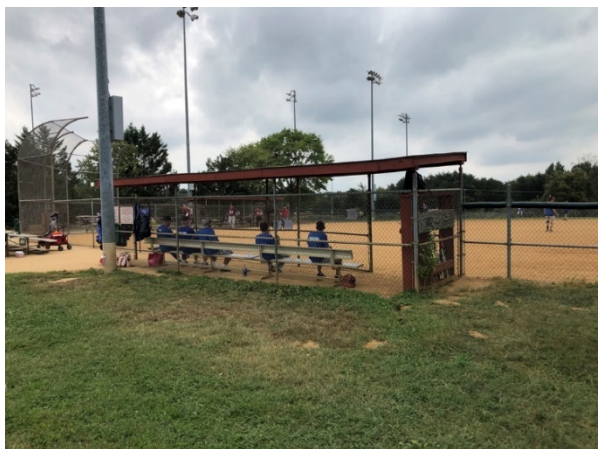
Figure 8: Braddock Park Dug Out Shelter
