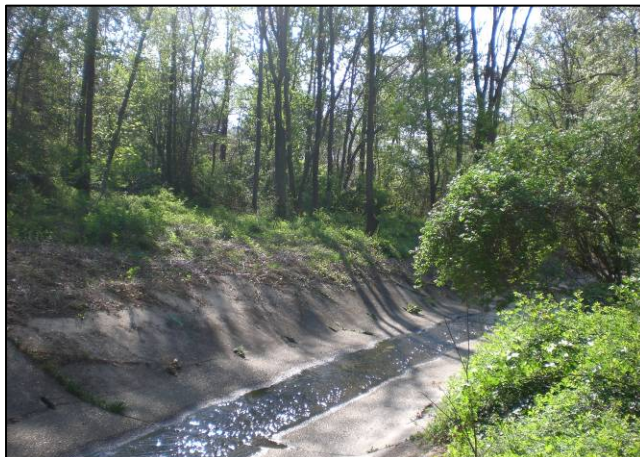
Channelized portion of Long Branch Stream
