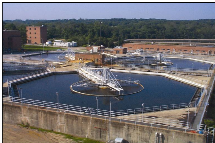
Photo of the Noman M. Cole Jr. Pollution Control Plant for wastewater treatment.
