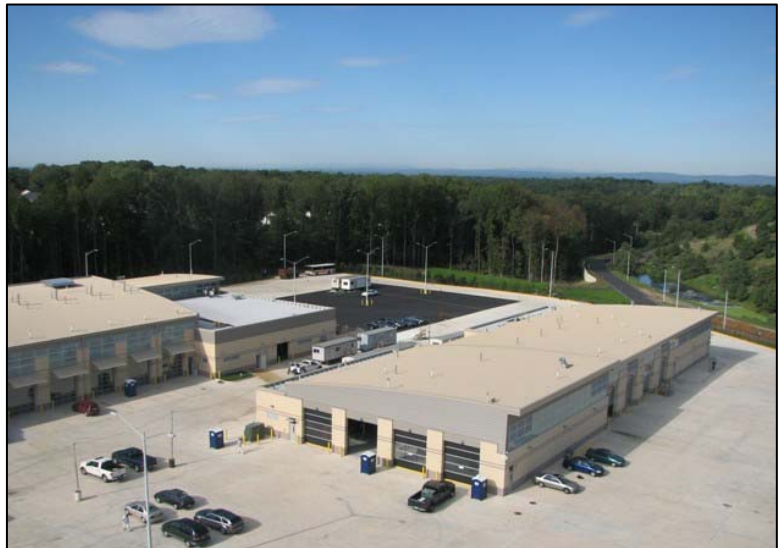
New West Ox Bus Operations Center, to commence operations in summer 2009.
