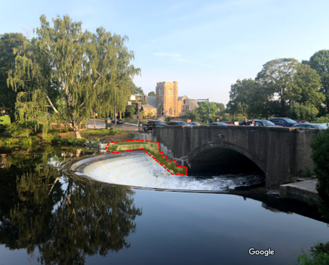
Retrofit of an existing dam. Image credit: Google / Fanuel Muindi
