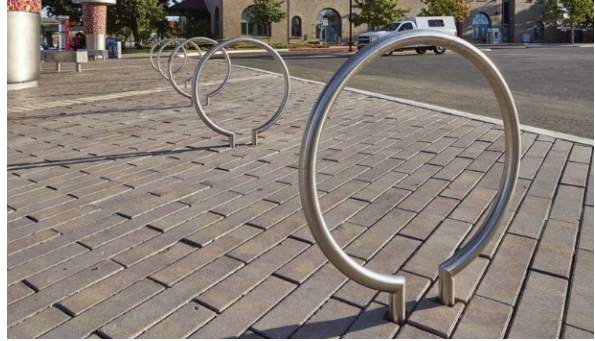
Short-term bike parking on permeable pavers example (PHOTO CREDIT: ANTHONY TERREBONNE)
