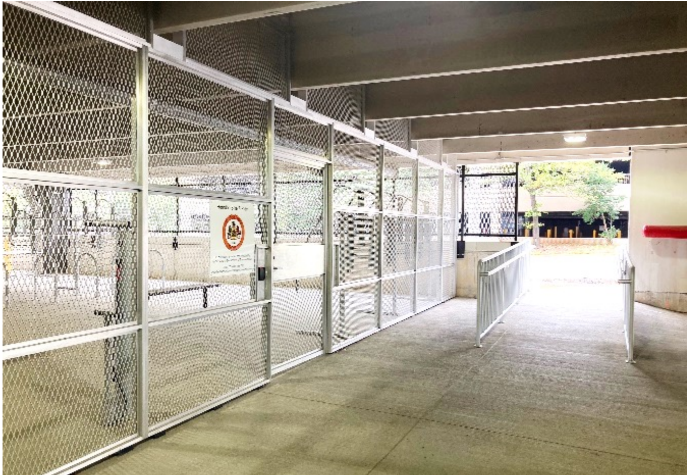
Bike room with controlled access
