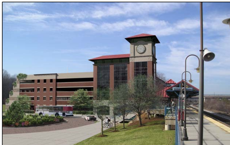
Burke Virginia Railway Express (VRE) Station.
