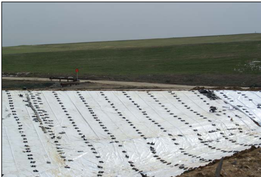
I-95 Ashfill Cell – Phase IIIA, constructed and ready for use
