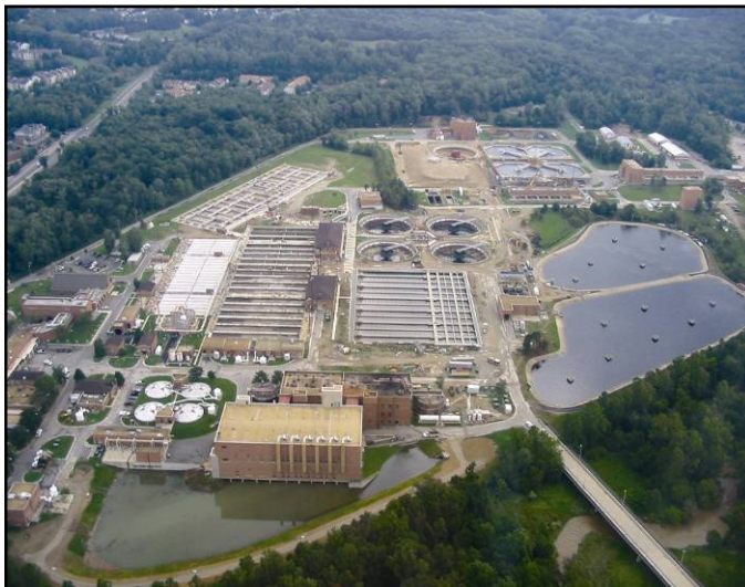
The County's wastewater treatment plant serves an estimated 364,500 households with public sewer service.
