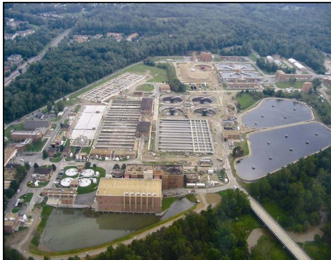
The County's wastewater treatment plant serves an estimated 365,838 households with public sewer service.
