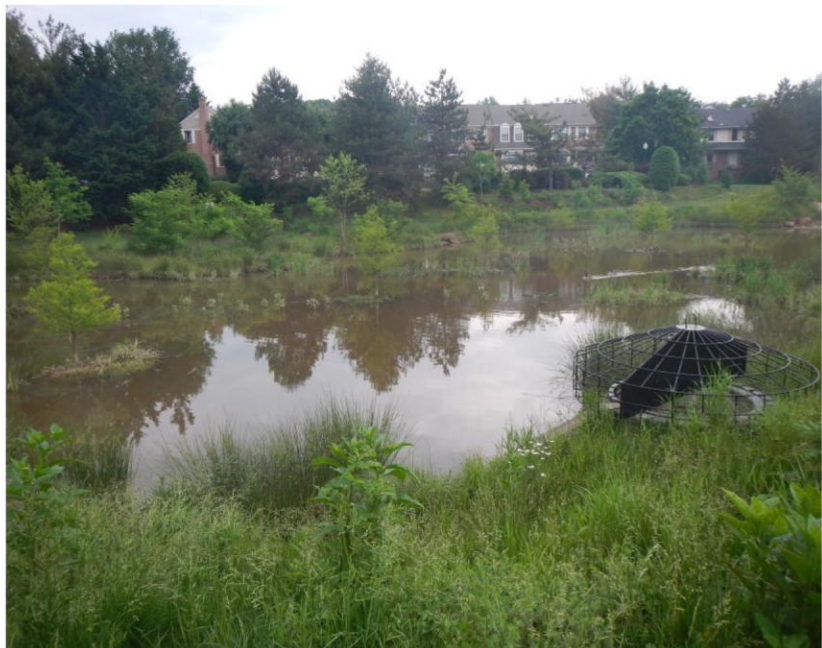
Wetland-enhanced stormwater pond retrofit
