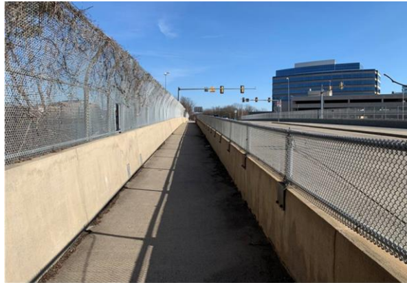
Barrier Separated Sidewalk
