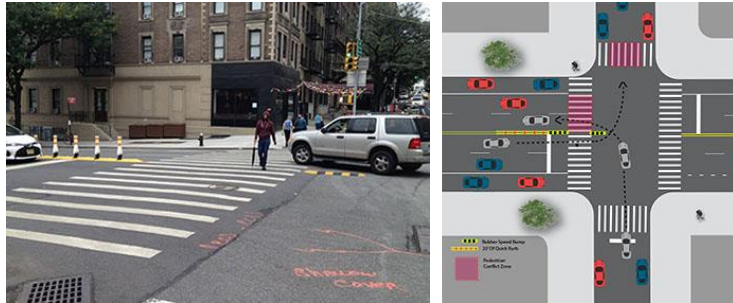
Figure 5. Low cost but effective turning barriers for left turning traffic can be installed immediately at signalized intersections (example from nyc.gov)
