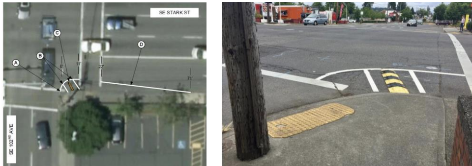
Figure 6 Low cost but effective turning barriers for right turning traffic can be installed immediately at signalized intersections (Portland.gov).
