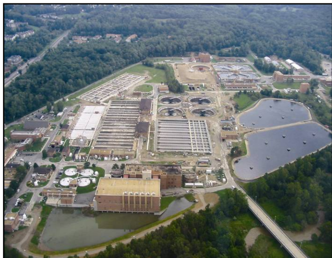
The County's wastewater treatment plant serves an estimated 355,208 households with public sewer service to help maintain a safe and caring community.
