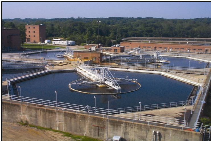
Photo of the Noman M. Cole Jr. Pollution Control Plant for wastewater treatment.
