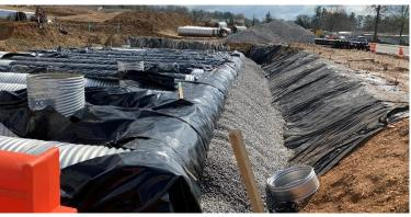
**Pictured From Top to Bottom:** Rendering of the Residences at North Hill Development; Garage slab for building 2A ready for concrete placement; Pipes in place for underground stormwater management. **Below:** Aerial photo of the site.
