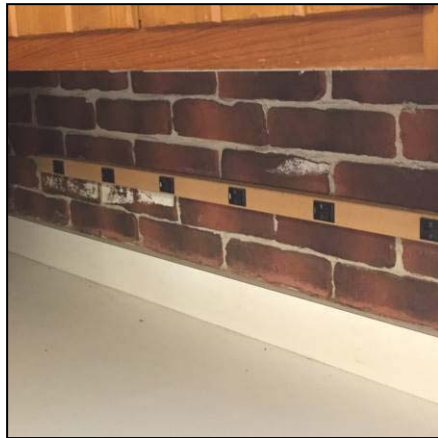
Image 20: Wiremold Strip in Kitchen
