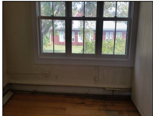
Image 7: Another Damaged Radiator, 2 nd floor bedroom
