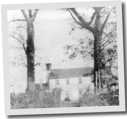
Oak Hill (north facade), ca. 1900
