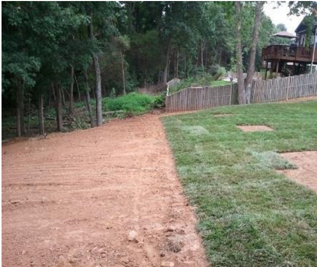
Orange Hunt Estates- Construction & clearing land in RPA
