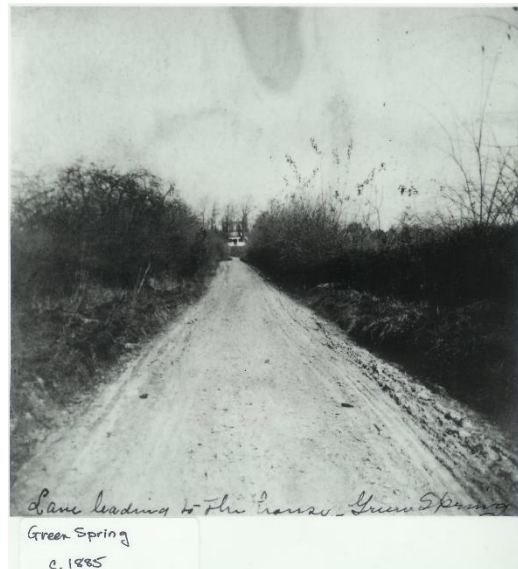
Figure 52 : Entrance Drive to Historic House, circa 1885
