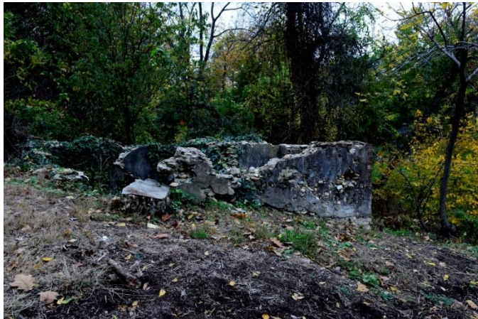
Figure 38: Foundation of Fermentation Tank
