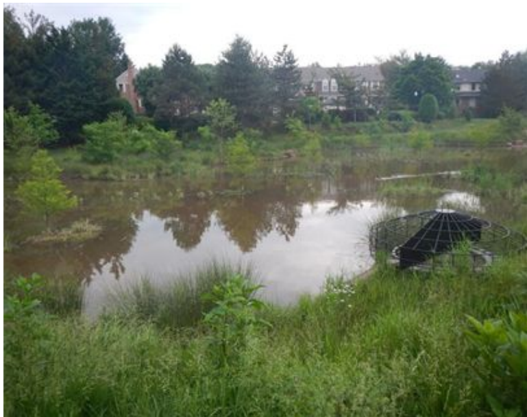
Wetland-enhanced stormwater pond retrofit
