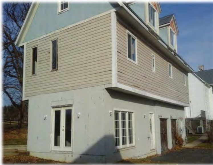
Figure 15: Turner Farm Garage with Apartment
