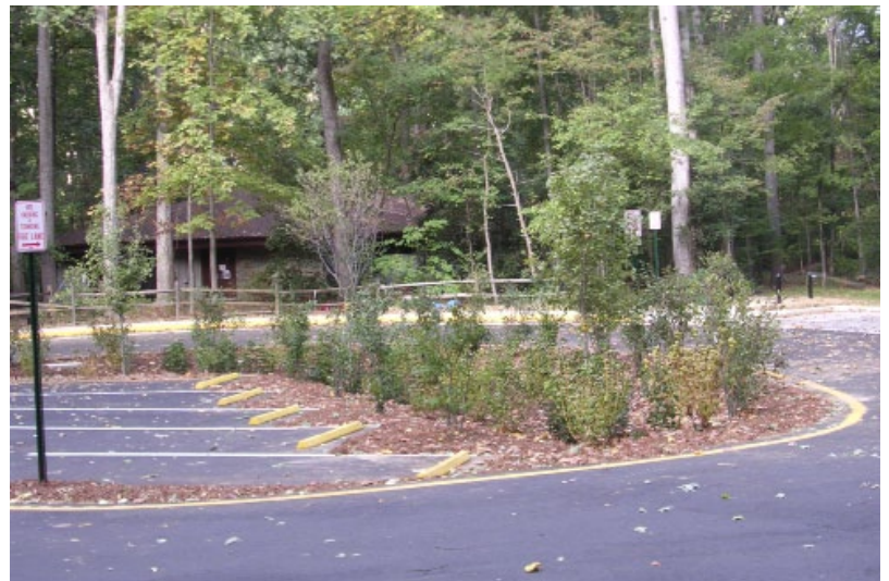
Figure 38: Rain Garden in Parking Lot Example
