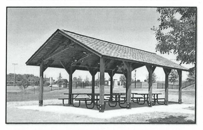
Please find the shelter and trail location in the attached Bowman Consulting site permit layout. See the RCP Shelters, Inc. rendering of the 20' x 20' custom scissor truss gable shelter with shingle roof with tables and accessible trails as recommended by the Planning & Development Division of FCPA.
