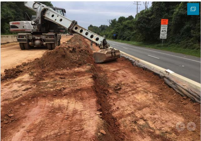
Grading material along the future Route 7 eastbound travel lanes
