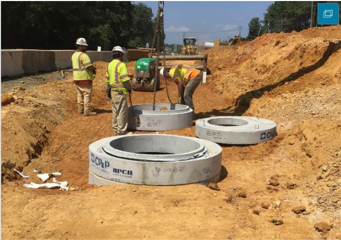
More stormwater structures
