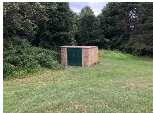
Figure 24: Irrigation Control Shed
