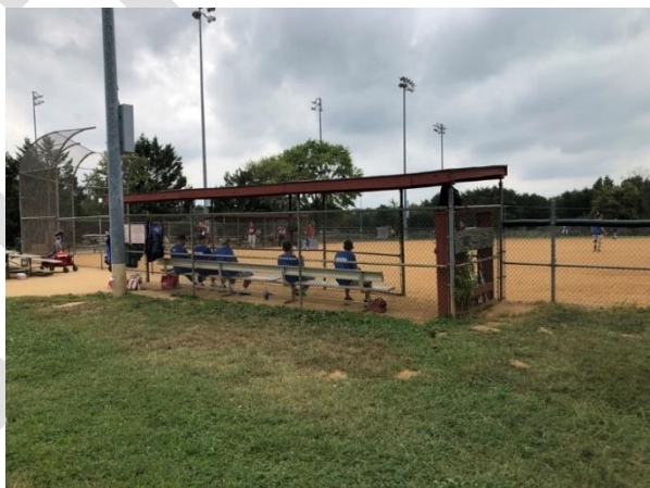
Figure 8: Braddock Park Dug Out Shelter
