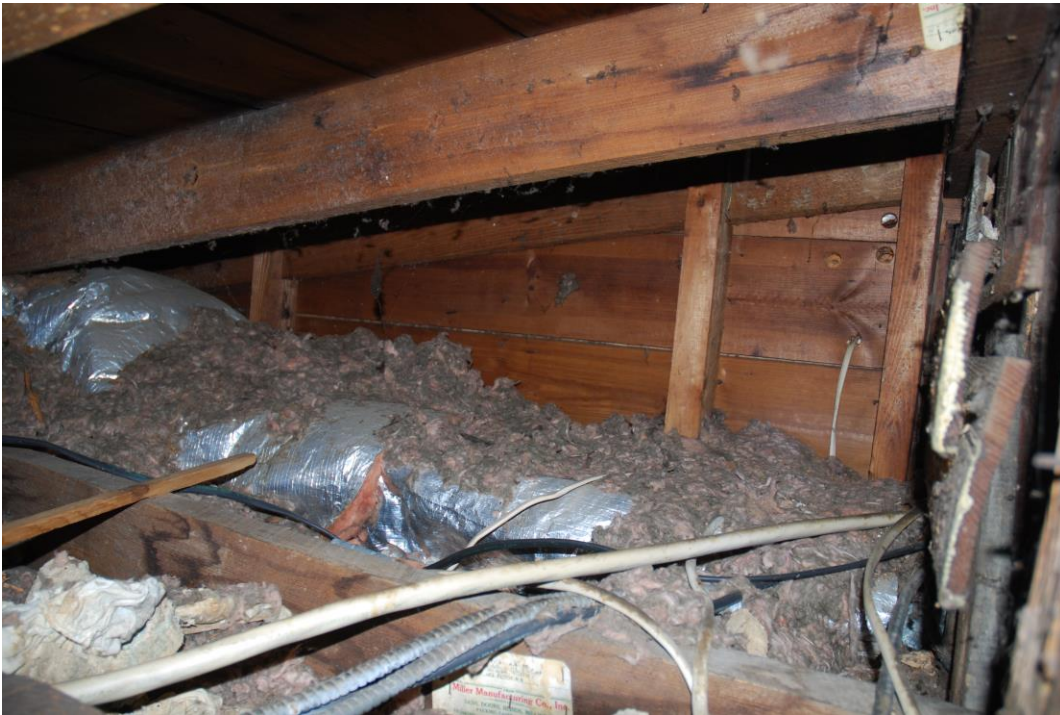
20 Room 209 Kitchen Attic
