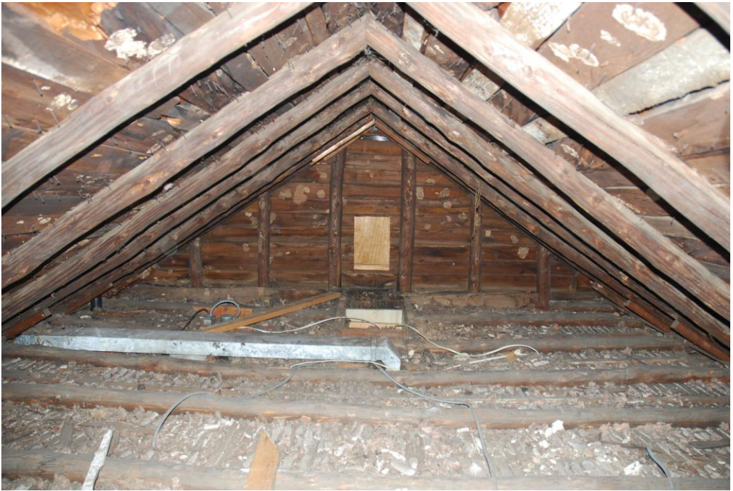
22 Room 301 East Attic
