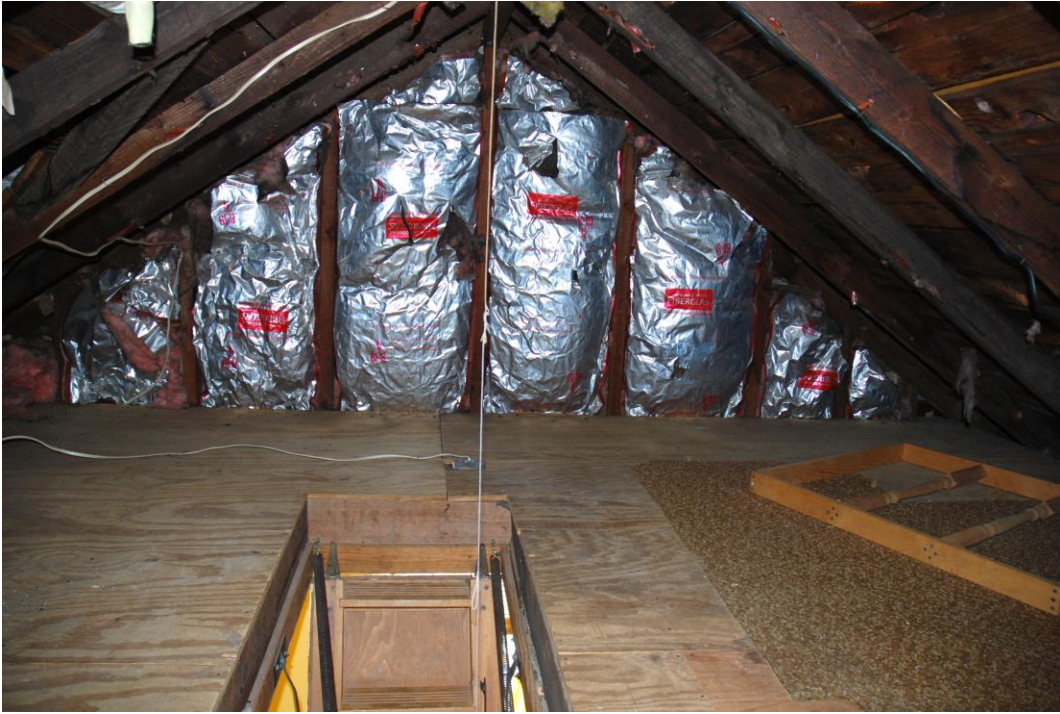
21 Room 300 West Attic
