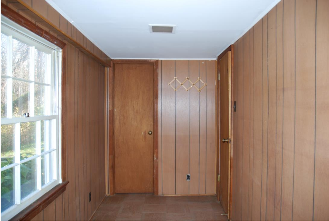
13 Room 103 Front/Enclosed Porch
