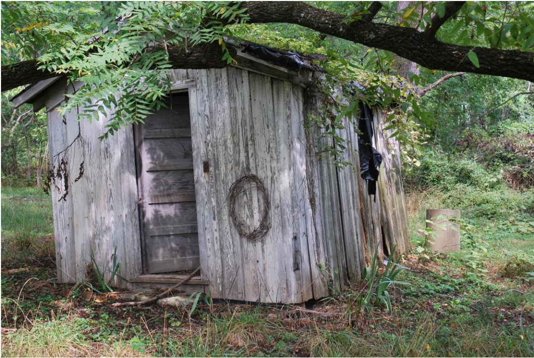
8 Railroad tool shed
