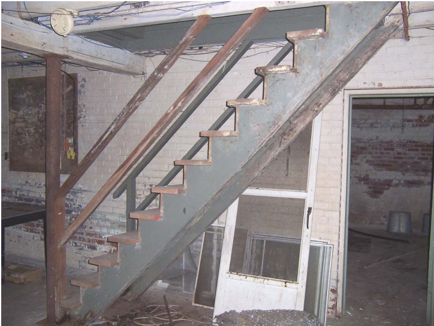
Existing Condition Photo B18: Stempson House Basement Basement Stairs
