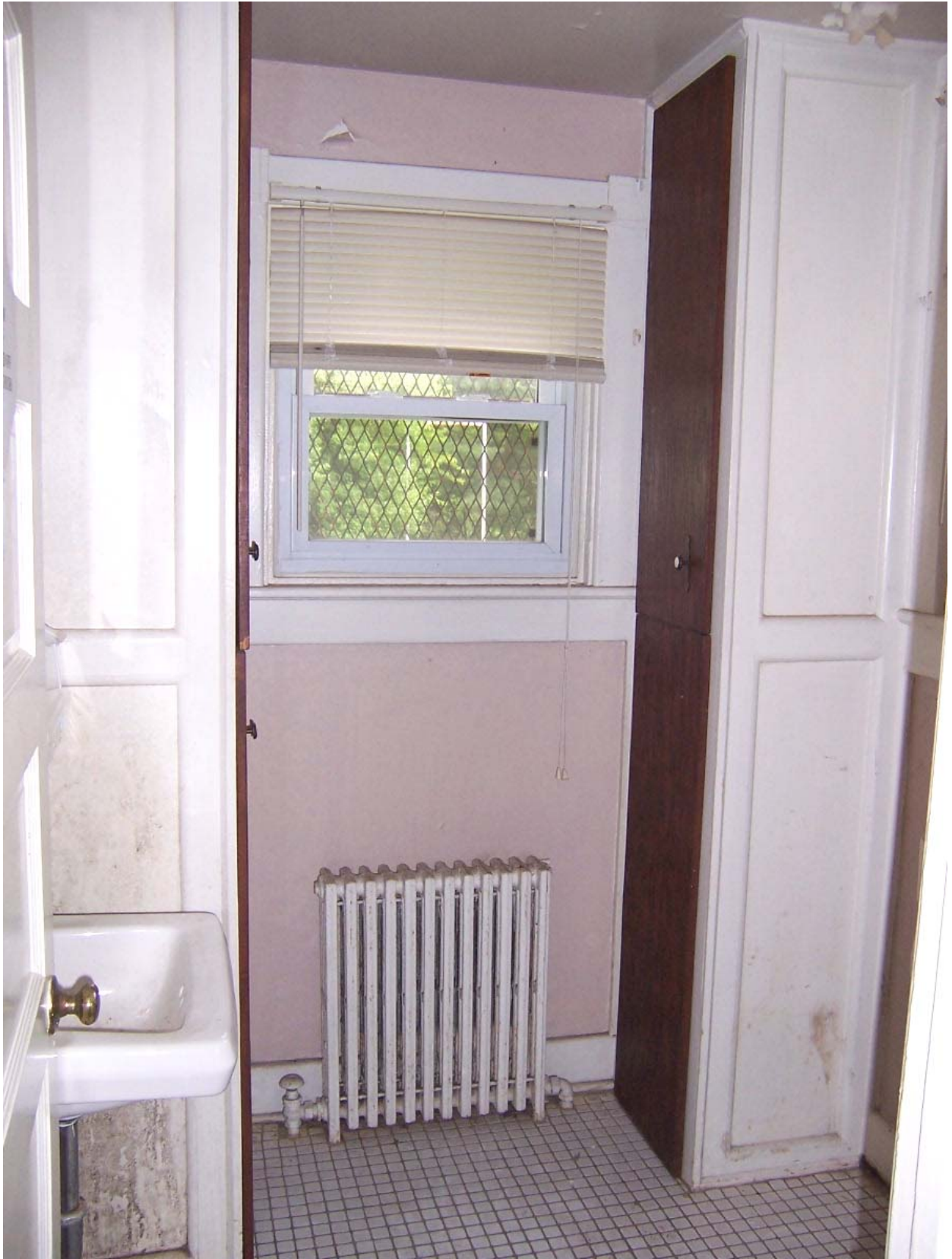
Existing Condition Photo B49: Stempson House First Floor Toilet Room (Room 105)
