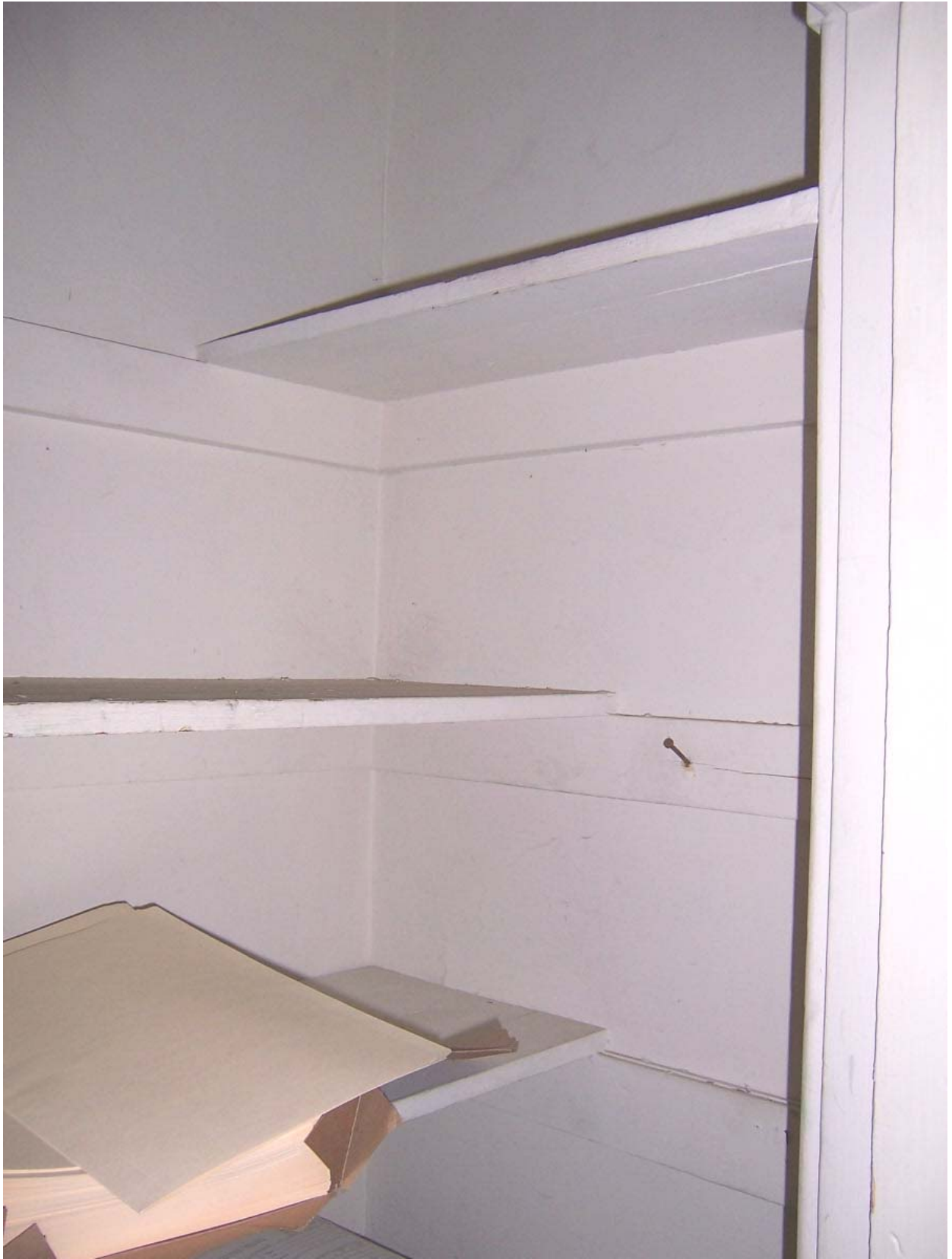
Existing Condition Photo B78: Stempson House Second Floor Closet (Room 209)
