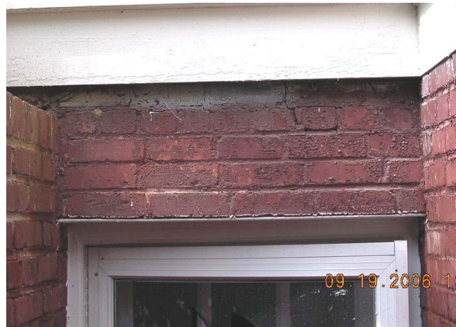
Image 3.97: Brick Infill Above Door (D01)
