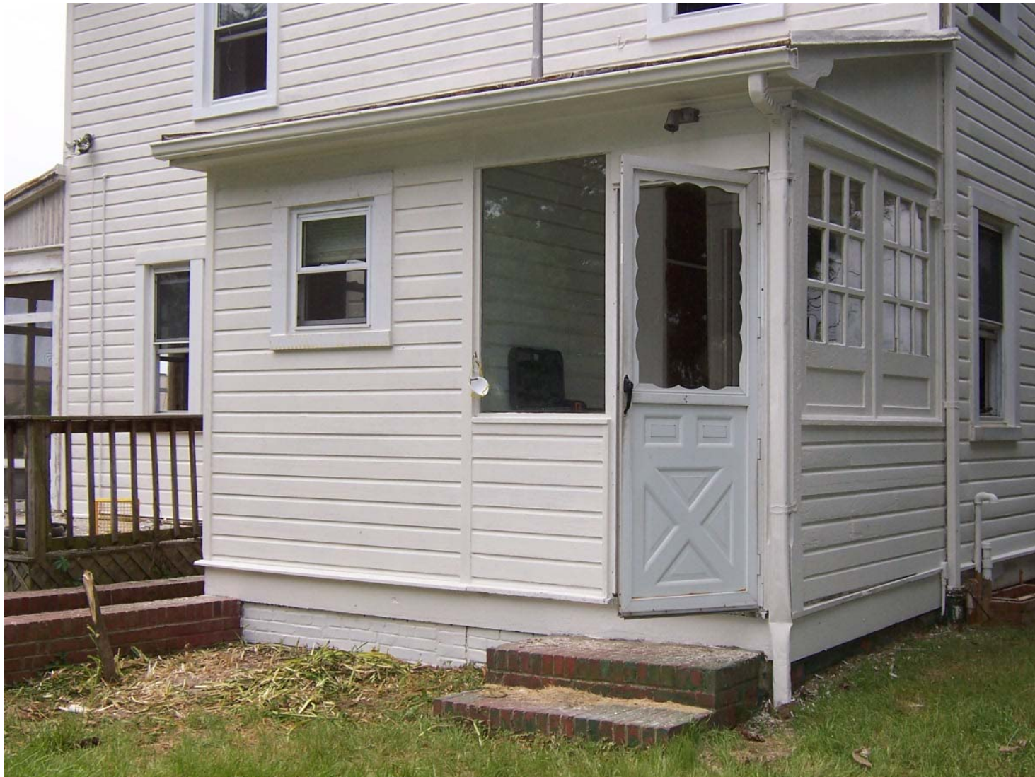
Existing Condition Photo B11: Stempson House Exterior Enclosed East Porch
