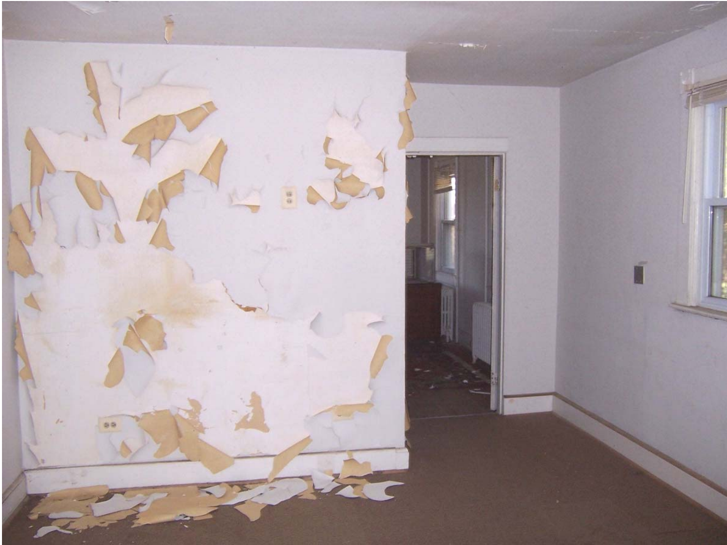
Existing Condition Photo B38: Stempson House First Floor Kitchen (Room 102)
