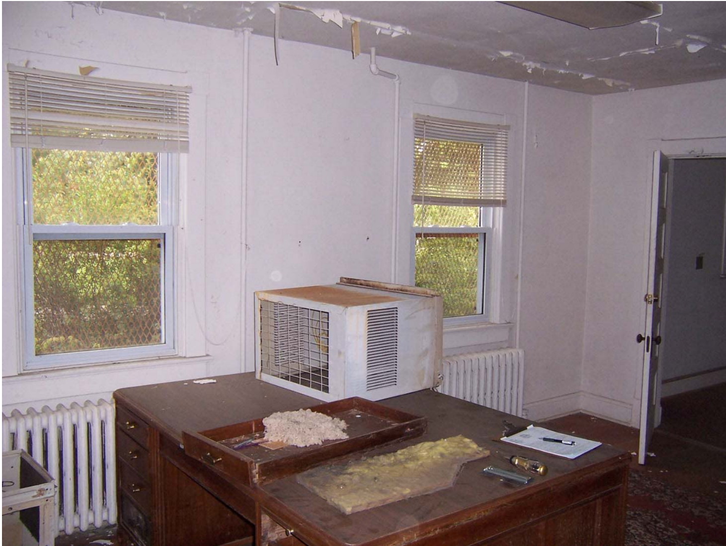
Existing Condition Photo B35: Stempson House First Floor Room 101
