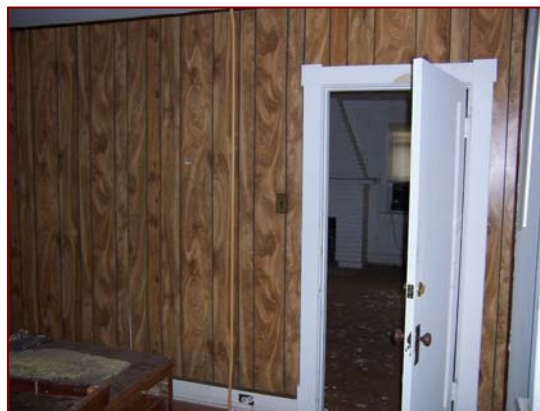
Image 3.54: Fiberboard Paneling in Room 101
