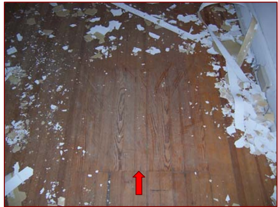
Image 3.61: Wood Flooring Infills Penetration
