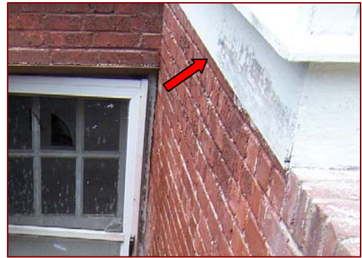
Image 3.100: Sloped Porch Floor
