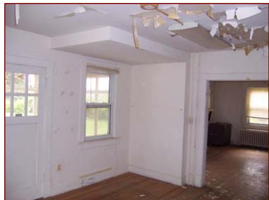
Image 3.110: Bulkhead and Plumbing Chase
