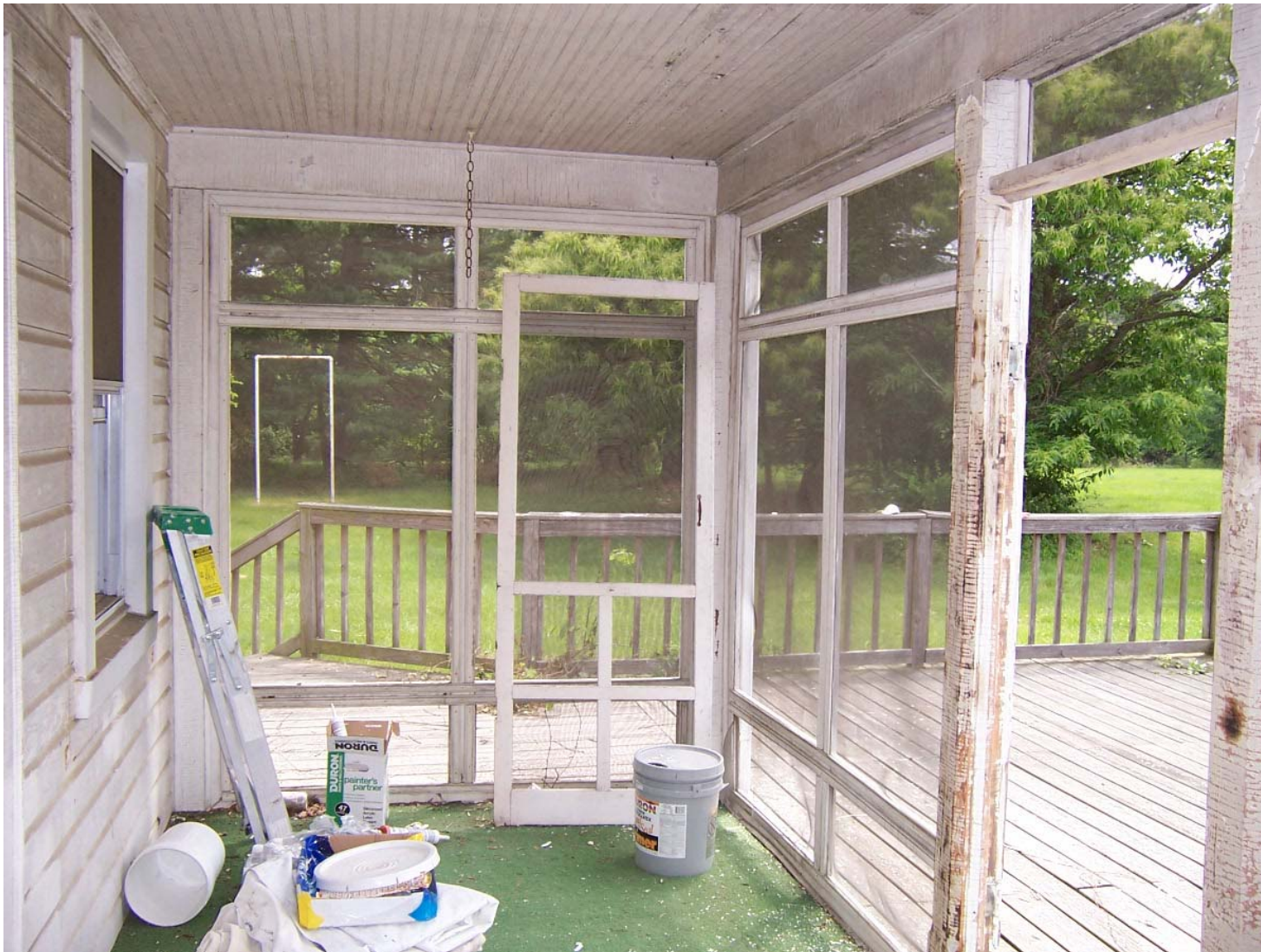
Existing Condition Photo B52: Stempson House First Floor Screened Porch (Room 106)
