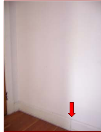
Image 3.108: Arrow Locates Start of Baseboard Infill in Hall
