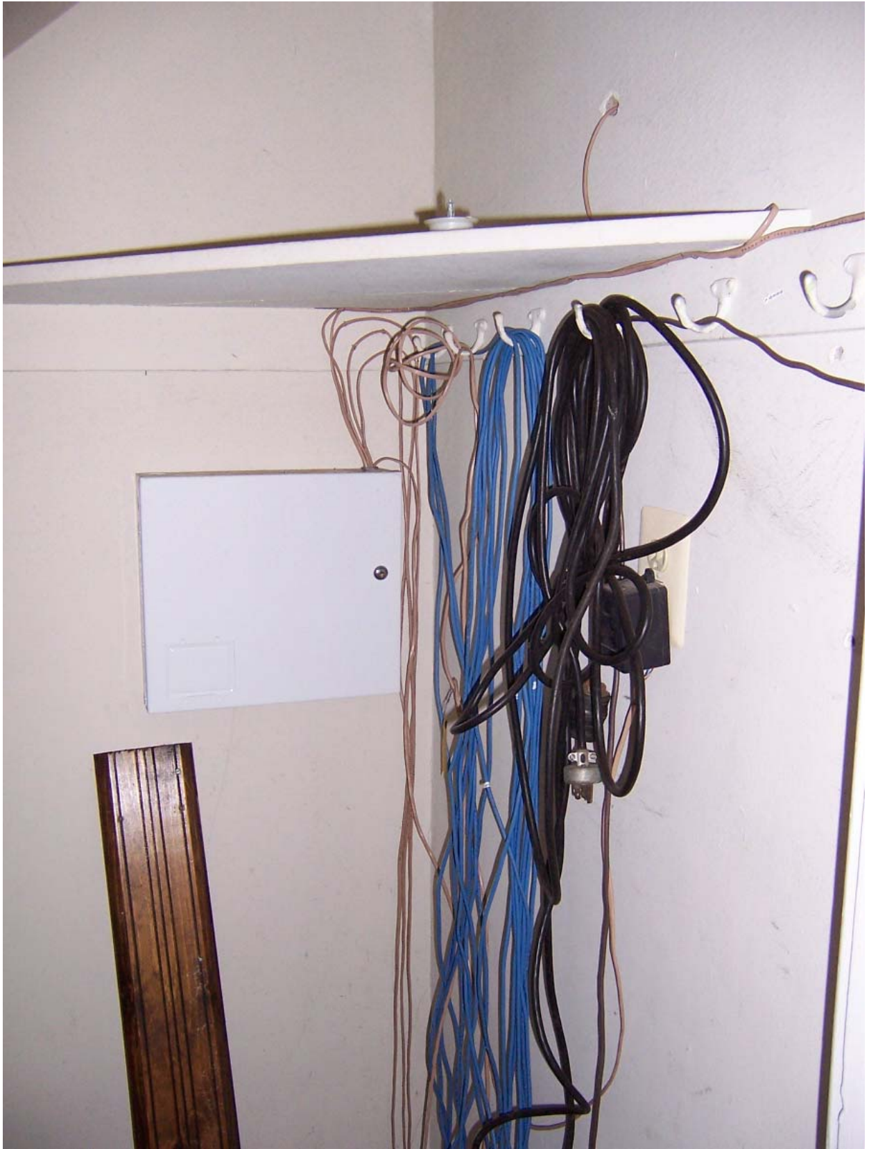
Existing Condition Photo B54: Stempson House First Floor Closet (Room 107)
