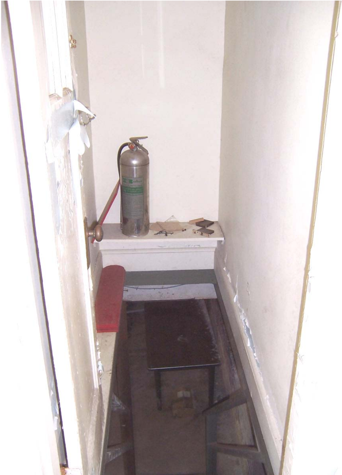
Existing Condition Photo B41: Stempson House Basement Basement Stairs From Room 102
