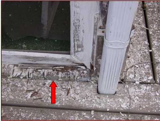
Image 3.91: Screened Porch Flooring
