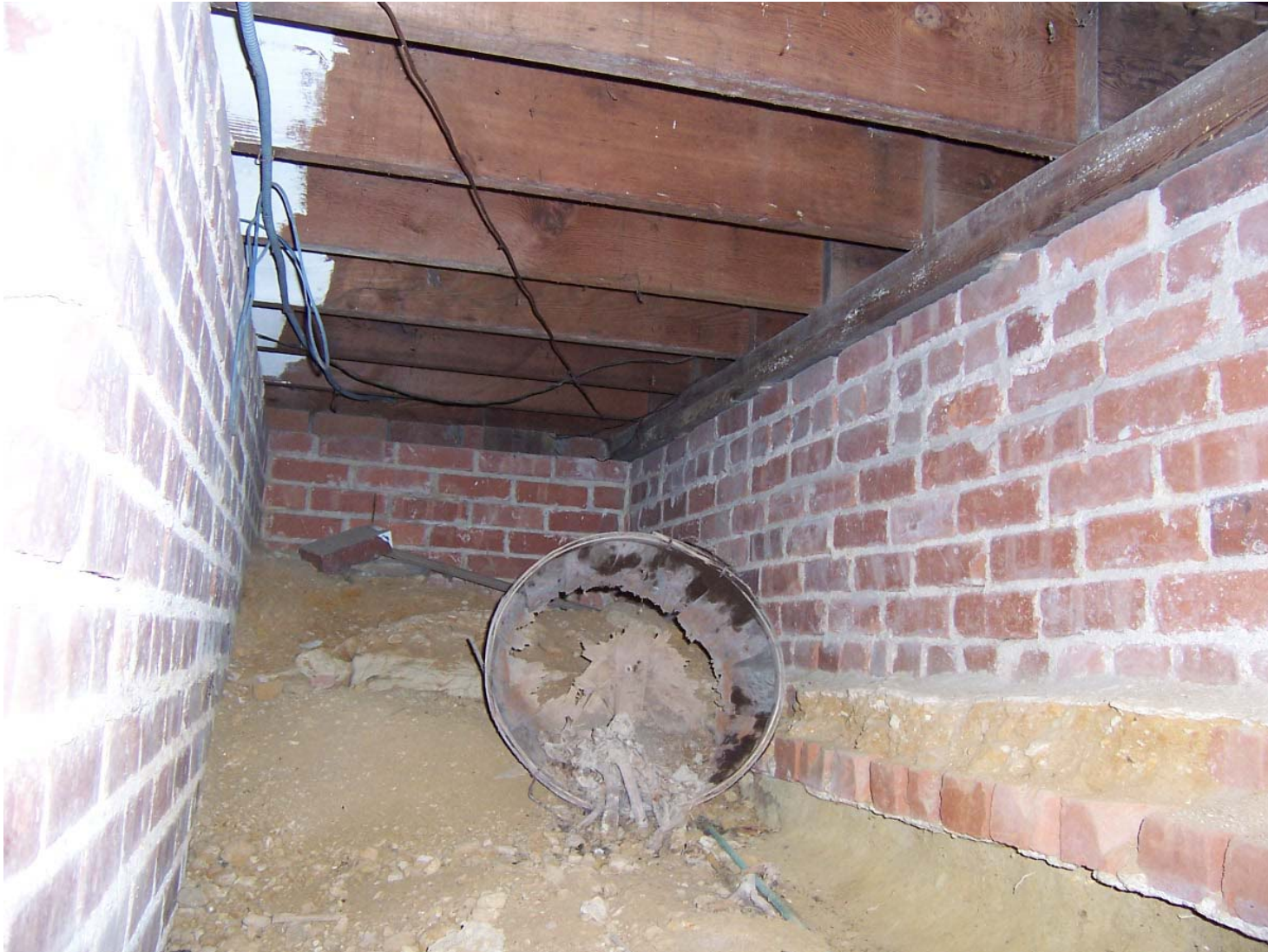
Existing Condition Photo B16: Stempson House Basement Basement Space B2
