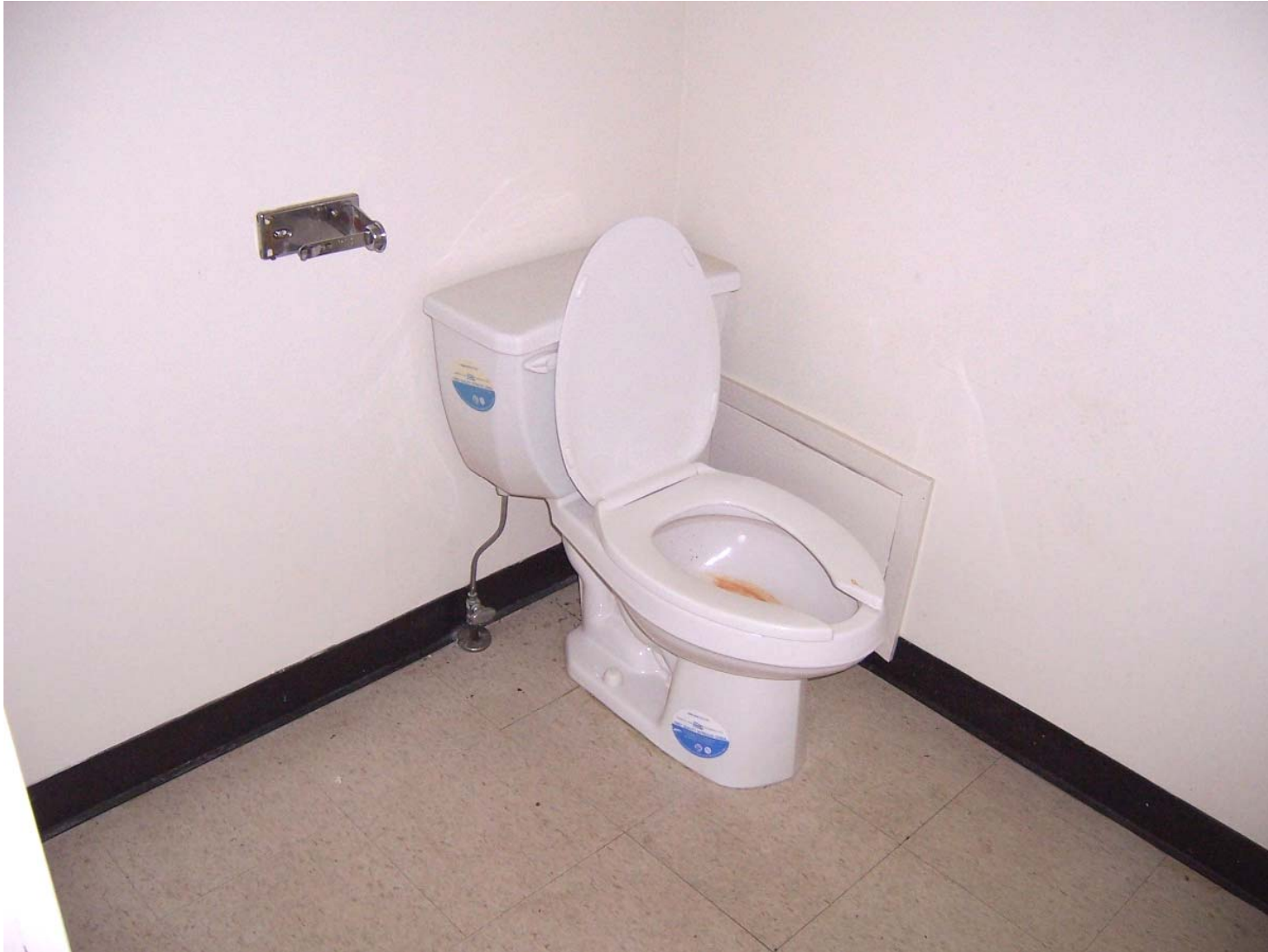
Existing Condition Photo B73: Stempson House Second Floor Toilet Room (Room 206)
