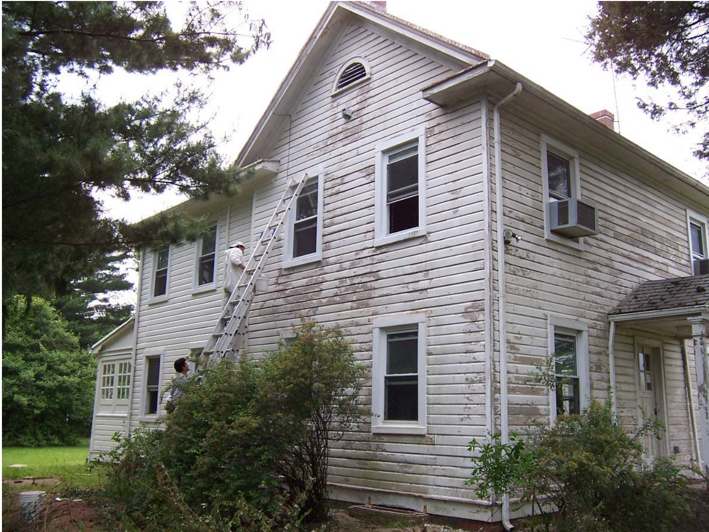
Existing Condition Photo B4: Stempson House Exterior Northwest Elevation
