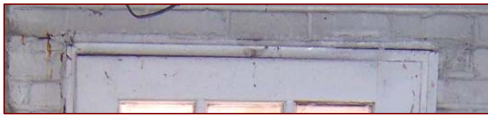
Image 3.95: Lintel Above Exterior Basement Door
