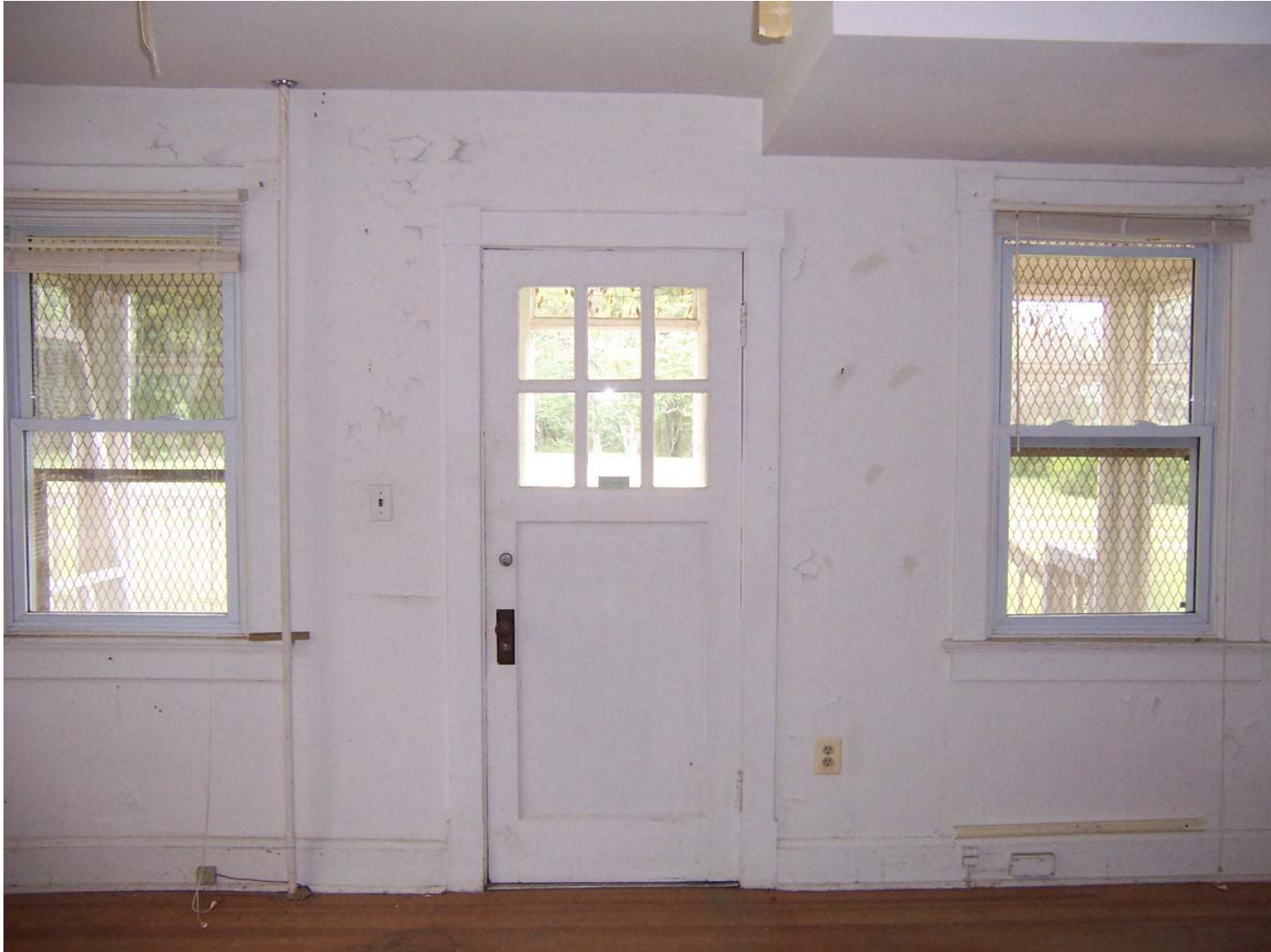
Existing Condition Photo B44: Stempson House First Floor Room 103
