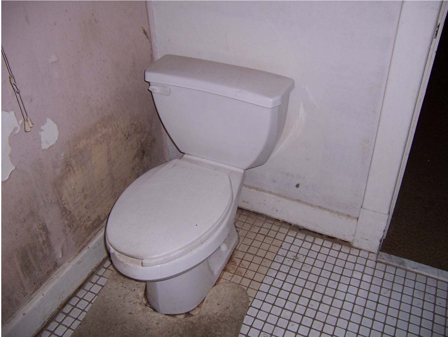
Existing Condition Photo B50: Stempson House First Floor Toilet (Toilet Room 105)
