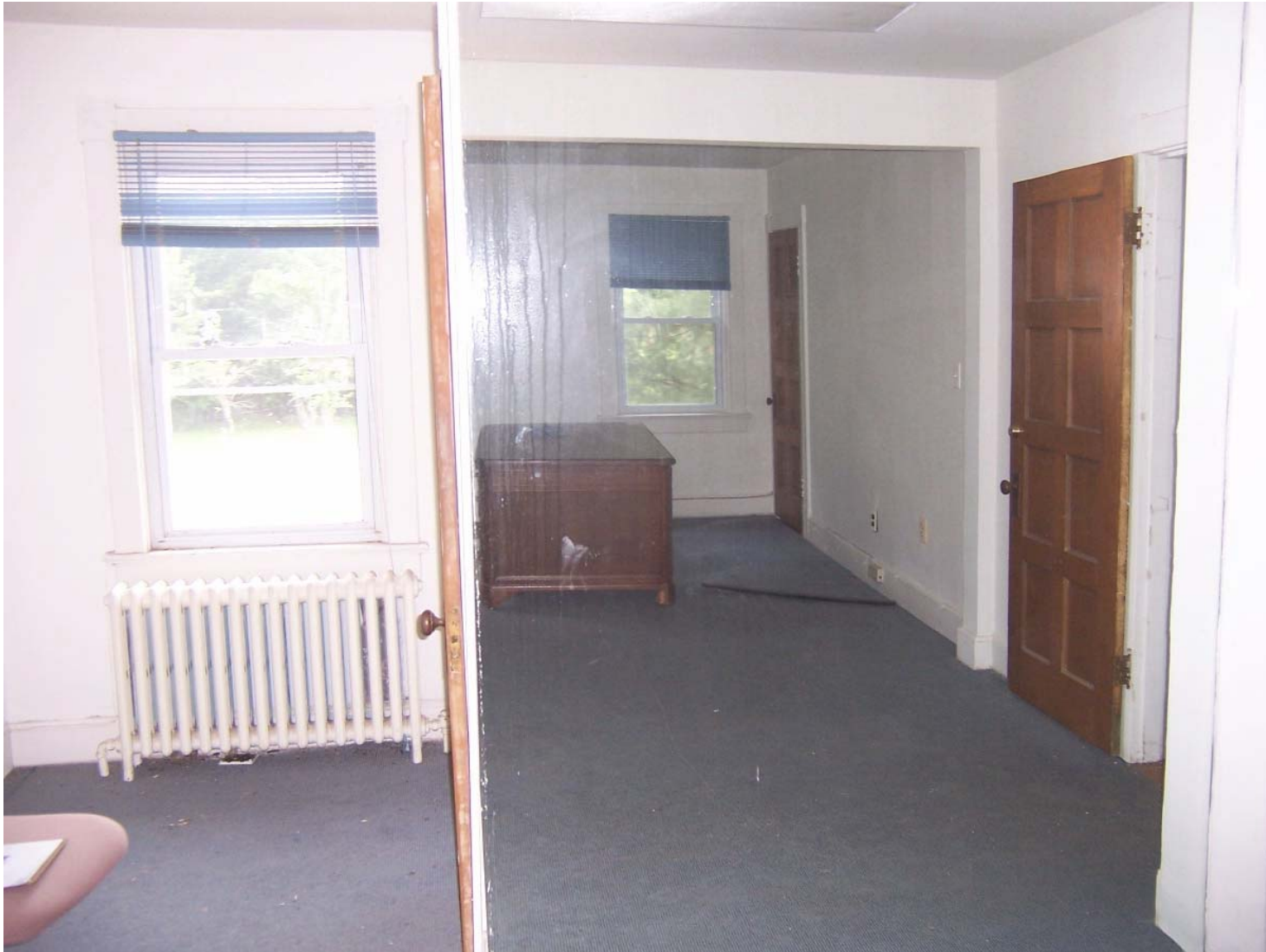
Existing Condition Photo B64: Stempson House Second Floor Bedroom/Office (Room 203)
