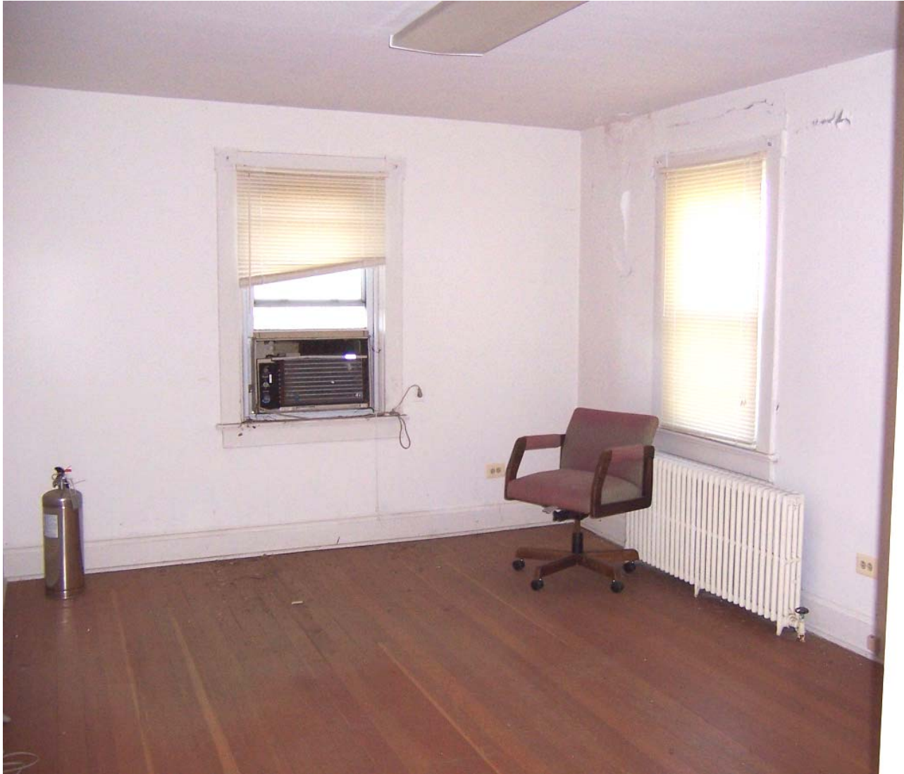
Existing Condition Photo B59: Stempson House Second Floor Bedroom (Room 201)
