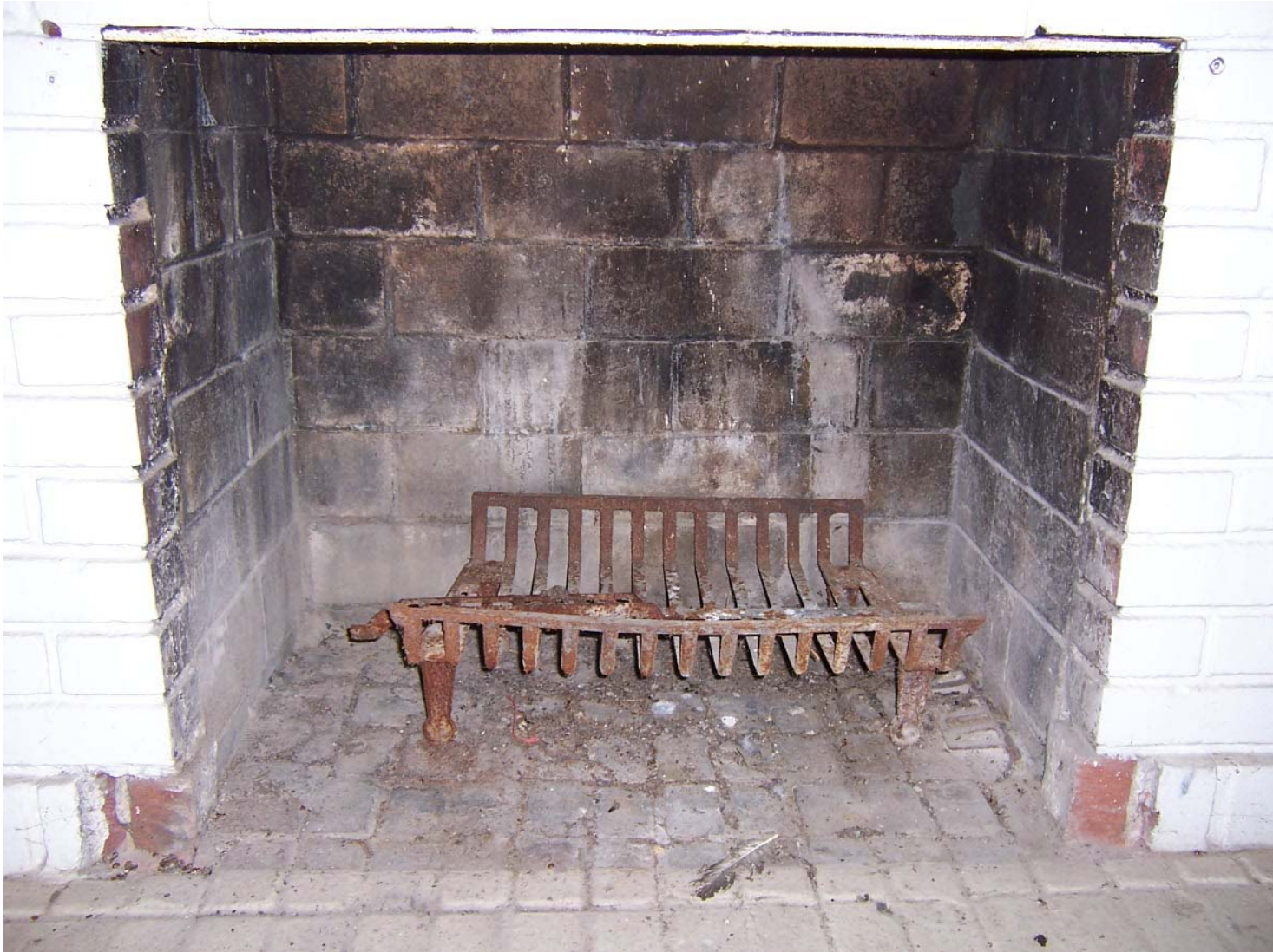
Existing Condition Photo B32: Stempson House First Floor Firebox
