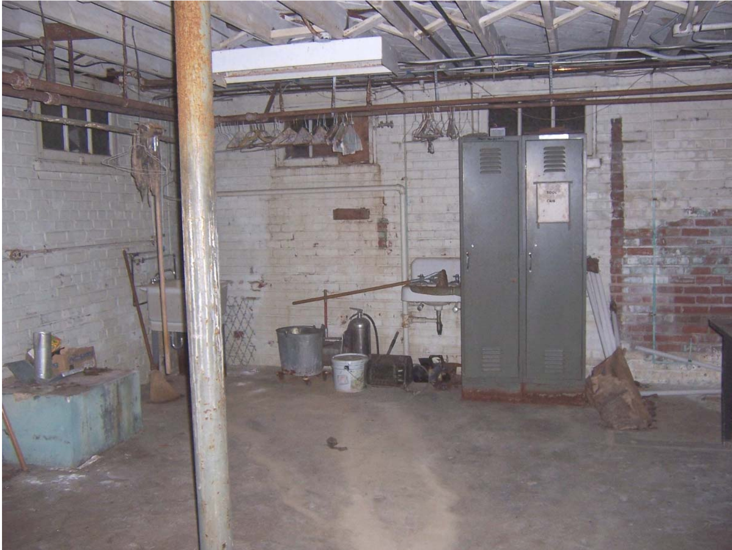
Existing Condition Photo B20: Stempson House Basement Basement Room B4
