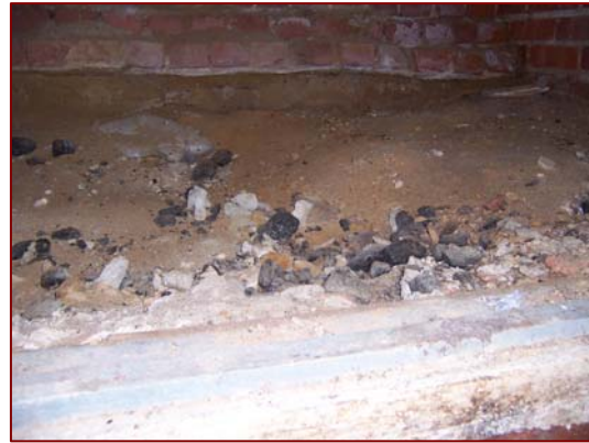
Image 3.11: Extant Coal in Space B2
