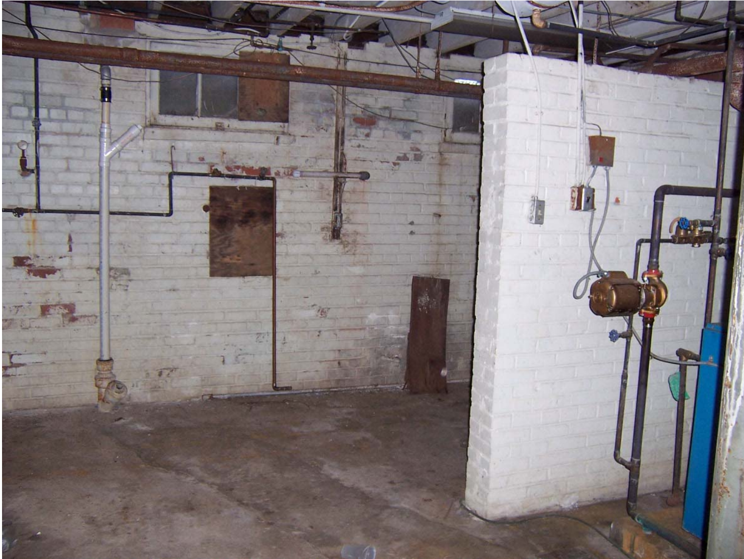
Existing Condition Photo B21: Stempson House Basement Basement Room B4
