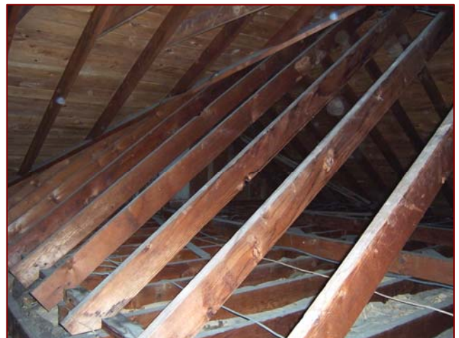
Image 3.28: Rafter and False Plate at Eave
