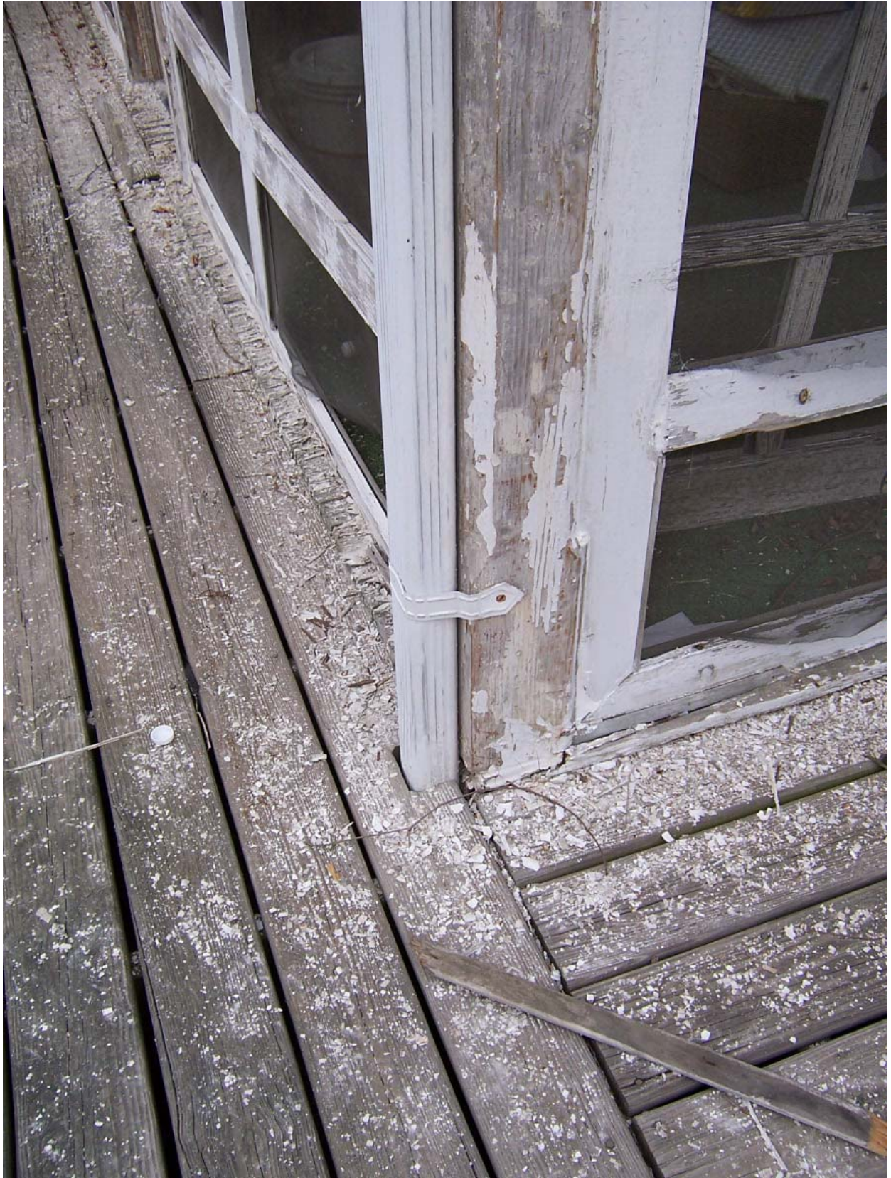
Existing Condition Photo B09: Stempson House Exterior Chamfered Screened-Porch Column
