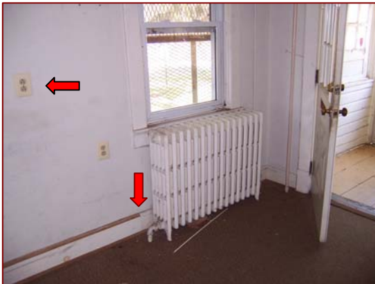
Image 3.86: Arrows Locate Transition Between Old and New Baseboard and Counter-Height Outlet
