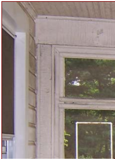
Image 3.102: Screen Wall Framing Butts Siding
