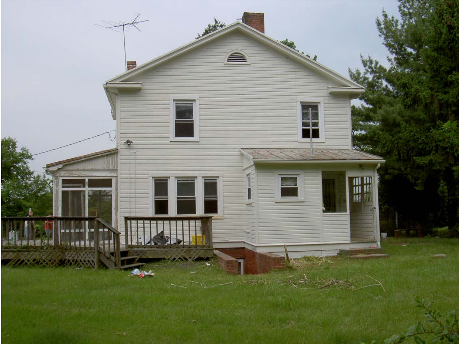
Existing Condition Photo B3: Stempson House Exterior East Elevation
