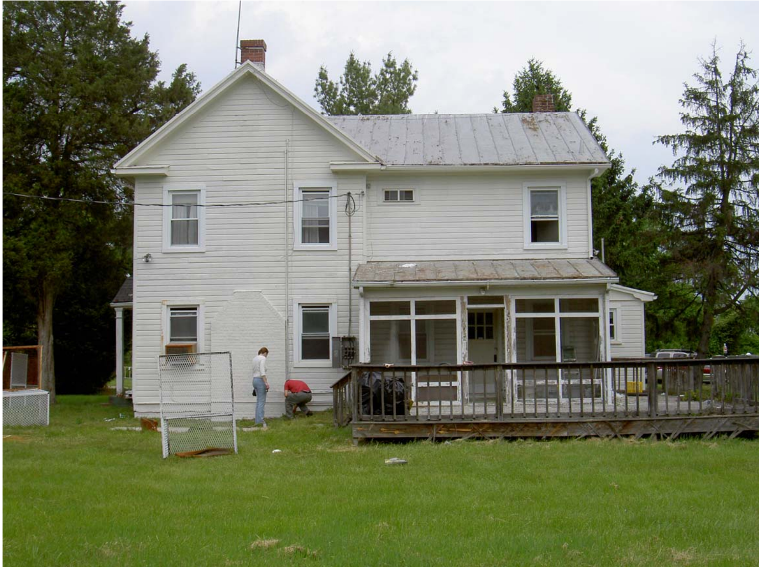
Existing Condition Photo B2: Stempson House Exterior South Elevation
