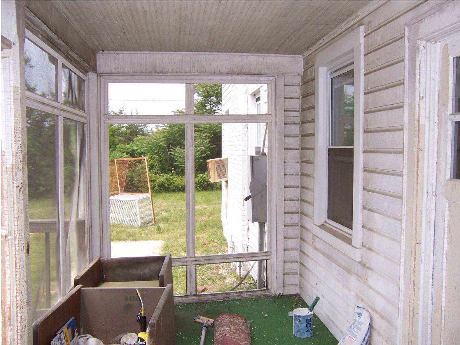
Existing Condition Photo B53: Stempson House First Floor Screened Porch (Room 106)
