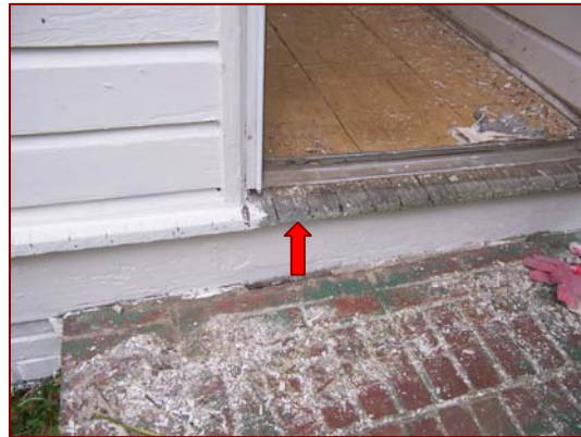
Image 3.92: Rear Porch Flooring
