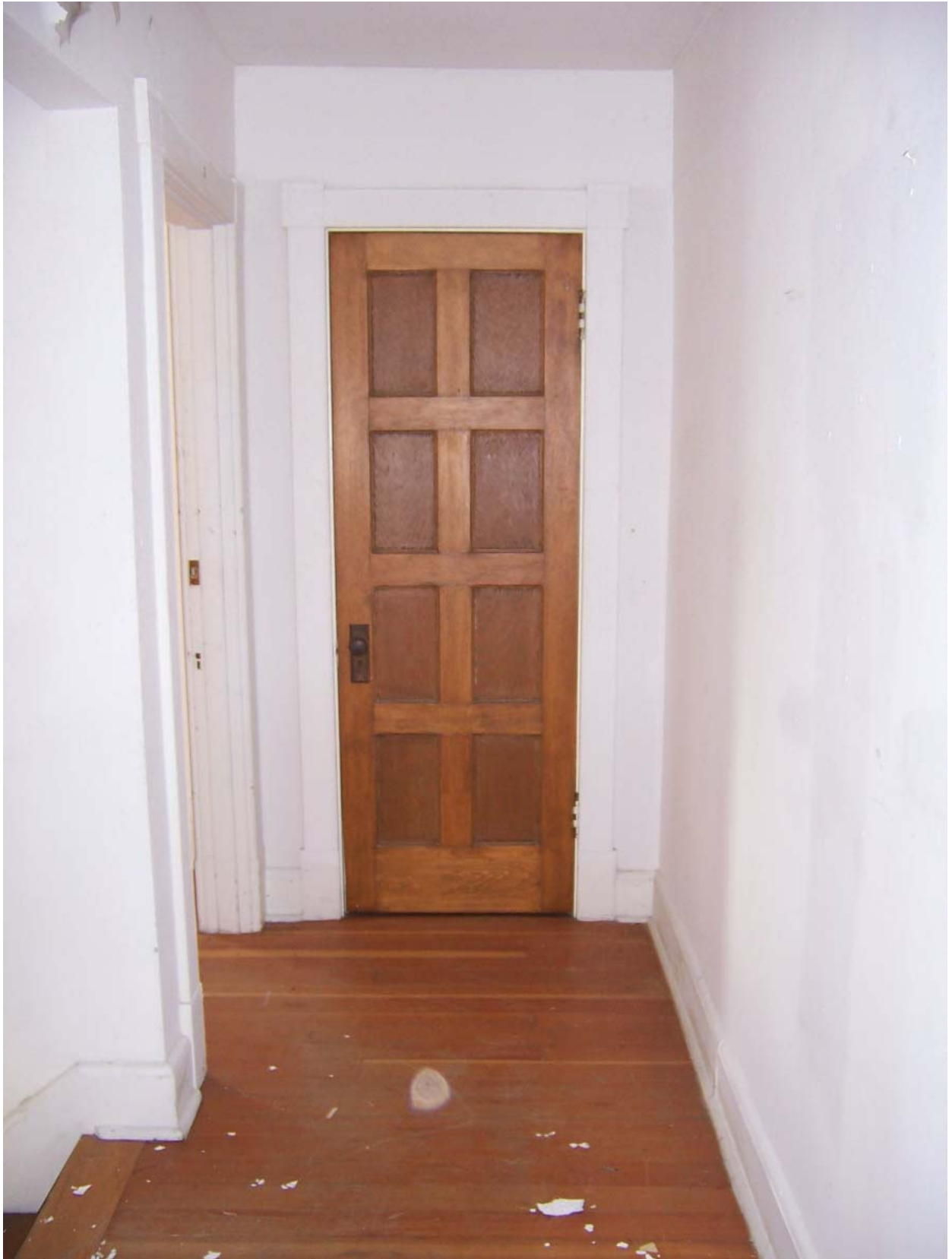
Existing Condition Photo B69: Stempson House Second Floor Hall (Room 204)
