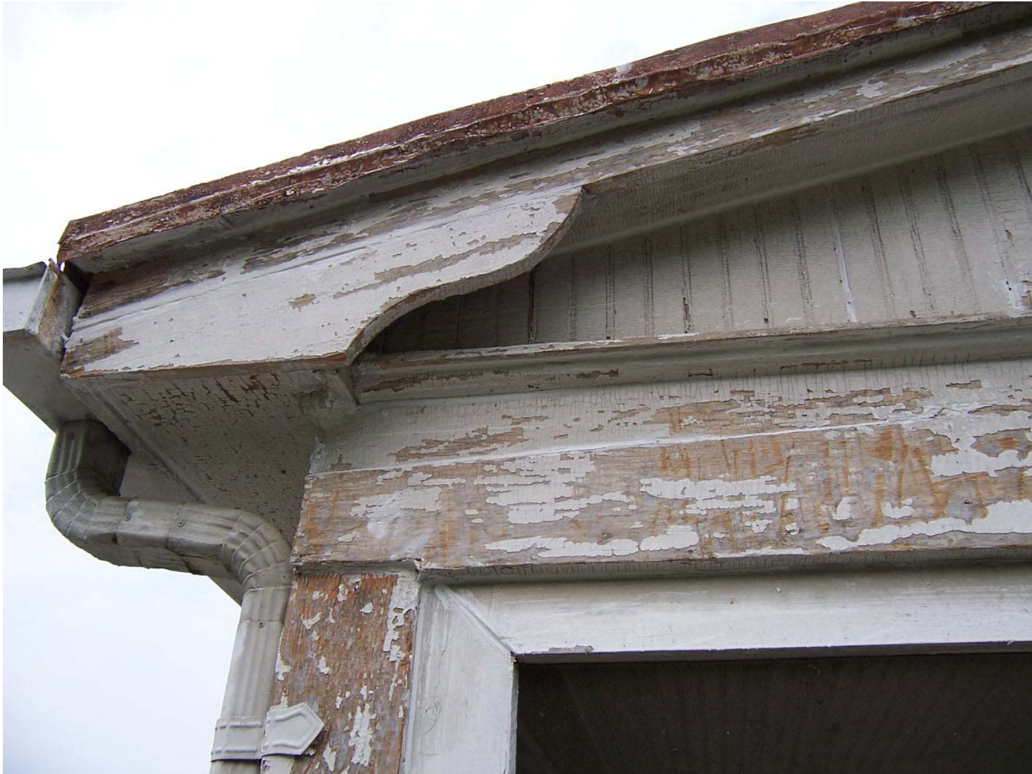
Existing Condition Photo B12: Stempson House Exterior Enclosed East Porch Detail
