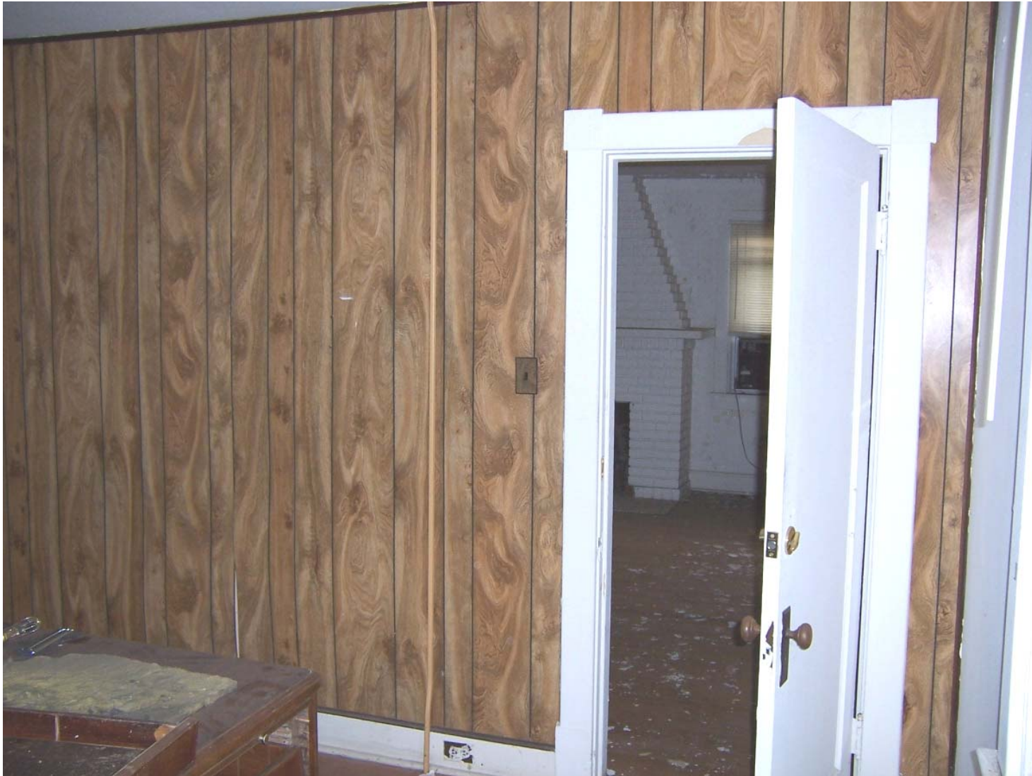
Existing Condition Photo B34: Stempson House First Floor Room 101
