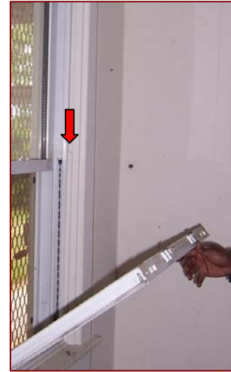
Image 3.106: Frame at Lower Sash
