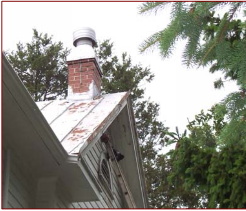
Image 3.23: Northern Chimney with Ventilator
