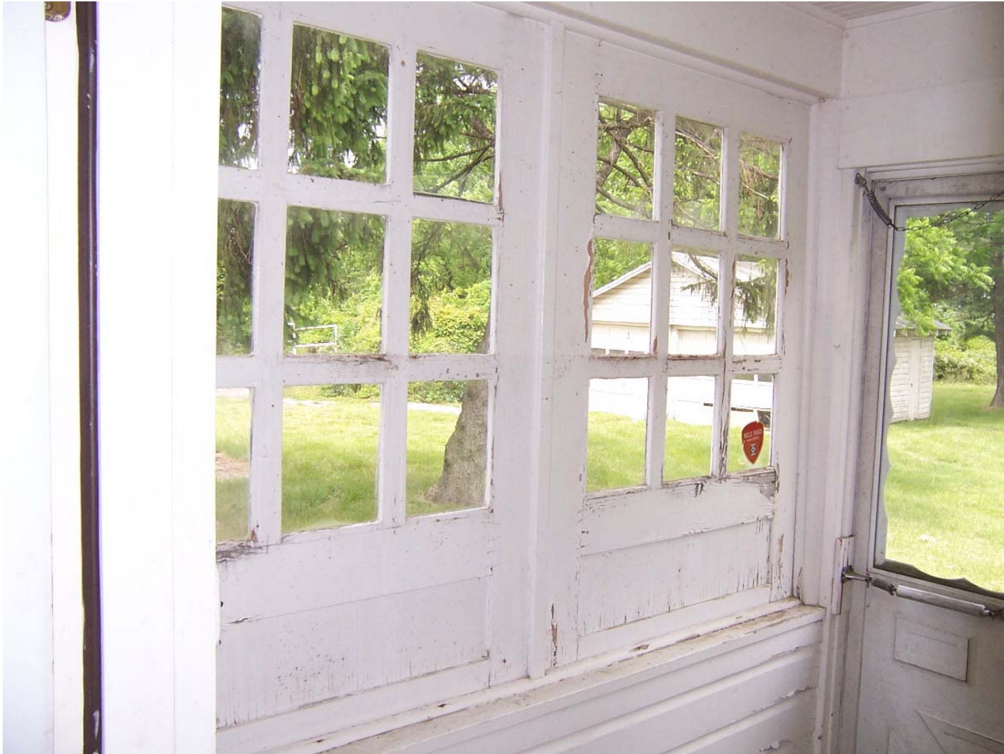
Existing Condition Photo B46: Stempson House First Floor Vestibule (Room 104)
