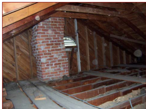
Image 3.78: Eastern Chimney in Attic
