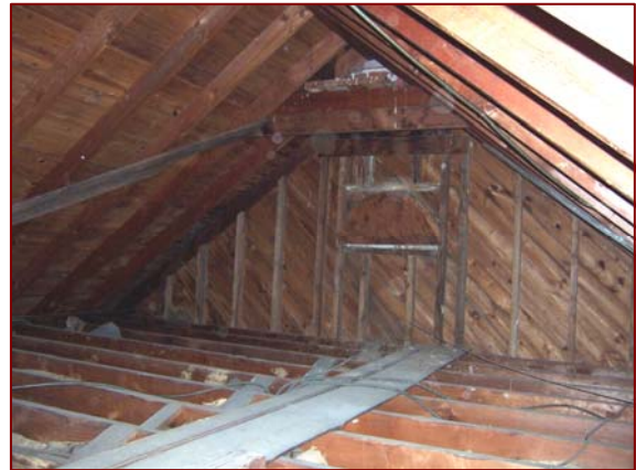
Image 3.27: Framing in Attic Space
