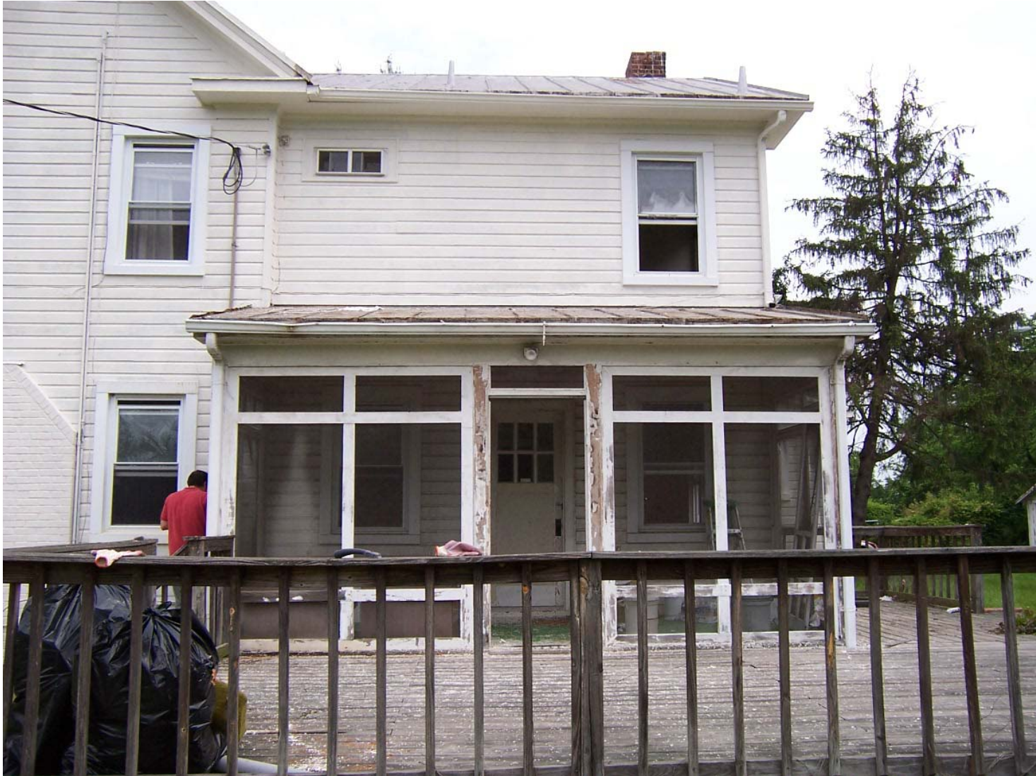
Existing Condition Photo B8: Stempson House Exterior Screened Porch
