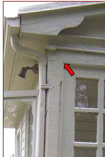
Image 3.94: Rear Porch Column Detail
