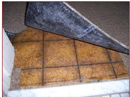
Image 3.87: Kitchen-style Vinyl Flooring
