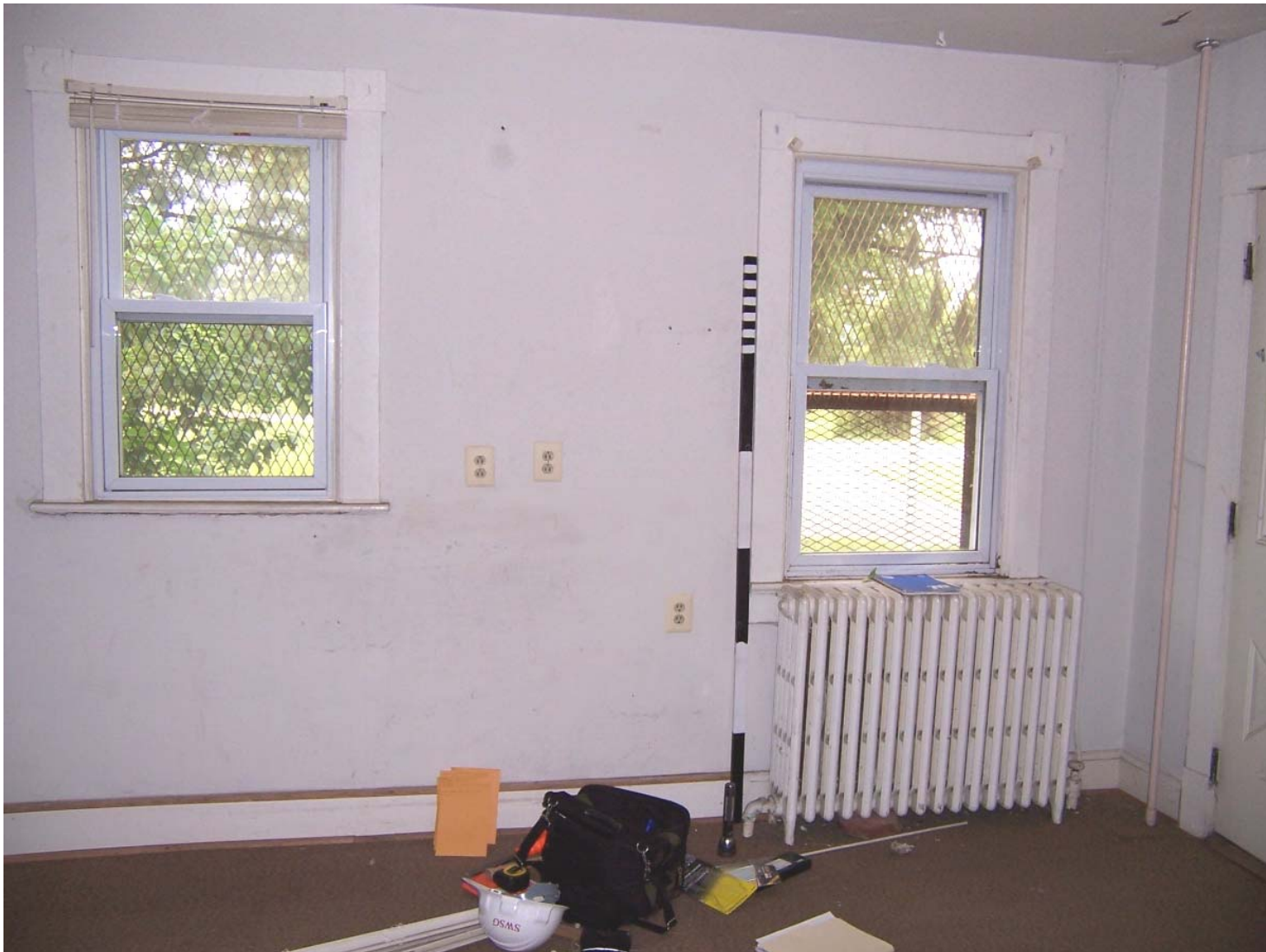
Existing Condition Photo B39: Stempson House First Floor Kitchen (Room 102)
