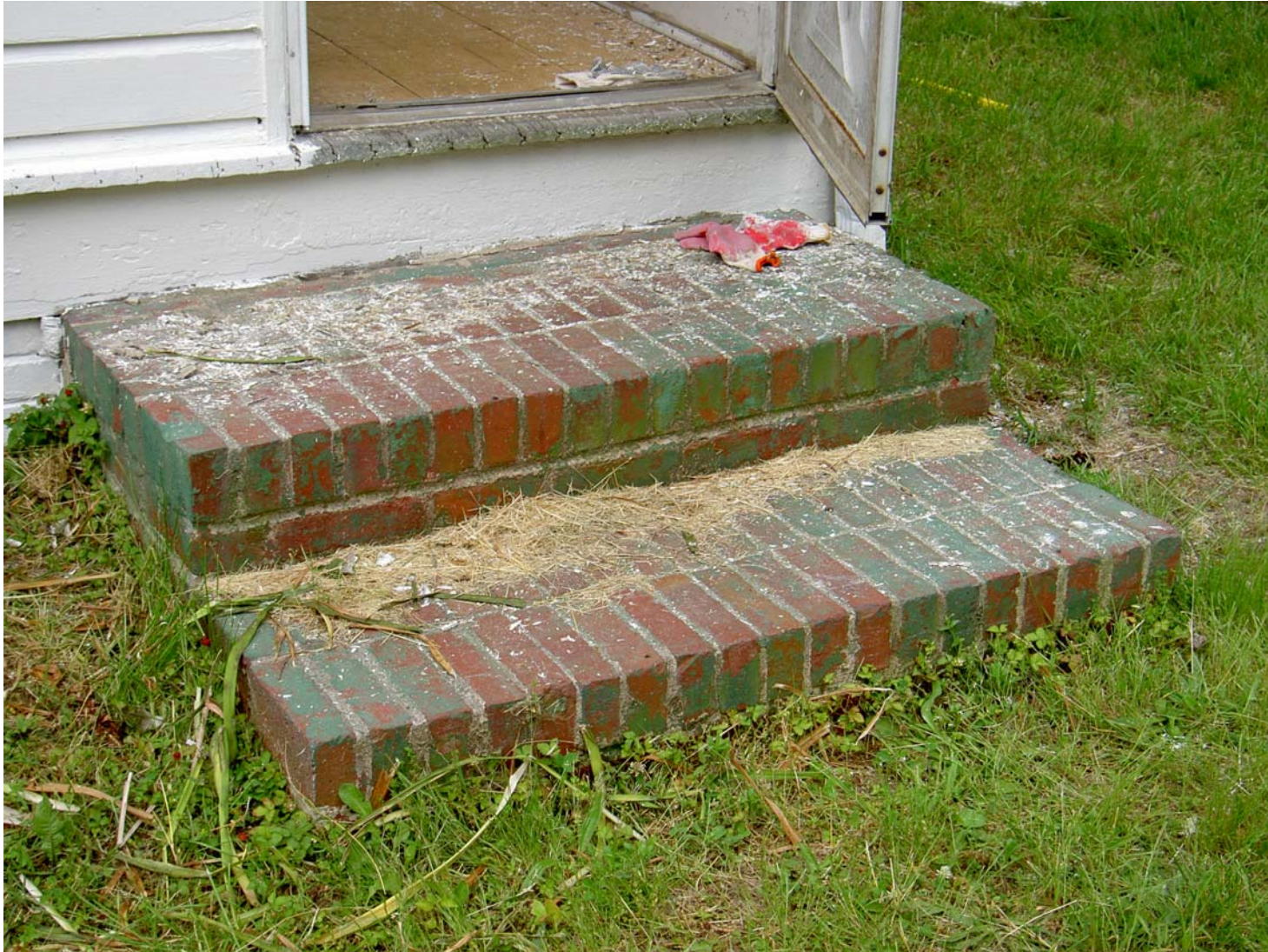
Existing Condition Photo B13: Stempson House Exterior East Porch Steps
