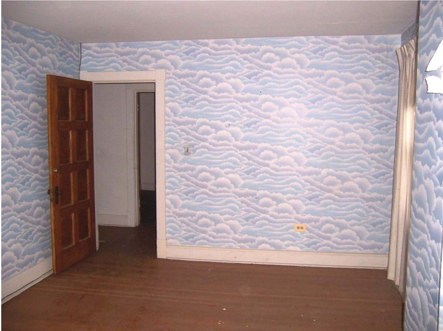
Existing Condition Photo B57: Stempson House Second Floor Bedroom (Room 200)
