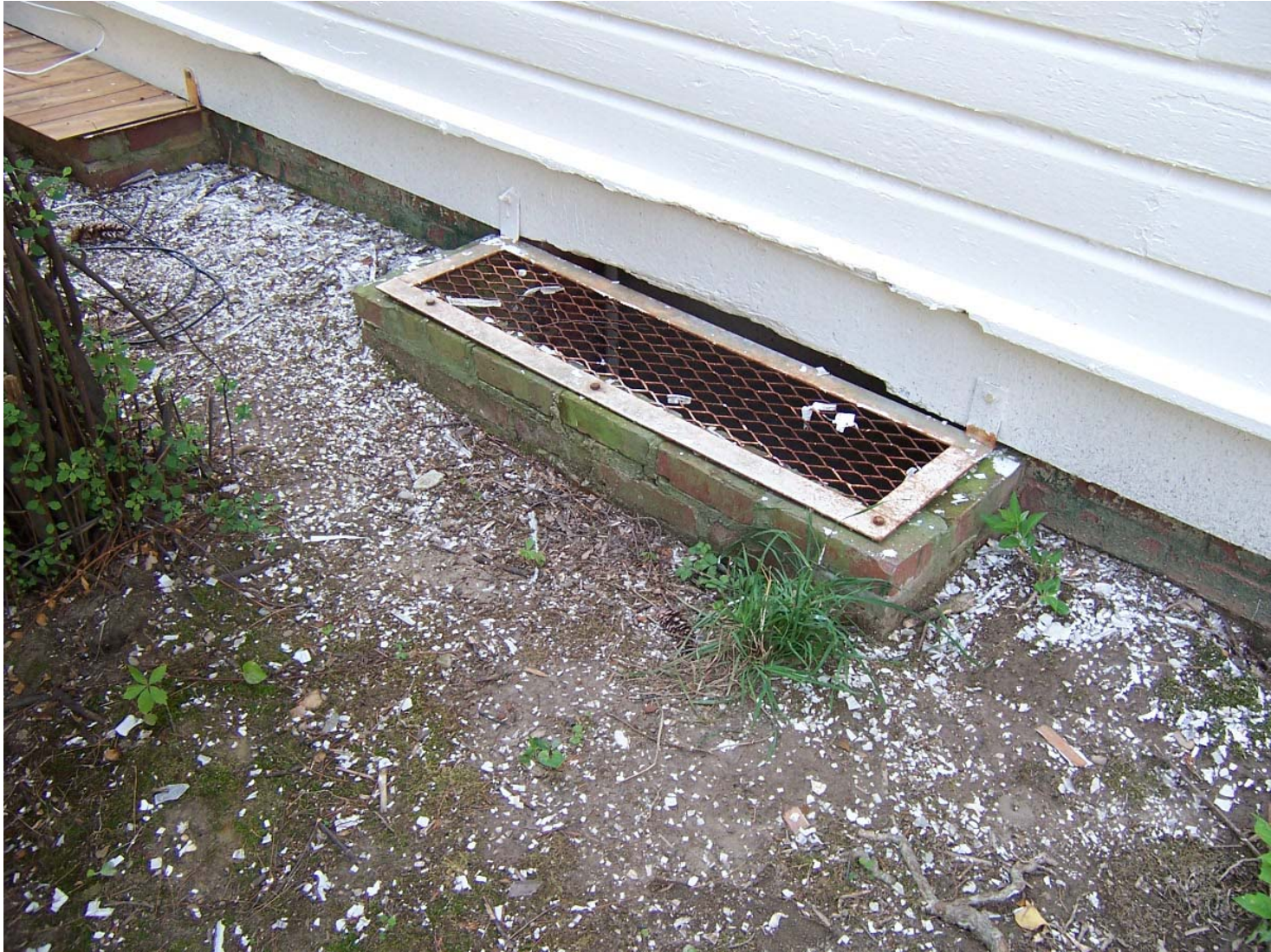
Existing Condition Photo B14: Stempson House Exterior Typical Basement Areaway
