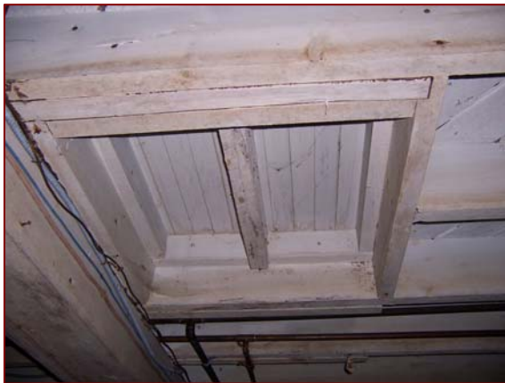
Image 3.60: Framed Out Penetration
