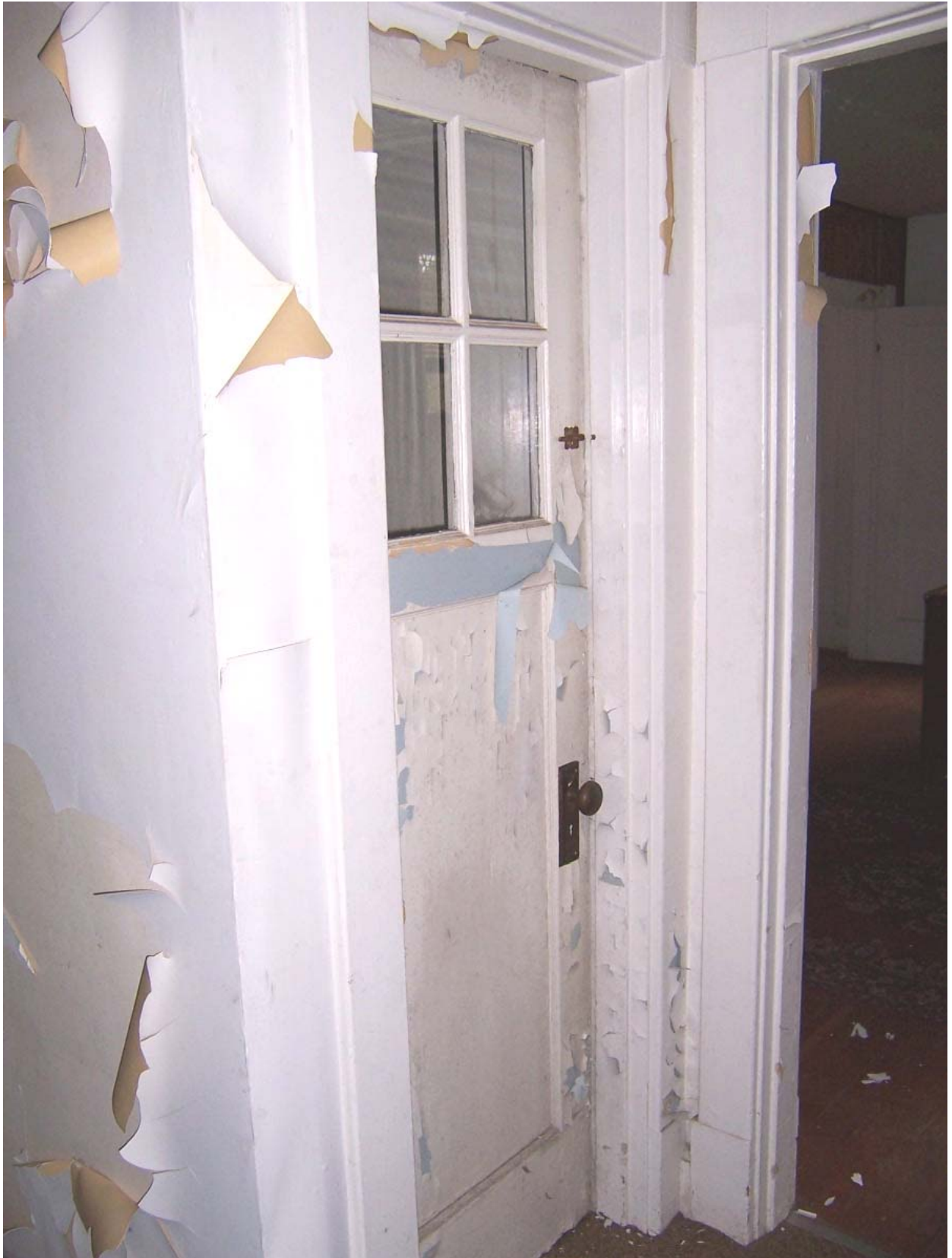
Existing Condition Photo B40: Stempson House Basement Interior Door (D105)
