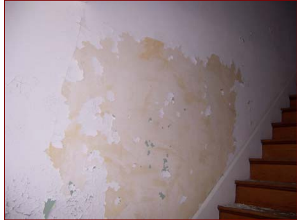
Image 3.44: Plaster Wall Covered With Painted Brown Paper
