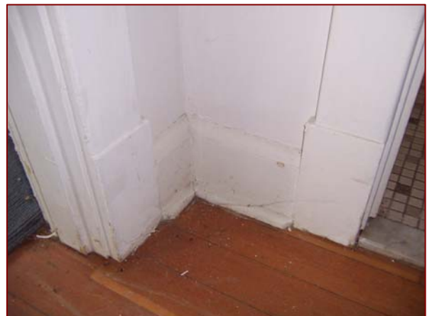
Image 3.90: Baseboard at Bathroom
