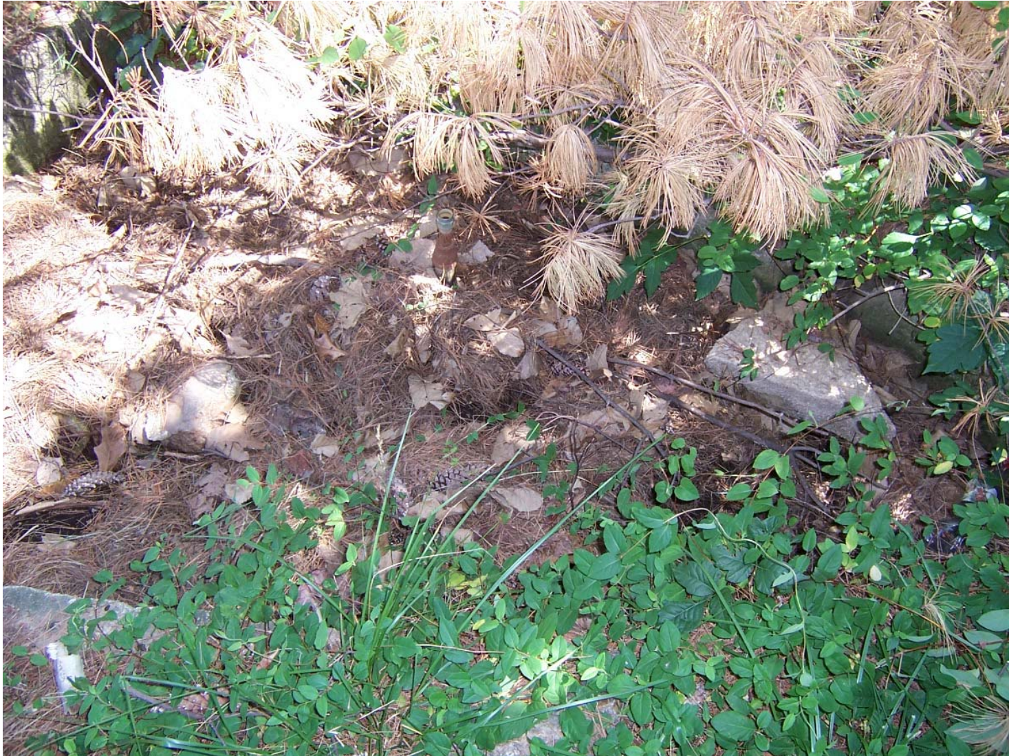
Existing Condition Photo B87: Stempson House Site Landscape Water Feature
