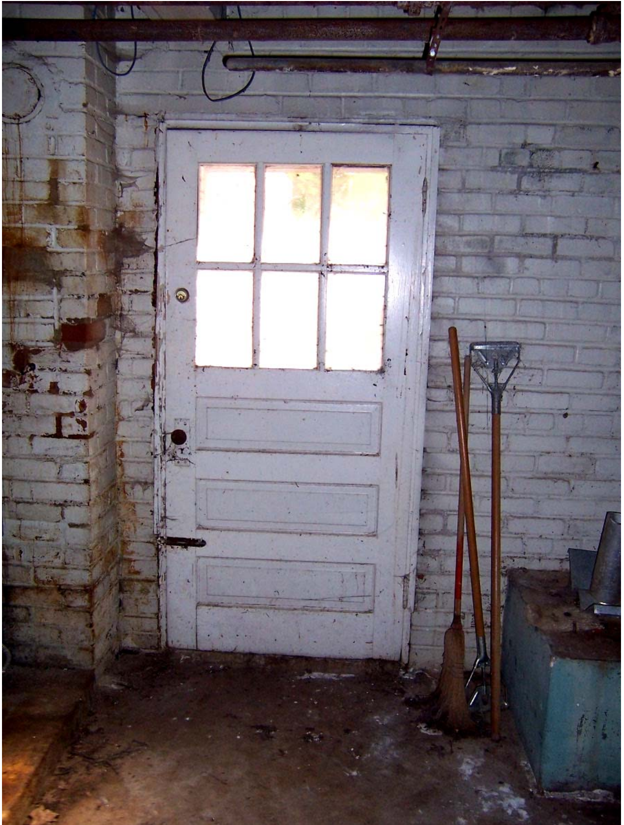
Existing Condition Photo B24: Stempson House Basement Exterior Door (D01)
