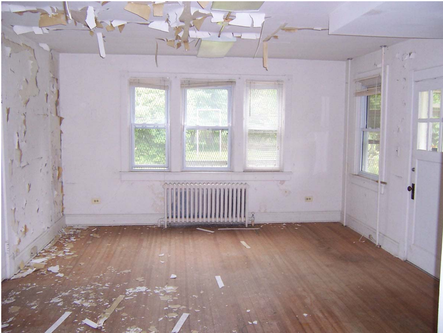
Existing Condition Photo B42: Stempson House First Floor Room 103
