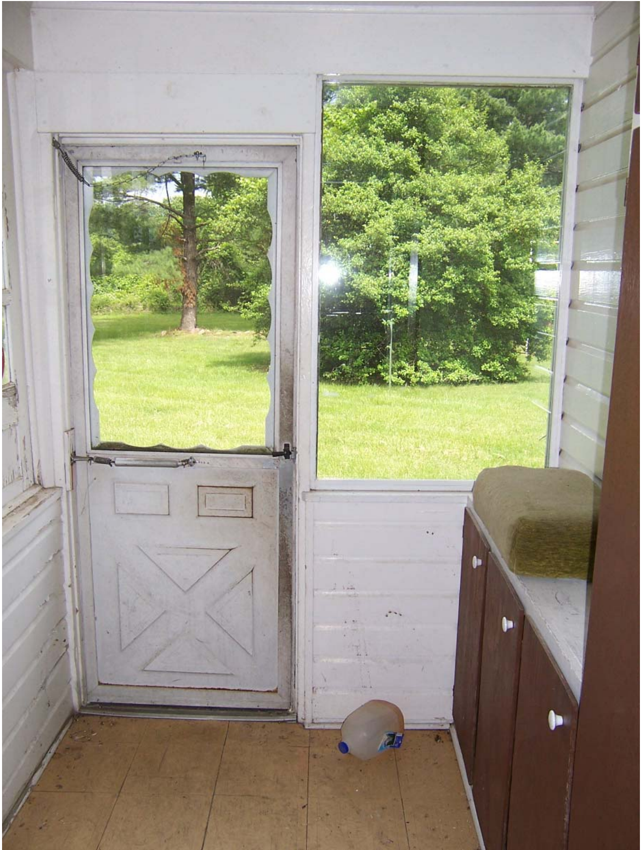
Existing Condition Photo B45: Stempson House First Floor Vestibule (Room 104)
