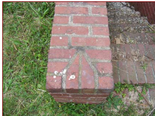
Image 3.13: Stair Well Detail
