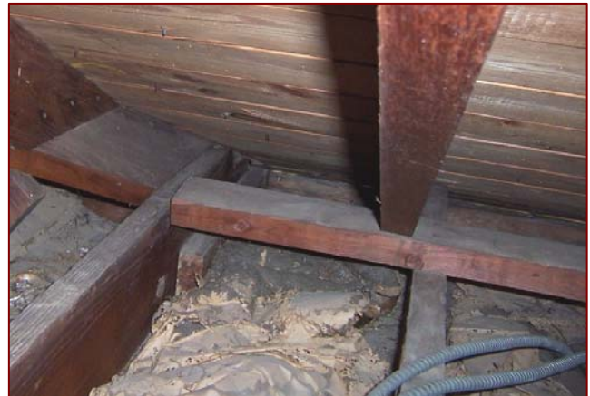
Image 3.28: Rafter and False Plate at Eave
