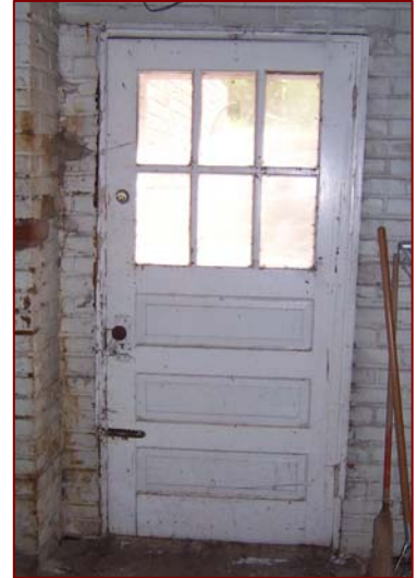
Image 3.96: Exterior Basement Door
