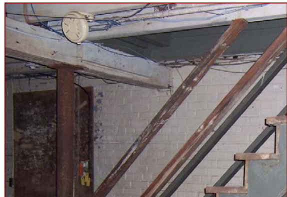
Image 3.26: Support Beam in Basement
