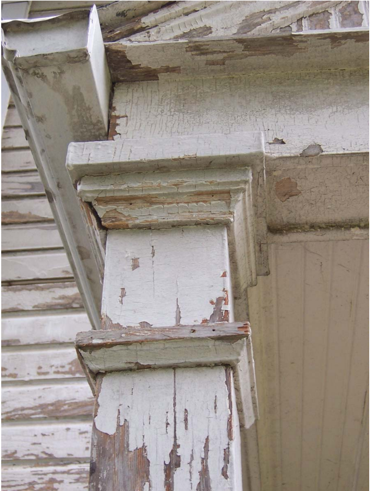
Existing Condition Photo B06: Stempson House Exterior West Porch Column Detail
