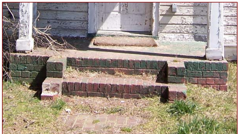
Image 3.18: Brick Entry-Portico Floor and Brick Walkway
