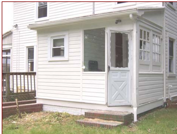
Image 3.64: Exterior of Vestibule (Room 104) and Toilet Room (Room 105)
