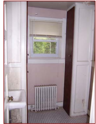
Image 3.65: Toilet Room (Room 105)
