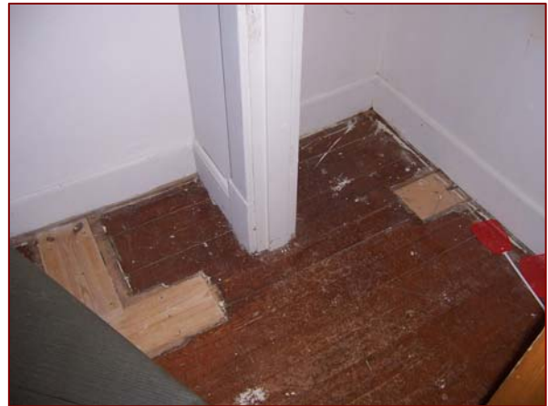
Image 3.109: Evidence of Original Closet Location
