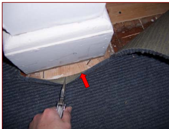
Image 3.107: Flooring Infill at Previous Wall Location
