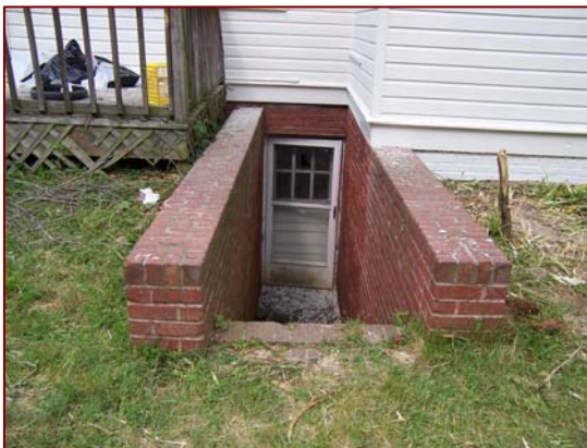
Image 3.12: Brick Stair Well
