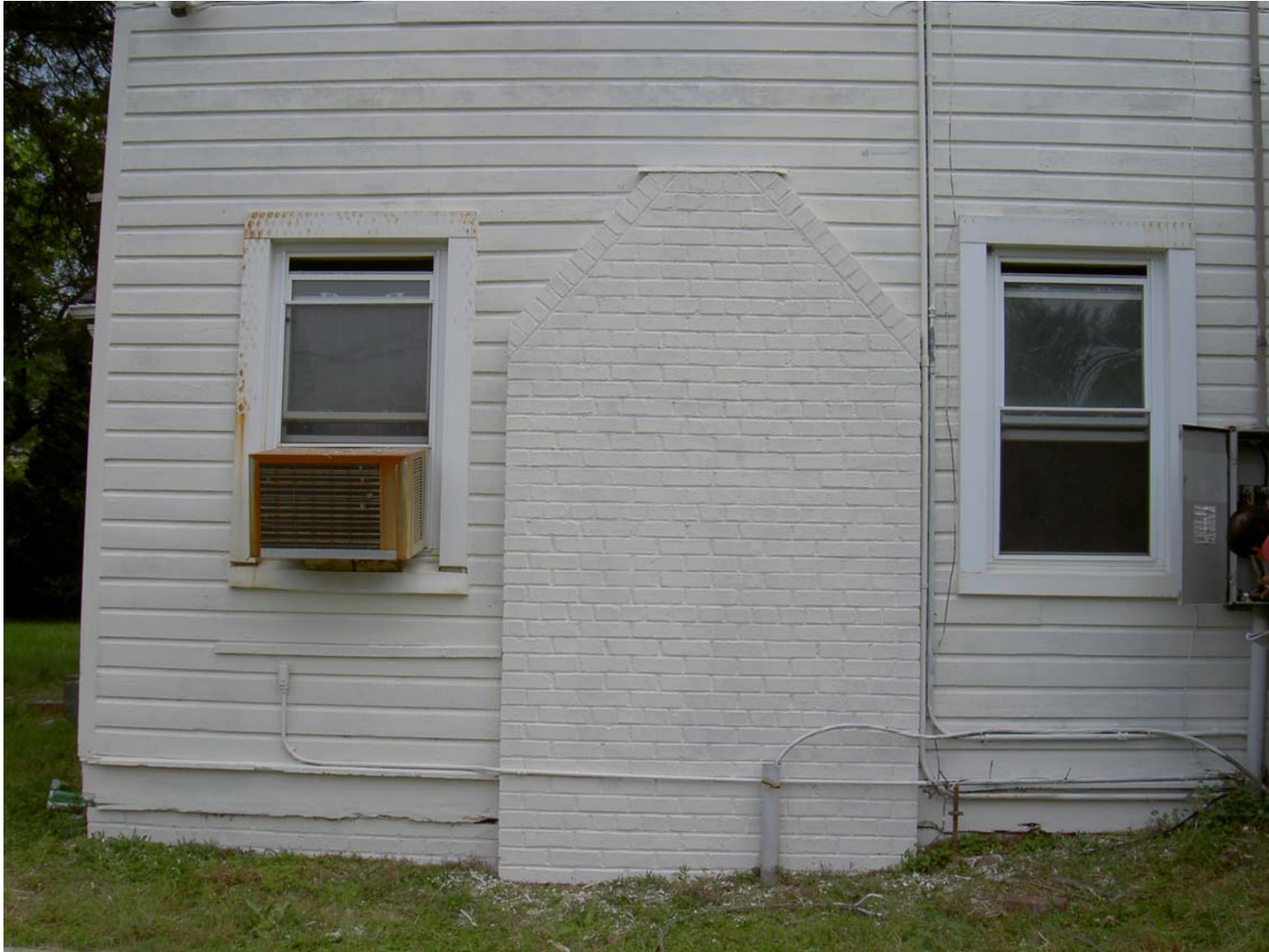
Existing Condition Photo B7: Stempson House Exterior Partially Exposed Brick Fireplace
