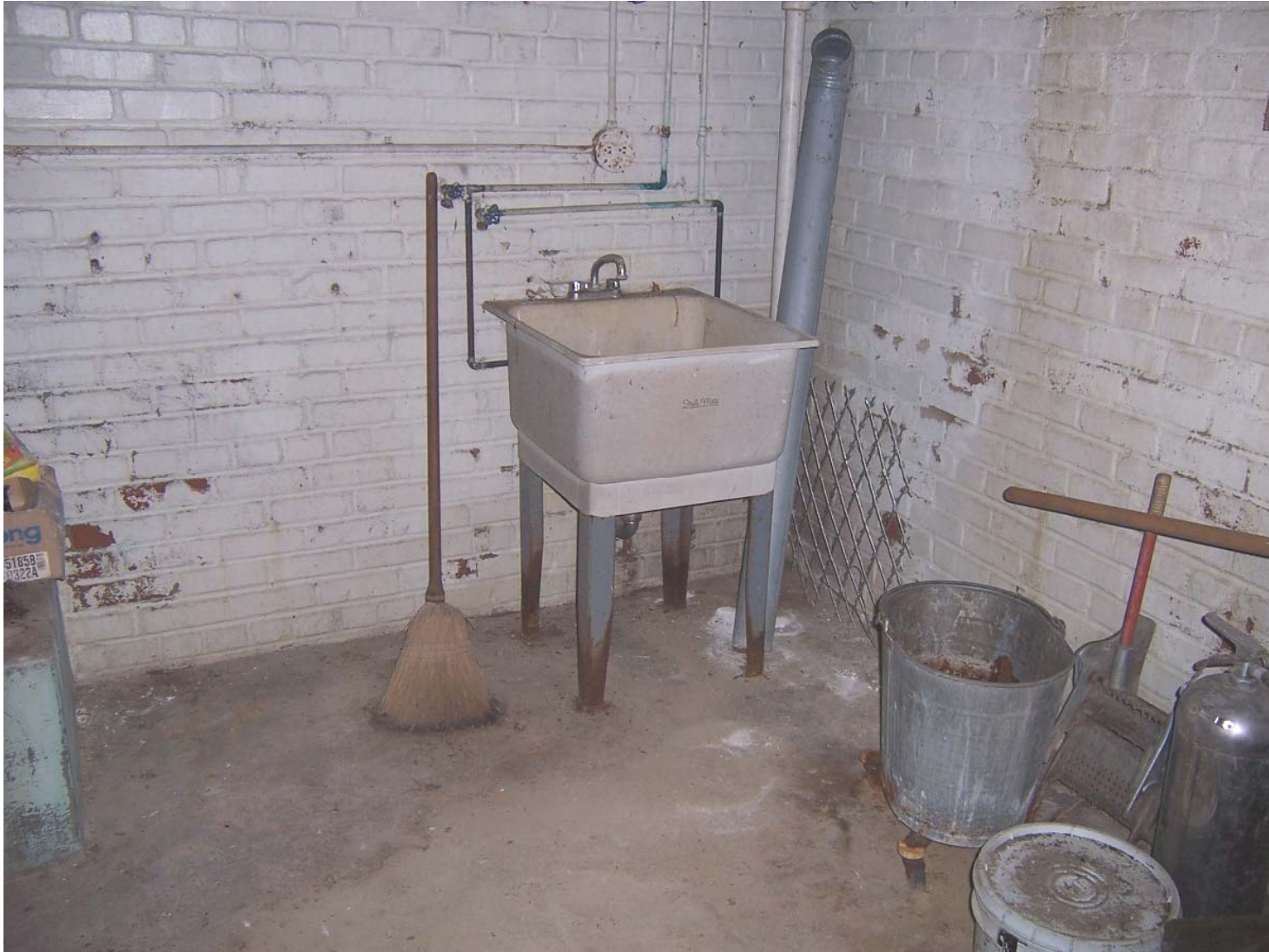
Existing Condition Photo B22: Stempson House Basement Basement Laundry Tub
