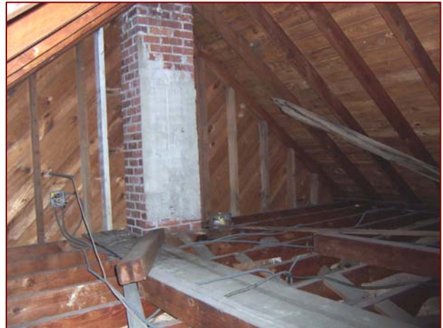
Image 3.25: Southern Chimney Within Attic
