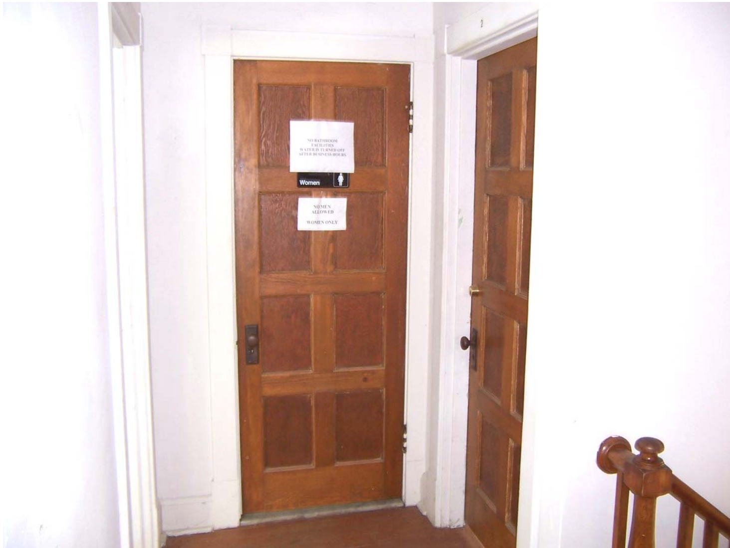
Existing Condition Photo B68: Stempson House Second Floor Hall (Room 204)
