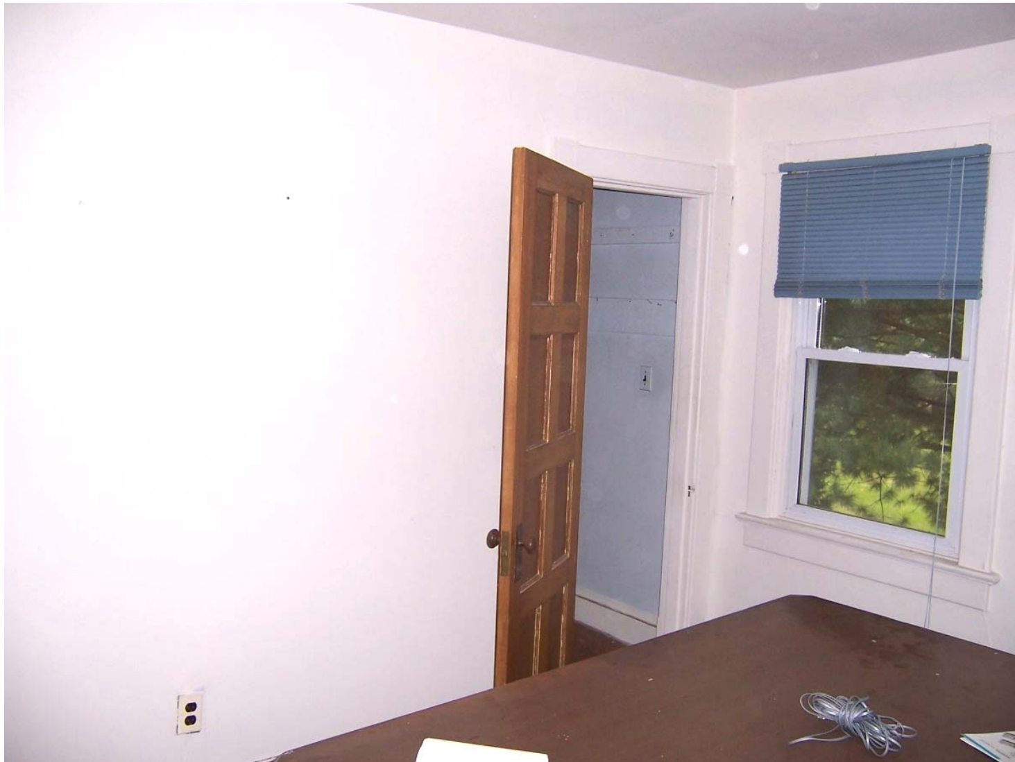
Existing Condition Photo B65: Stempson House Second Floor Bedroom/Office (Room 203)
