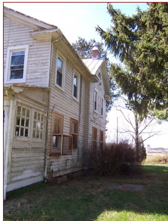
Image 3.2: Metal Window Guards at First Floor
