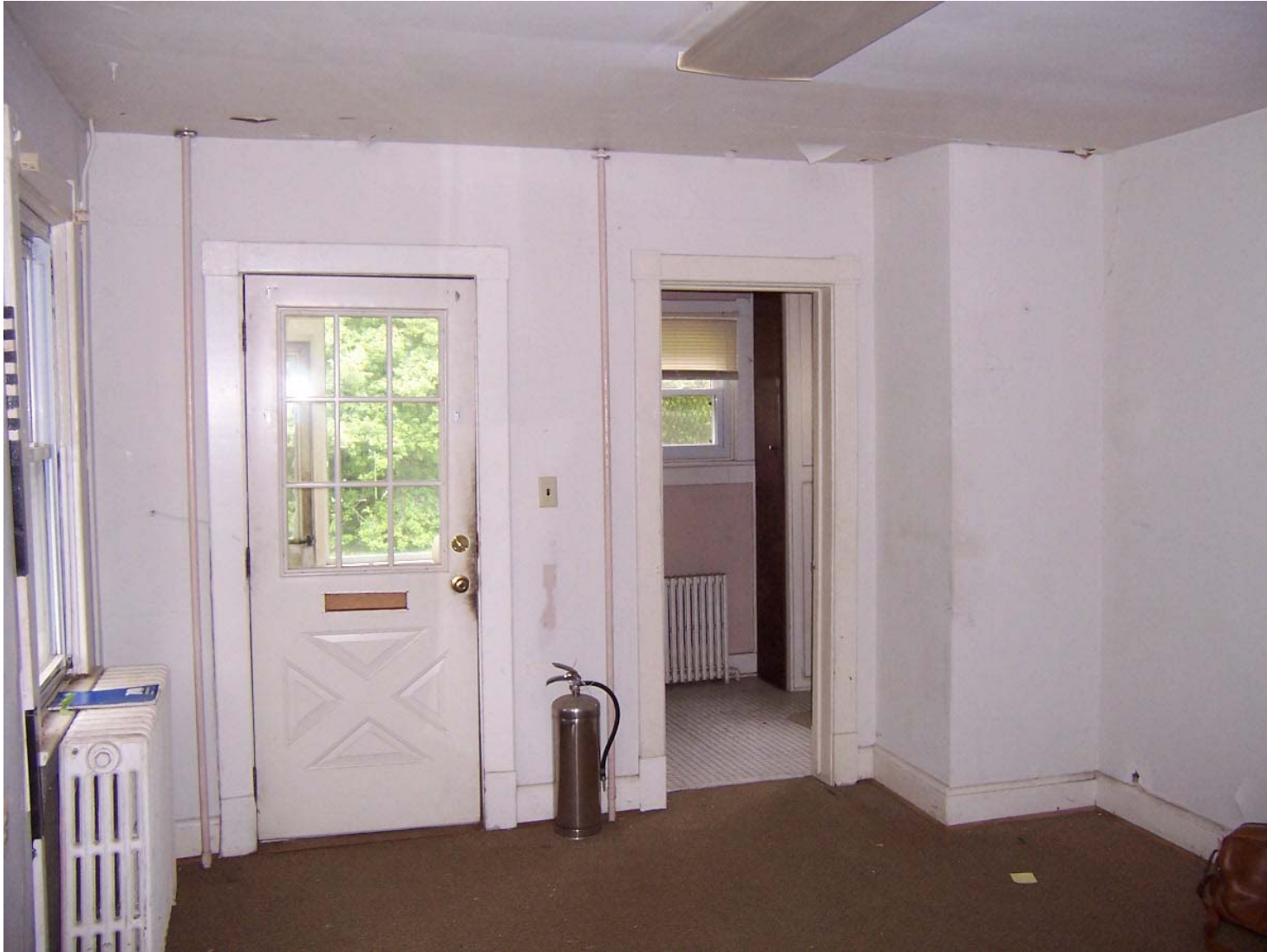
Existing Condition Photo B36: Stempson House First Floor Kitchen (Room 102)
