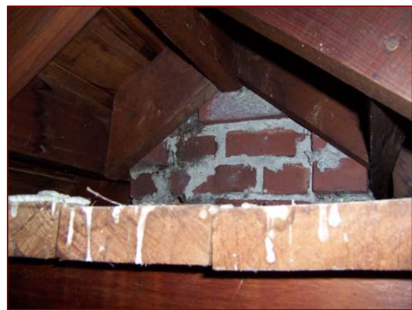
Image 3.22: Northern Chimney on Platform
