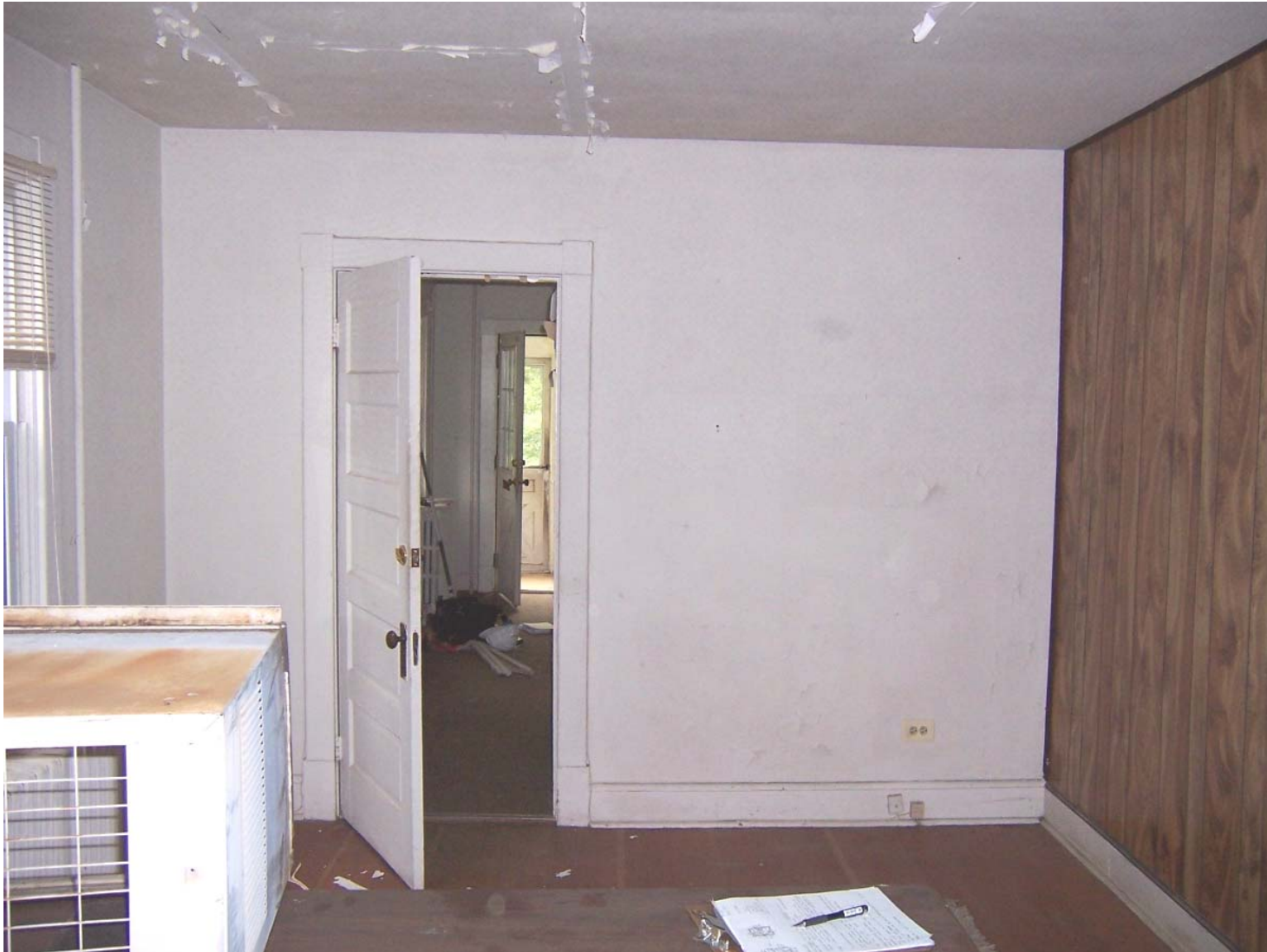
Existing Condition Photo B33: Stempson House First Floor Room 101
