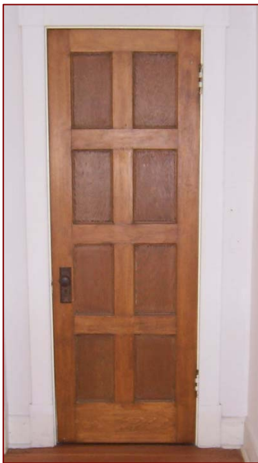
Image 3.5: Second-floor Door With Plywood Panels
