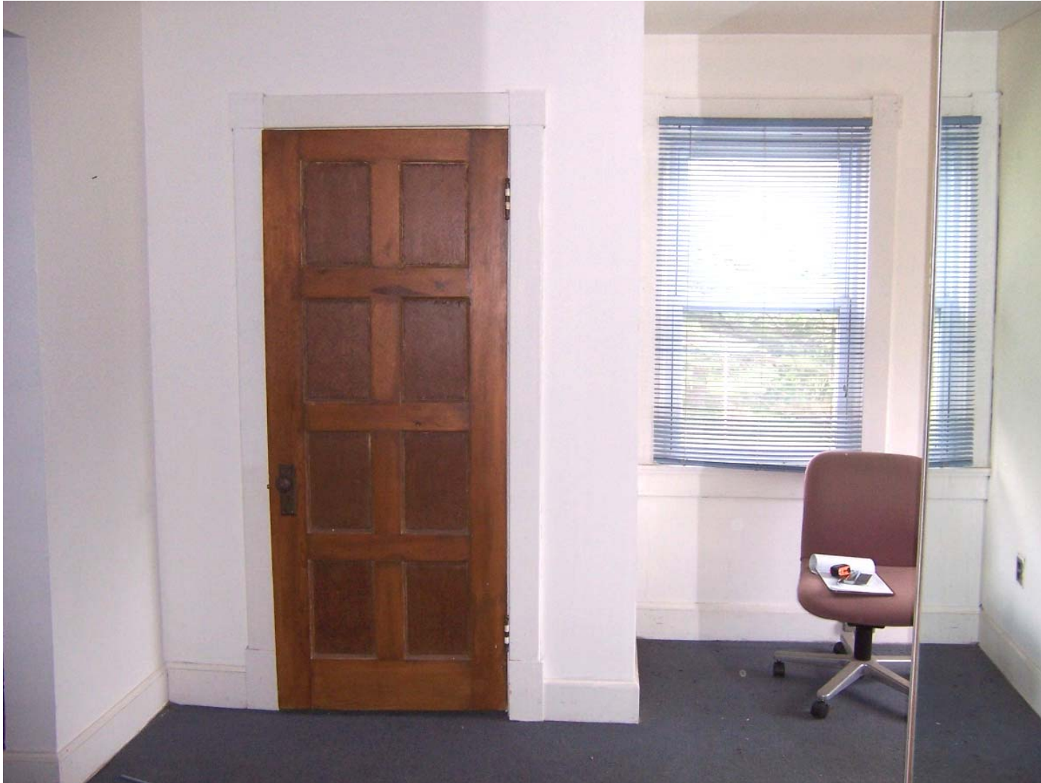
Existing Condition Photo B63: Stempson House Second Floor Bedroom/Office (Room 203)
