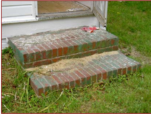
Image 3.19: Eastern Porch Steps
