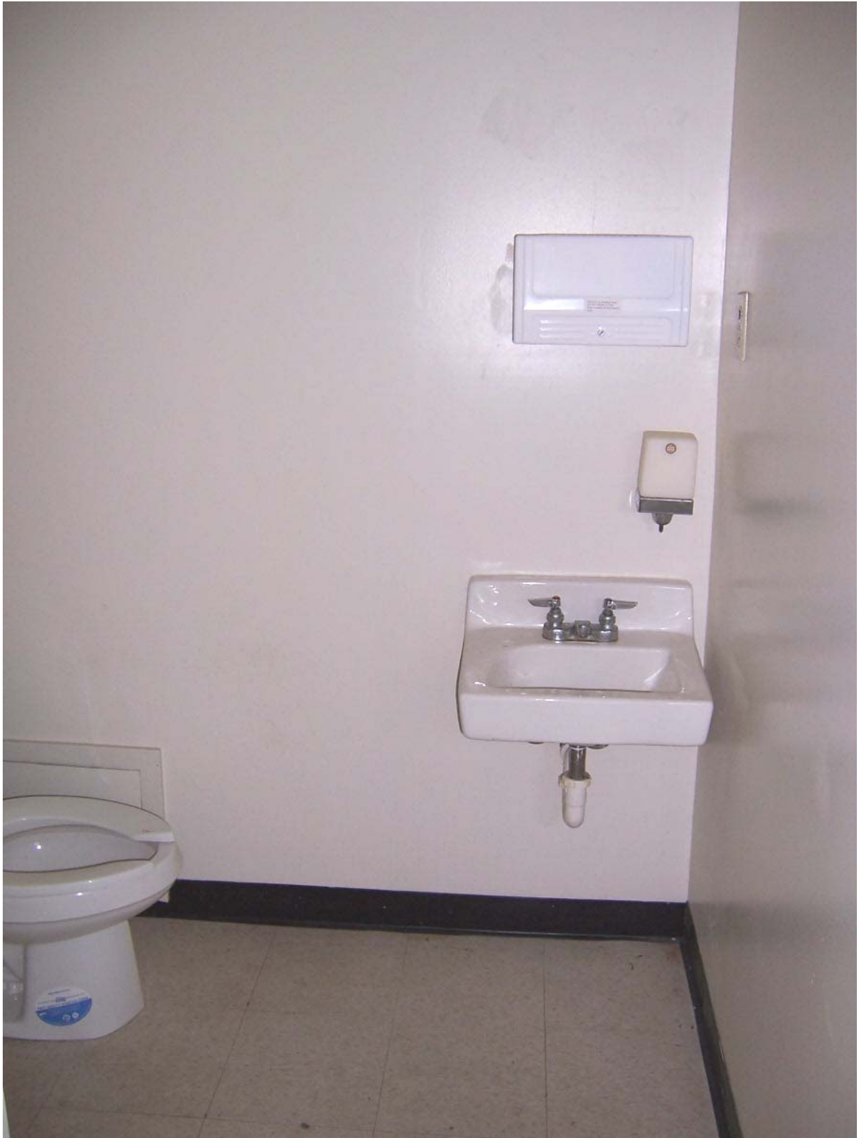
Existing Condition Photo B72: Stempson House Second Floor Toilet Room (Room 206)
