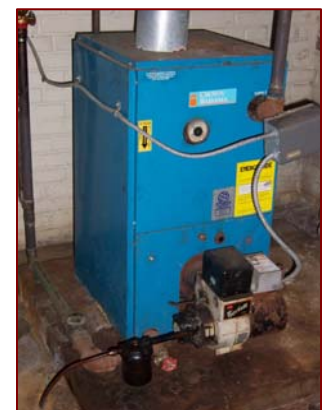
Image 3.15: Oil-fired Boiler
