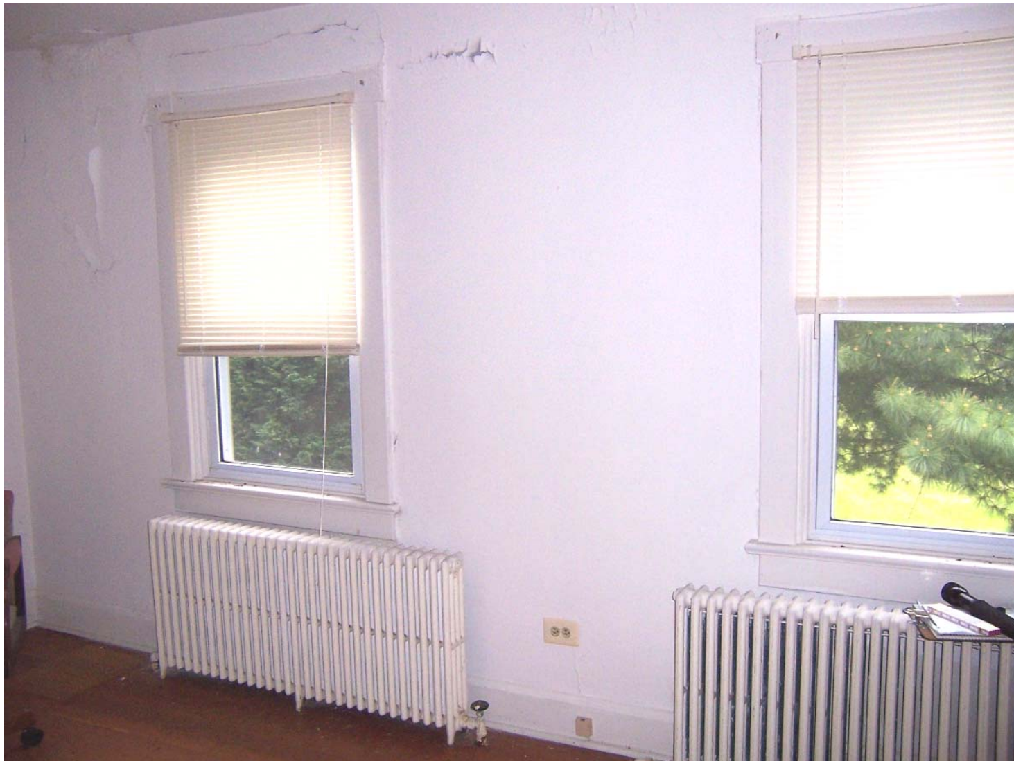
Existing Condition Photo B60: Stempson House Second Floor Bedroom (Room 201)
