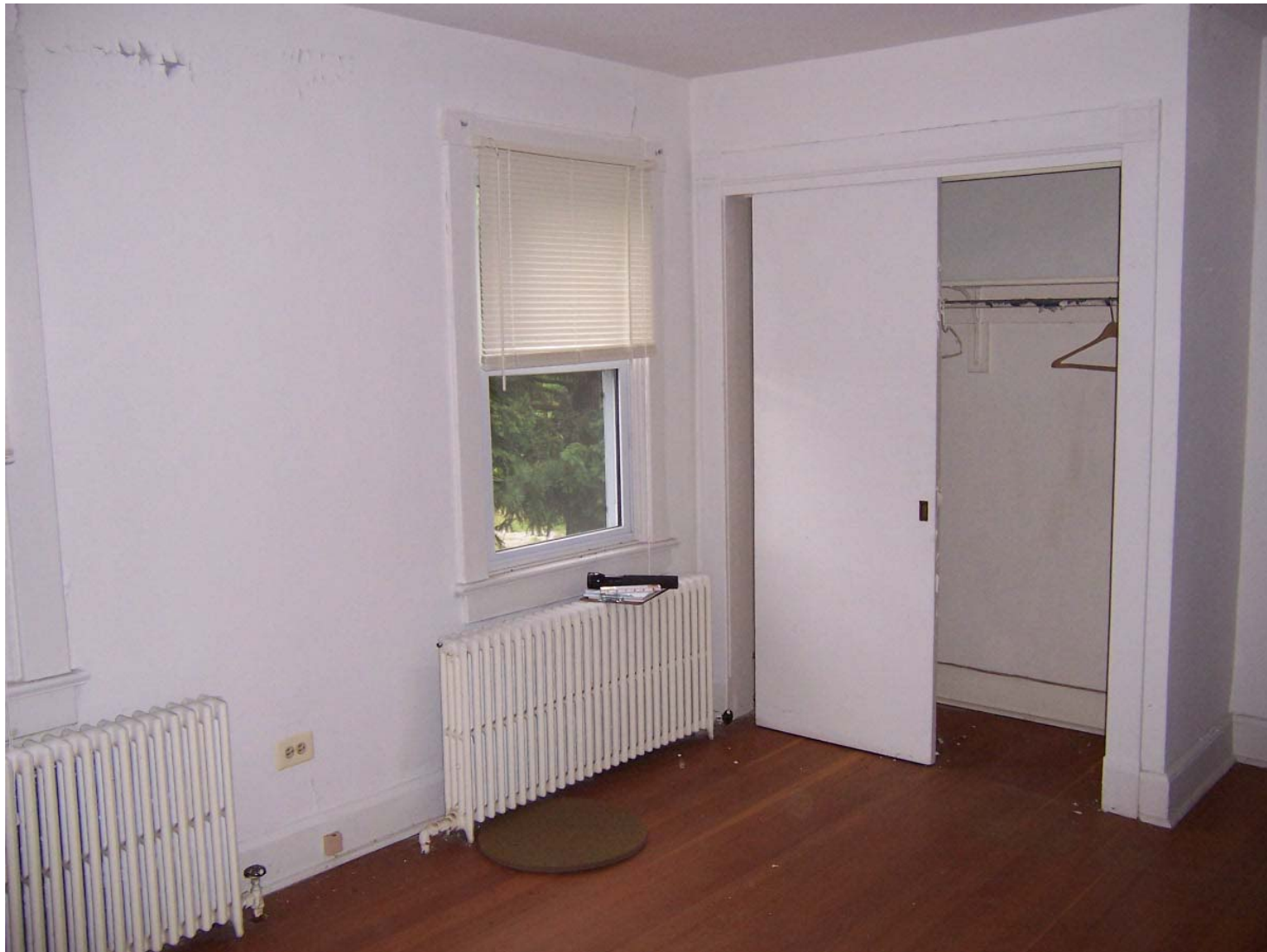
Existing Condition Photo B58: Stempson House Second Floor Bedroom (Room 201)
