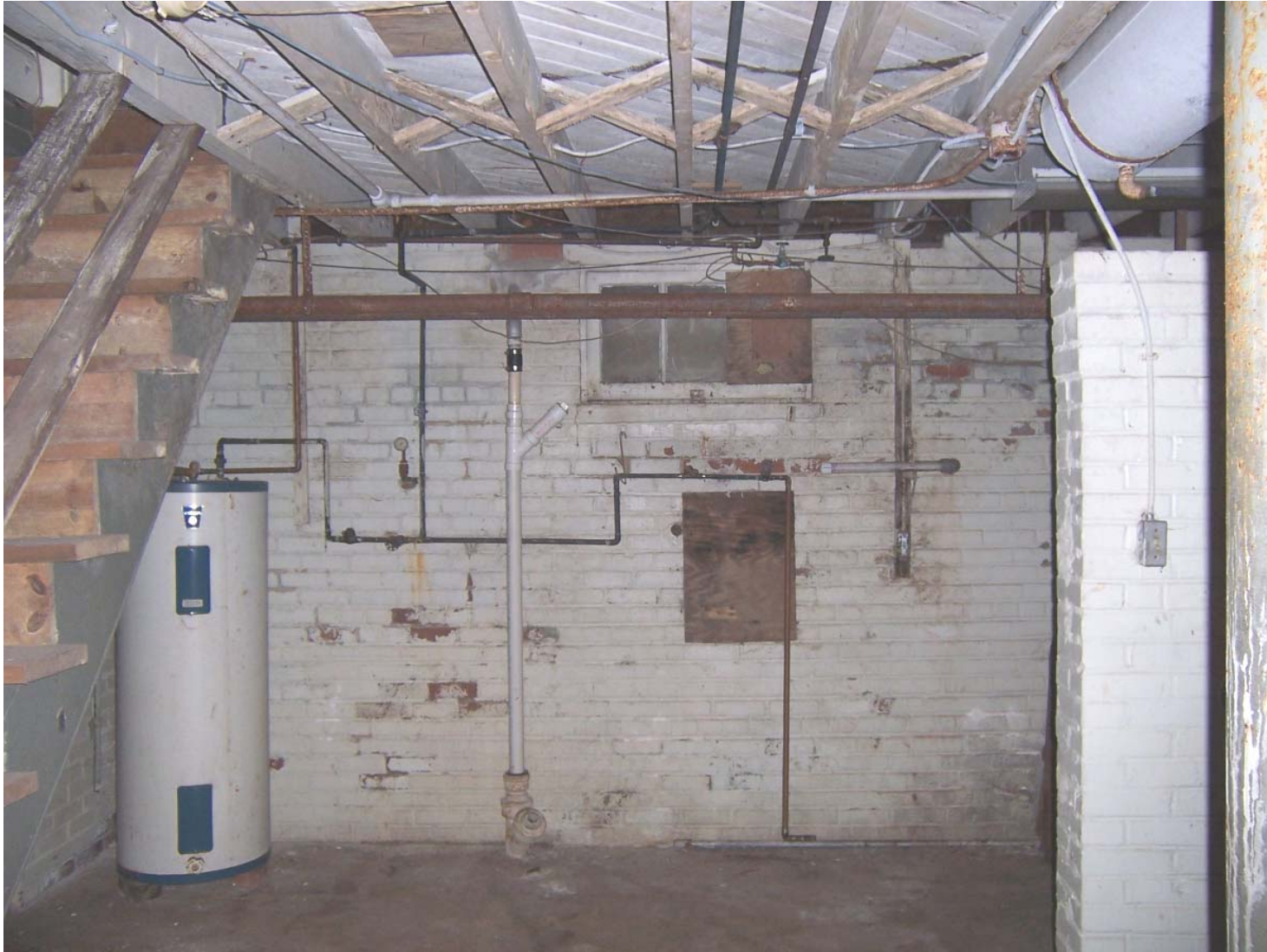
Existing Condition Photo B19: Stempson House Basement Basement Room B4
