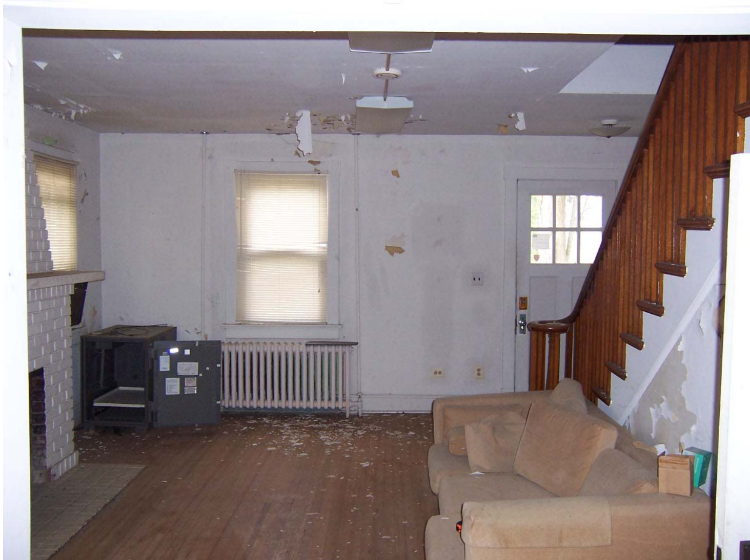
Existing Condition Photo B25: Stempson House First Floor Living Room (Room 100)
