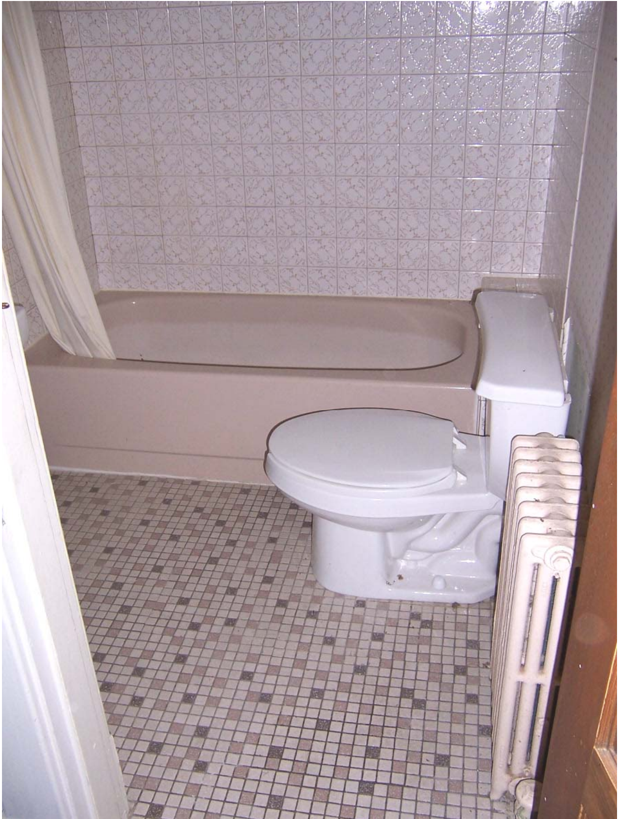
Existing Condition Photo B70: Stempson House Second Floor Bathroom (Room 205)
