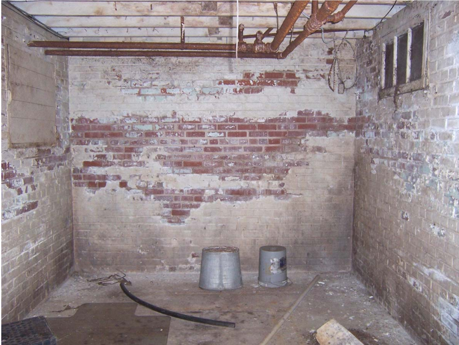
Existing Condition Photo B17: Stempson House Basement Basement Room B3
