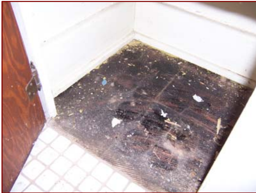
Image 3.99: Evidence of 9x9 Floor Tiles in Toilet Room Closet
