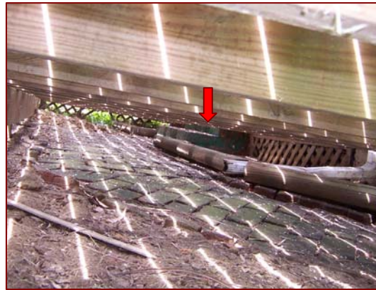
Image 3.20: Southern Porch Steps and Walkway Beneath Wood Deck
