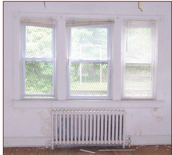
Image 3.32: Windows in Room 103
