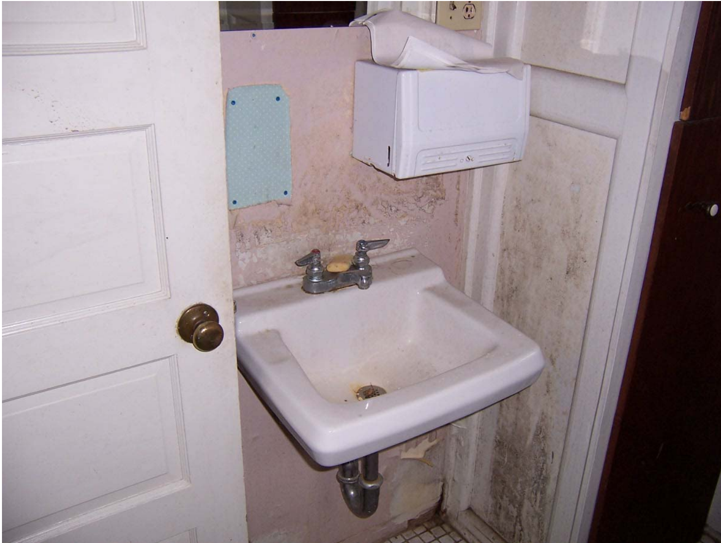
Existing Condition Photo B51: Stempson House First Floor Lavatory (Toilet Room 105)
