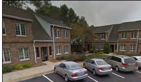
Office units along Bowman Green Drive
