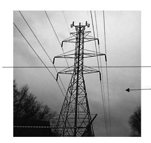
A "Fort Worth" structure integrates the telecommunication pole and antennas within an existing electrical transmission tower
