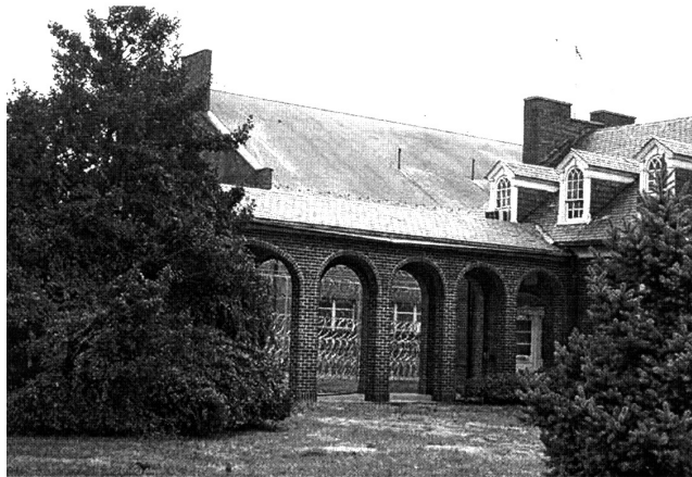
VIEW FROM ROUTE 123 OF THE ADMINISTRATIVE BUILDING AND THE OCCOQUAN FACILITY
