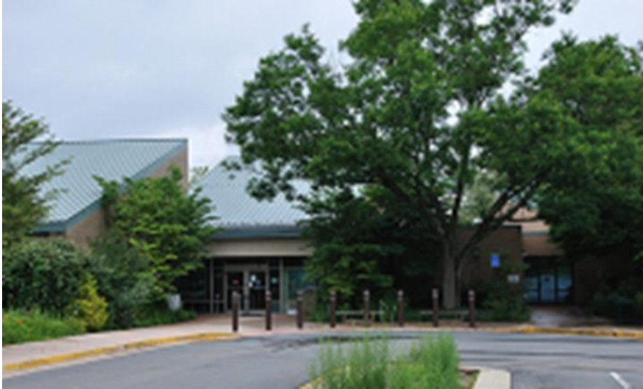
Kings Park Community Library (Braddock District)
