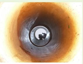
Photo 4 - Standing water observed inside observation well for more than 48 hours.
