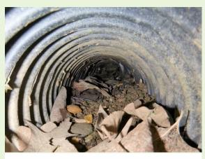
Photo 2 - Inflow pipe blocked by debris and sediment.
