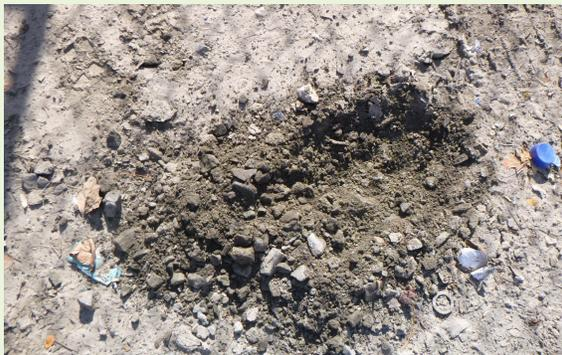
Photo 3 - Surface gravel clogged by excessive sediment.
