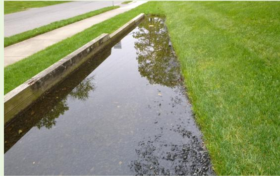
Photo 2 - Ponding water in the facility for more than 48 hours.
