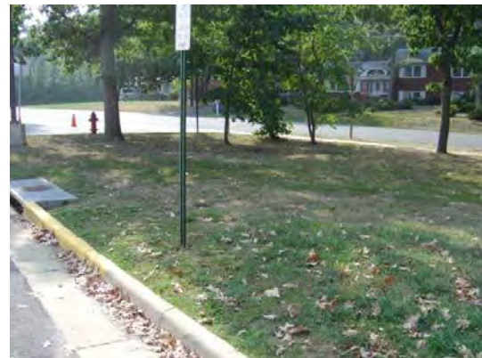
Add bioretention areas in this traffic island, and replace inlet with a tree box filter
