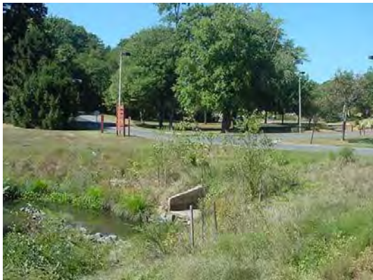
Existing stormwater pond with roadway in background
