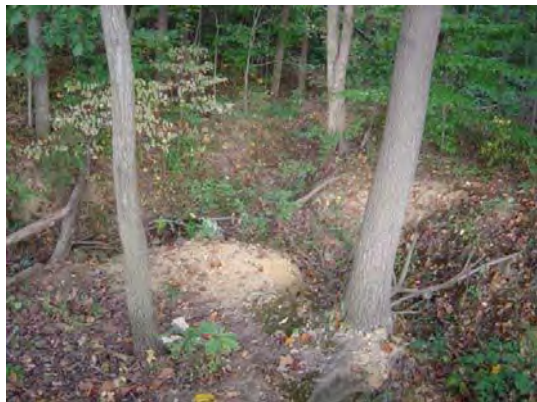
Eroded cut along streambank
