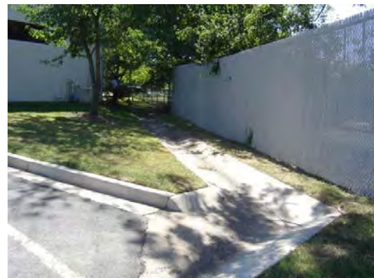
Convert concrete swale to linear bioretention area along NW side of building
