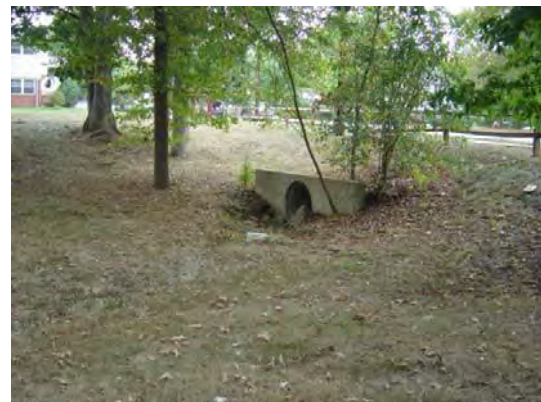
Stormwater pipe inlet at Deepford St where bioretention area could be utilized
