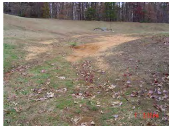
Stressed vegetation in existing grass swale on property
