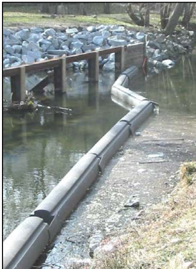
Trash skimmer on Tripps Run before it enters Lake Barcroft
