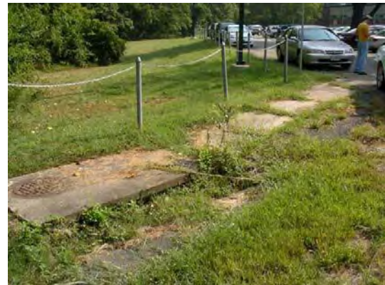
Potential bioretention area at stormwater inlet
