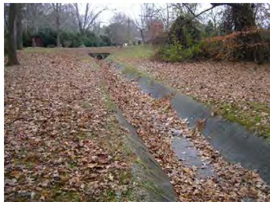
Ditch and outfall
