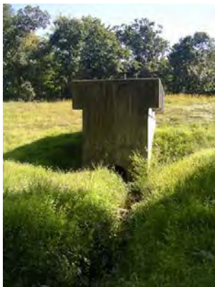
SWM pond control structure
