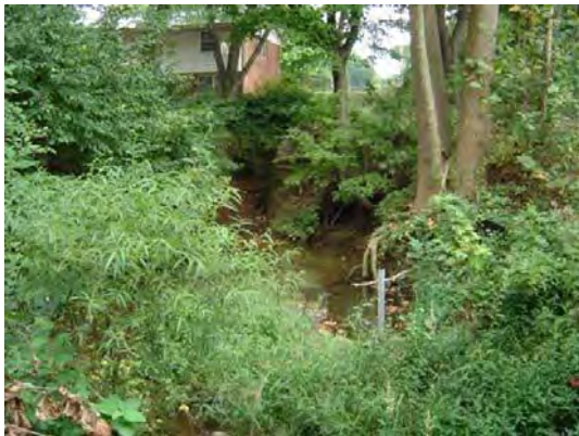
Existing stormwater pond
