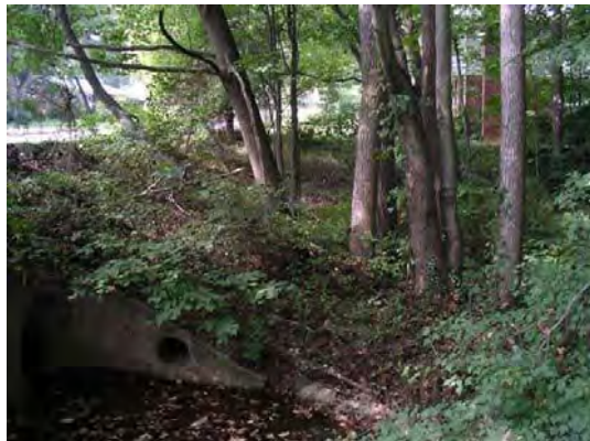
Stormwater pipe outfall
