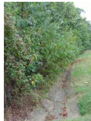
Concrete ditch behind houses
