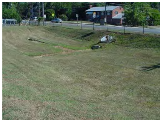
Dry pond with outlets and inlet structure
