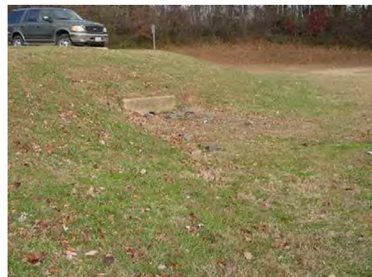
Potential bioretention area at stormwater outlet
