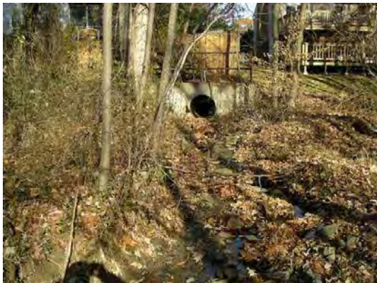
Outfall at end of Trail Run Road
