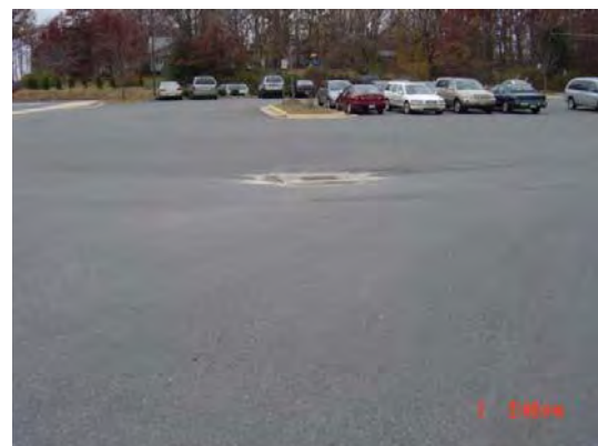
Inlet in east parking lot
