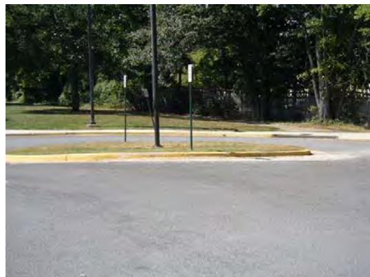
Potential bioretention area in traffic island
