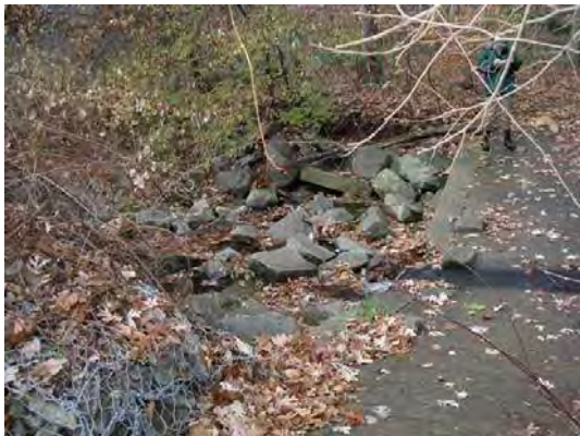
Concrete ford to be notched
