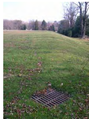
Grate inlet on athletic field could be surrounded by a rain garden
