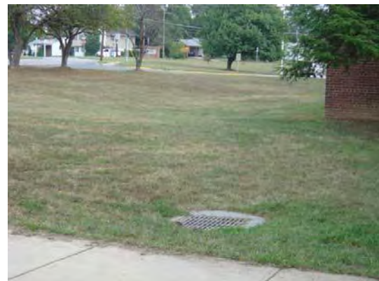
Inlet in grassy area where bioretention area could be installed. Note parking lot island in background where bioretention can be used
