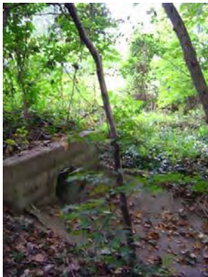
View of spillway
