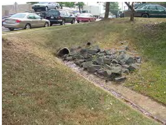
Concrete ditch below roadway
