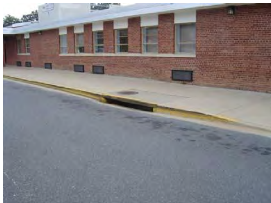
Inlet in front of school where tree box filter could be installed
