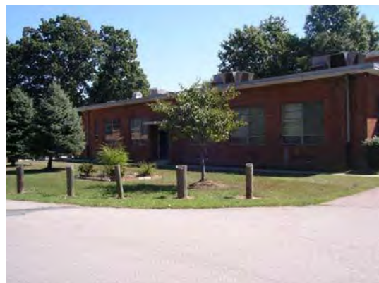
Potential bioretention area along NW corner of school
