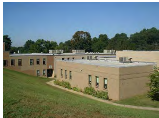
Potential bioretention areas located behind school building
