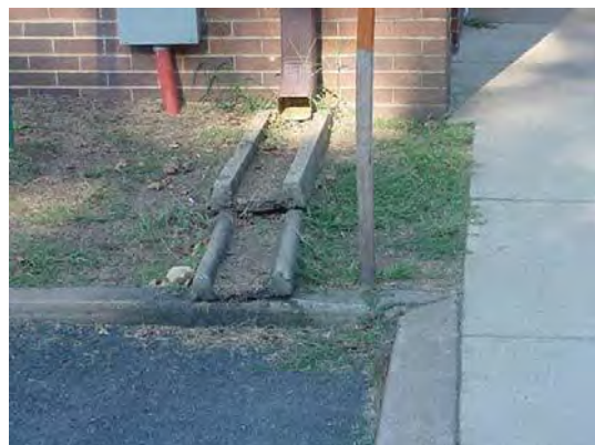
Rain gutter on side of building
