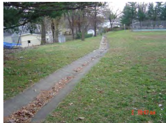
Convert concrete ditch to linear bioretention area
