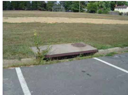
Inlet in parking lot where tree box could be installed
