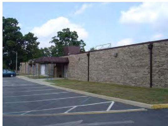
Roof drains at Fire Station can be diverted to cistern for filling fire trucks
