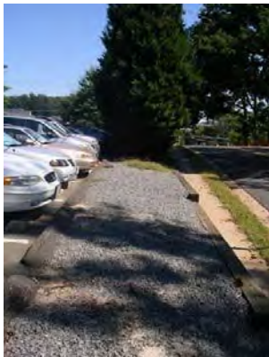
Existing infiltration trench alongside parking lot
