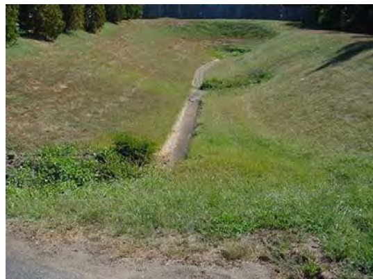
SWM dry pond
