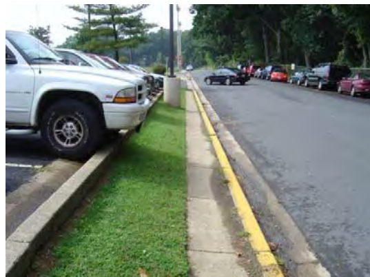
Partial sidewalk along Four Year Run could be converted to a grass filter strip
