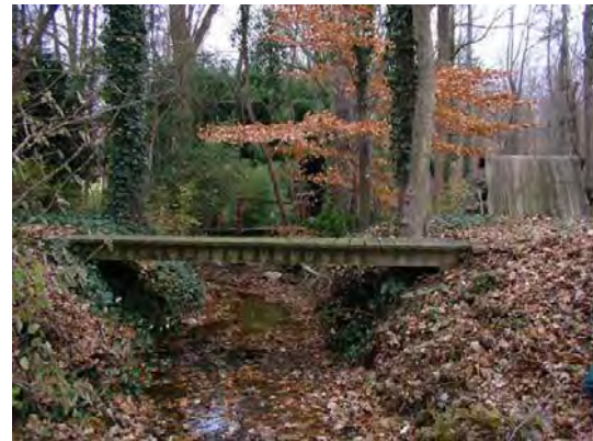
Streambanks to be stabilized and buffers planted to reestablish connection with floodplain
