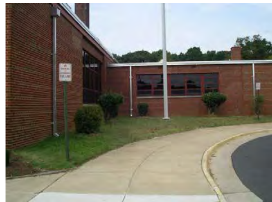
Divert downspouts into bioretention areas alongside building
