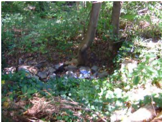
Stormwater pipe outfall
