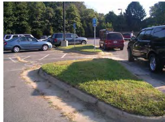
Convert traffic islands in parking lot to bioretention areas
