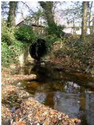
Stormwater pipe outfall
