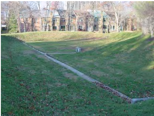
SWM dry pond
