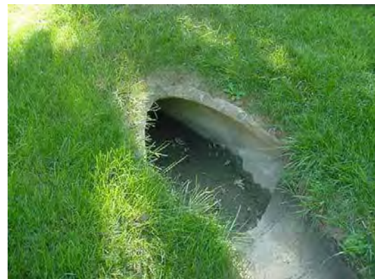
Outlet entering swale
