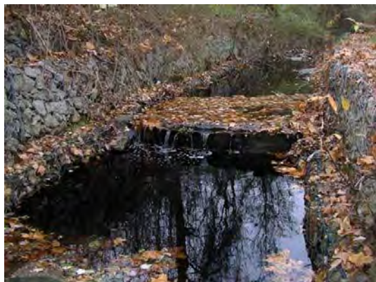
Stream lined with gabion baskets and concrete weirs
