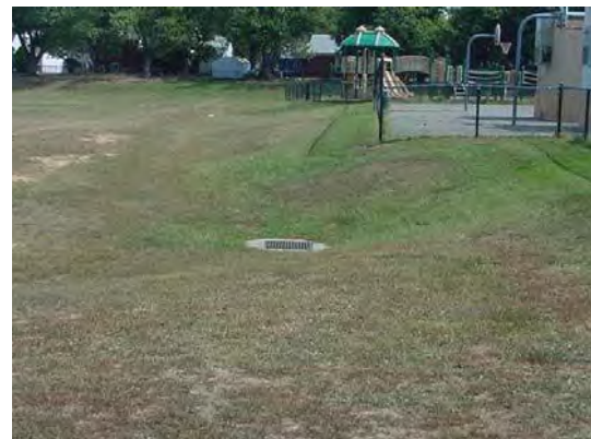
Stormwater inlet in lawn
