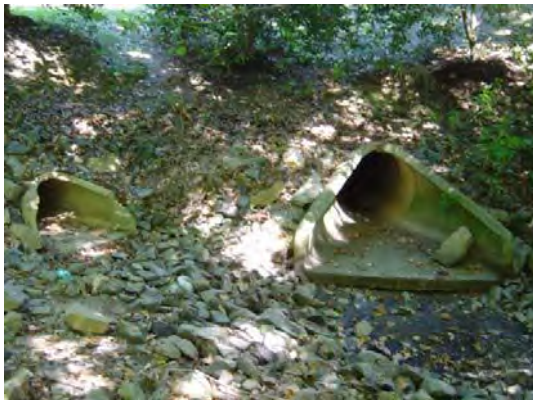
Potential bioretention area at end of stormwater outfalls
