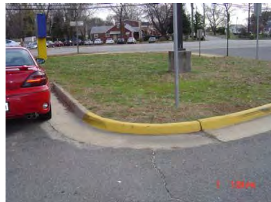
Potential bioretention area in traffic island
