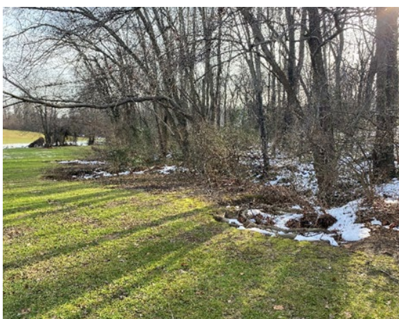
Sheet flow off lawn increasing erosion along the left bank of stream segment 0065-009.
