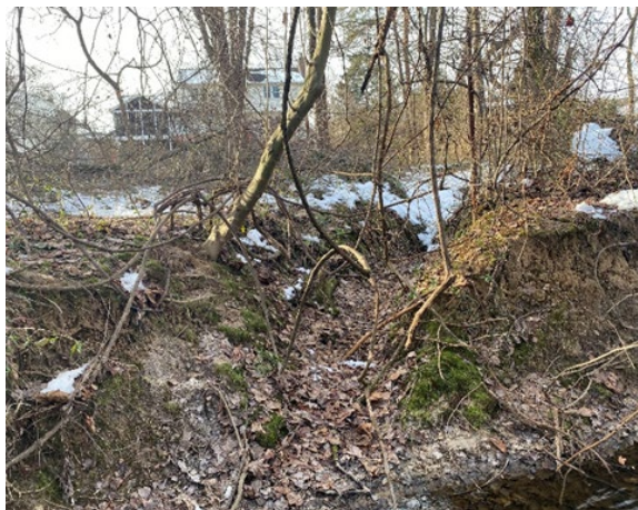
Widening outfall channel.
