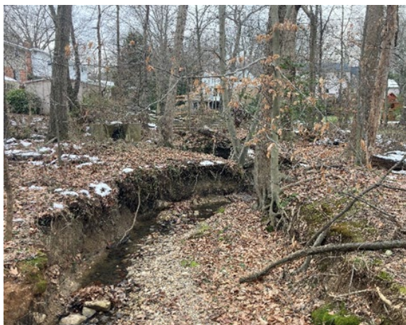
Widening outfall channel.
