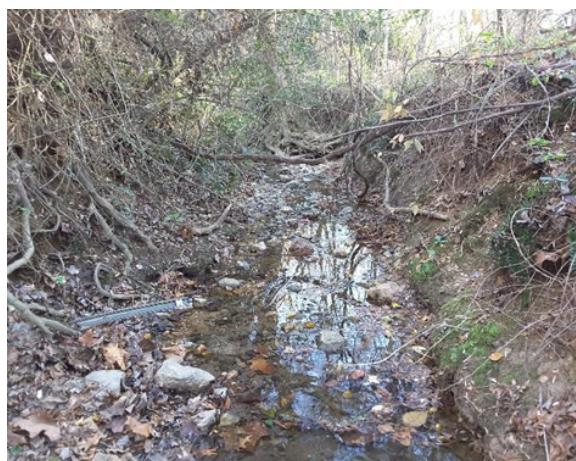
Example of a widening outfall channel.
