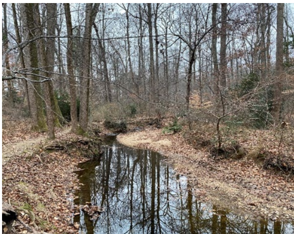
Widening channel with sediment deposition.
