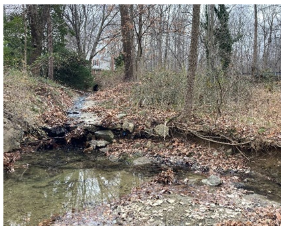
Concrete outfall channel discharging into widening natural channel.
