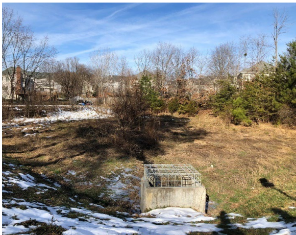
Channel entering riser, trees on pond embankment and vegetation in basin.
