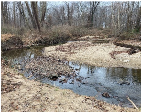
Widening stream channel; large supply of streambed material.
