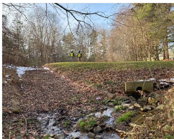
BMP-02 outfall and emergency spillway discharges into stream segment 0065-009.
