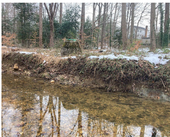
Trail culverts discharging into stream segment.
