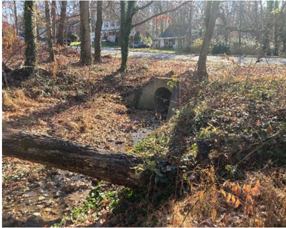
Stream segment entering the downstream culvert that passes under Braeburn Drive.
