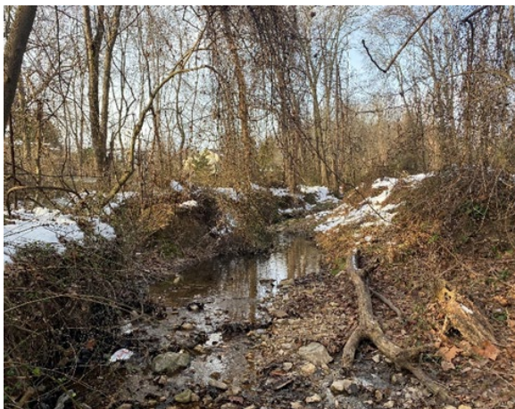
Widening channel with significant invasive species.
