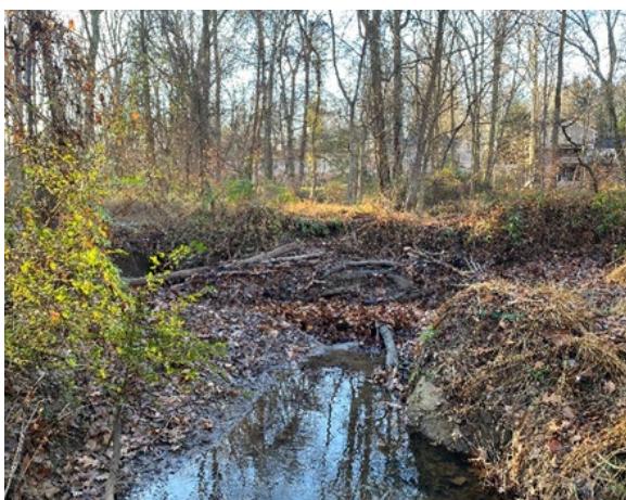
Debris blockage and exposed sewer manhole.
