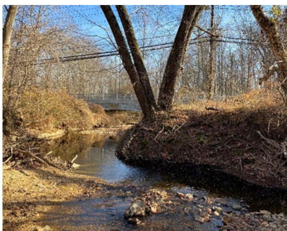
Overhead electric lines and road bridge at end of stream segment 0030-008.
