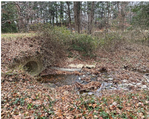
Exposed sewer encasement.
