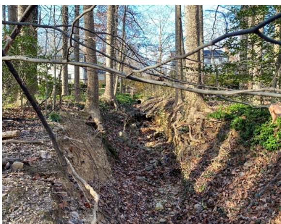
Widening outfall channel.
