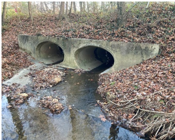
Double culvert at downstream project limits.
