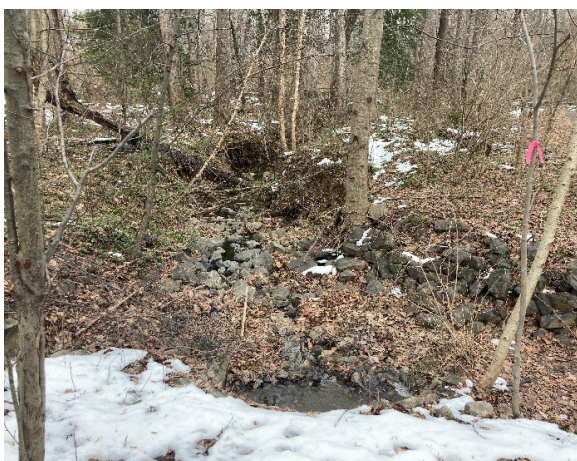
Incised outfall channel.
