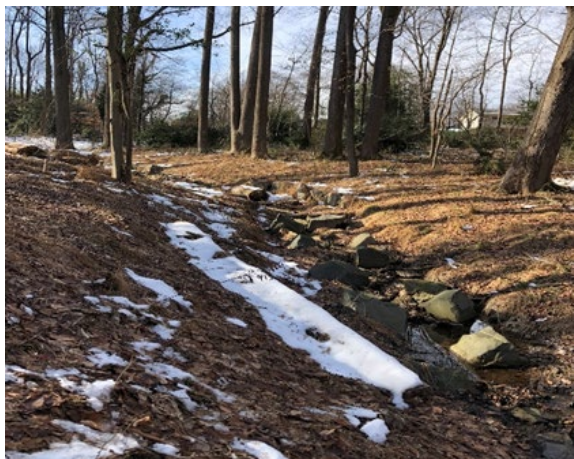
Restored upstream channel.
