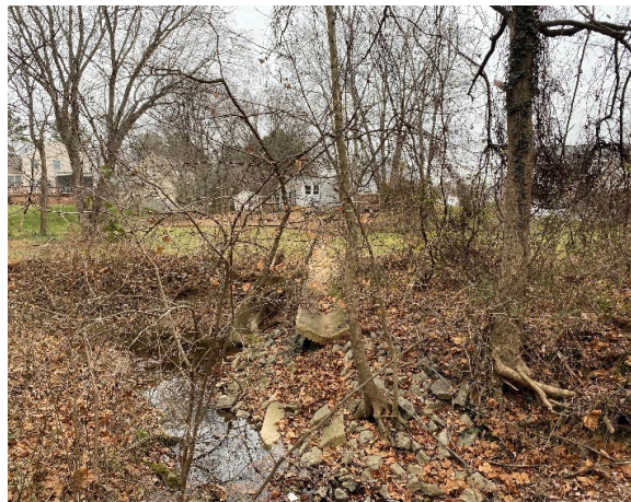
Paved outfall ditch discharging into stream.
