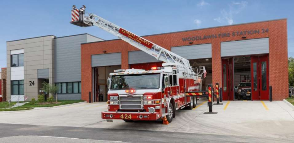
Woodlawn Fire Station – Alexandria, VA
