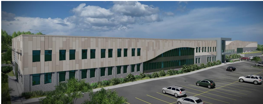
Building 1 – North Façade Main Entrance
