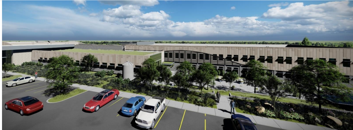
Building 1 – South Façade Front Elevation
