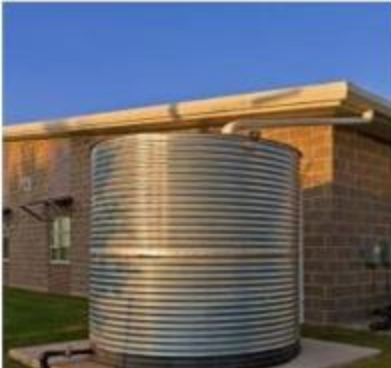
Stormwater Cistern
