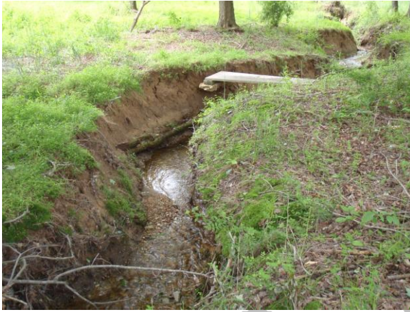
Figure 2-8: Bank erosion in excess of 3ft on small tributary near Cedar Ridge Drive
