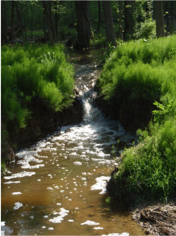
Figure 2-36: Approximately 2ft headcut in tributary upstream of regional pond R17
