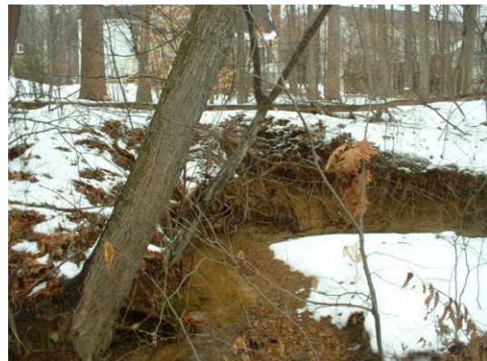
Figure 2-28: Erosion area on Willow Springs Branch upstream of Ashleigh Road
