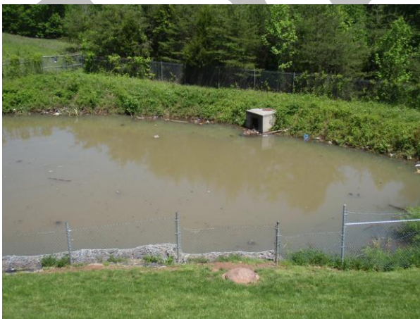
Figure 2-25: Wet Pond with significant amount of litter near Compton Valley Way
