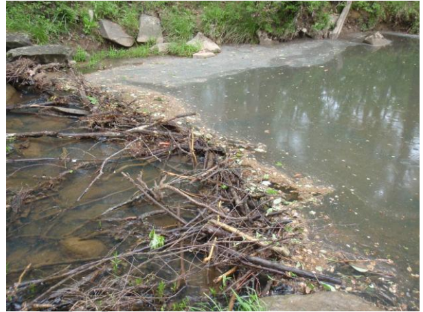
Figure 2-24: Debris obstruction in main stem of Little Rocky Run
