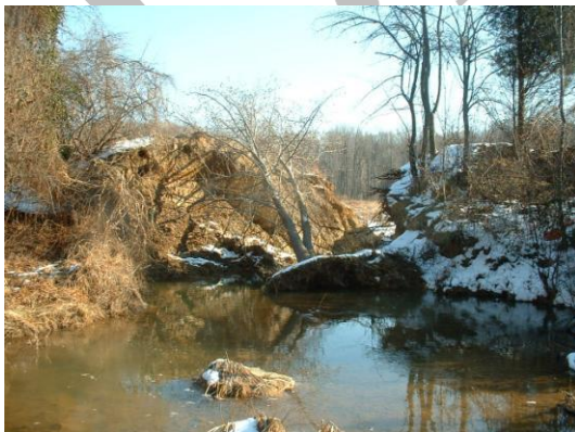
Figure 2-27: Erosion area on Little Rocky Run upstream of Willow Springs Branch
