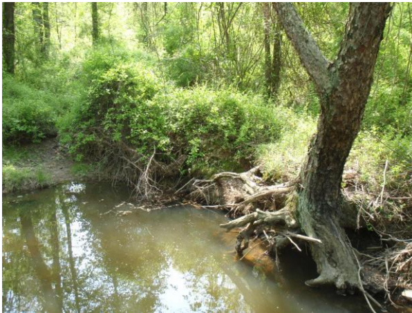
Figure 2-33: Severe erosion on Little Rocky upstream of Stringfellow Road
