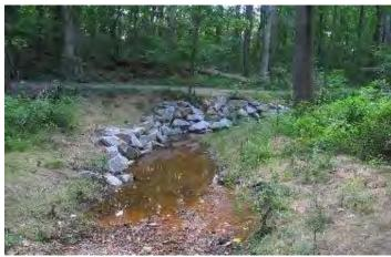
Figure 4: Typical riprap bank protection (VA DEQ)
