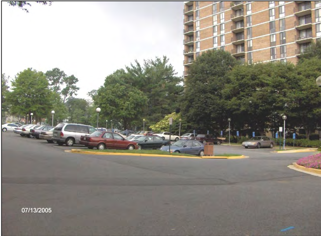
Site Photo: Looking west from the side parking lot
