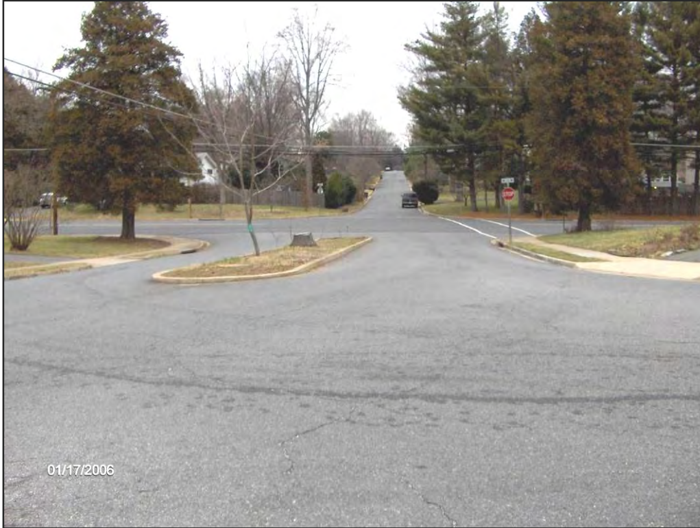
Site Photo: Roadside area suitable for bioretention in the Devon Park Neighborhood
