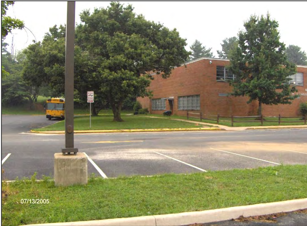
Site Photo: Looking south towards the school from the parking lot
