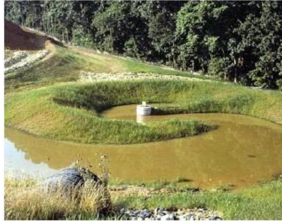
Photo 4.1 Extended Detention Basin Full of Stormwater
