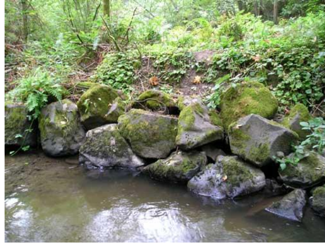
Photo 4.13 Boulder Revetment Source: Center for Watershed Protection
