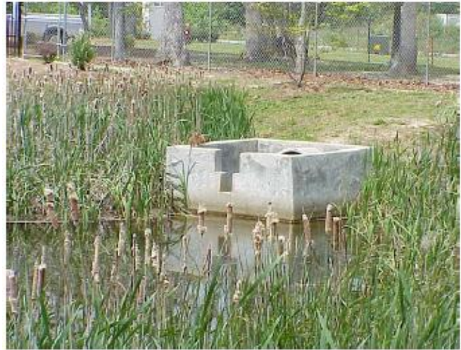
Photo 4.2 Enhanced Extended Detention Basin Full of Stormwater Source: Virginia Stormwater Management Handbook
