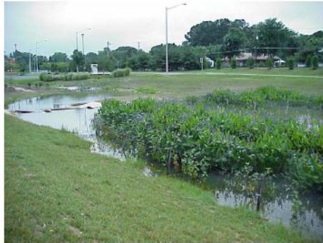
Photo 4.4 Constructed Stormwater Wetlands Source: Virginia Stormwater Management Handbook
