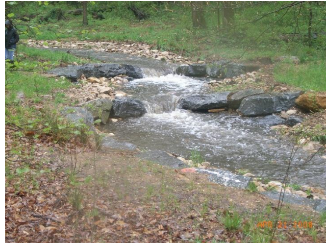
Photo 4.11 Step Pool Channel Source: Arlingtonians for a Clean Environment
