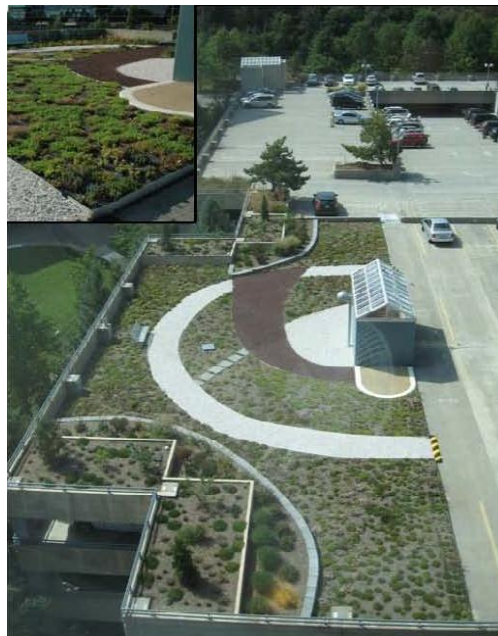
Photo 4.9 After Green Roof
