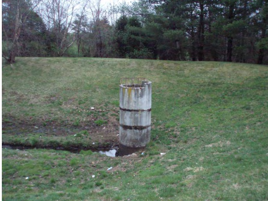
Site Photo: Existing Control Structure
