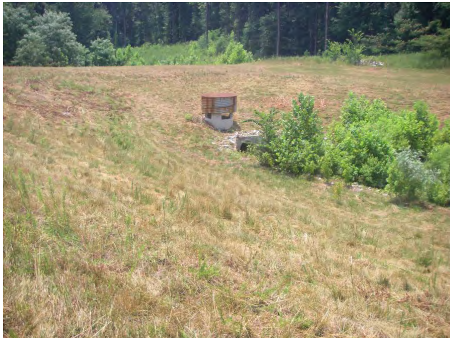
Site Photo: Existing Control Structure
