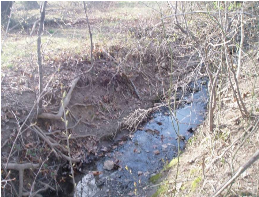
Site Photo: Erosion in Upstream Channel
