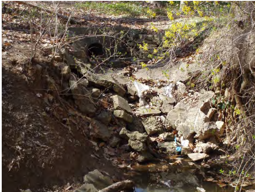
Site Photo: Storm Drain Outfall to Proposed Facility
