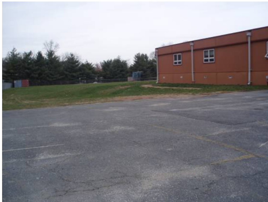
Site photo: Proposed location for a bioretention area to capture and treat parking lot runoff.
