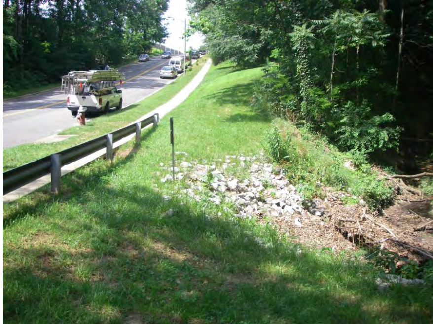
Site Photo: Existing Facility Embankment
