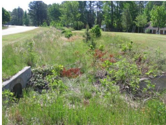
Figure 4-13: Vegetated swale for roadside drainage (Source: KCI)
