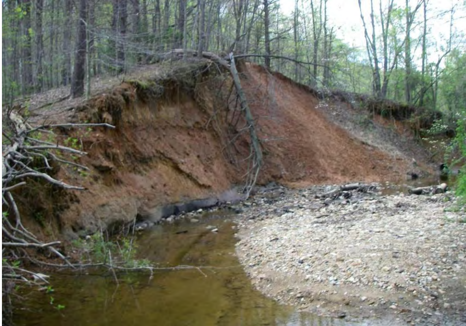
Site Photo: Severe bank erosion
