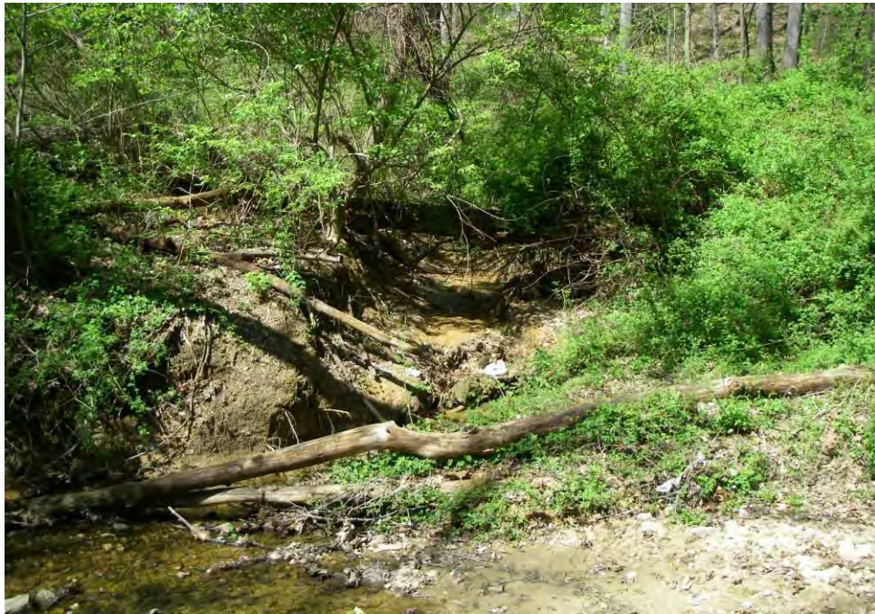
Site Photo: Eroded ditch paralleling Little River Turnpike
