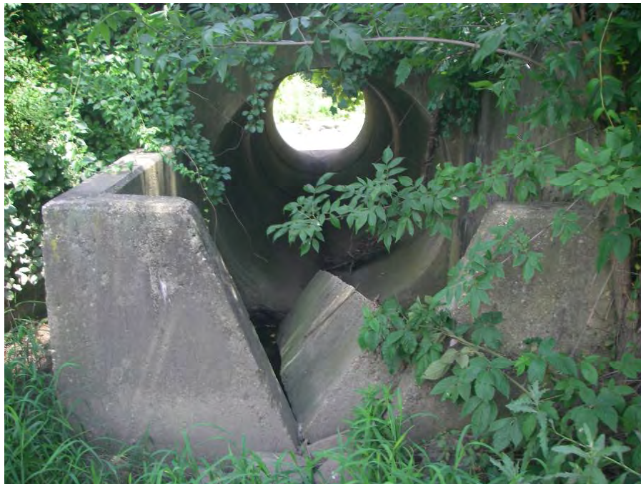
Site Photo: Existing Control Structure
