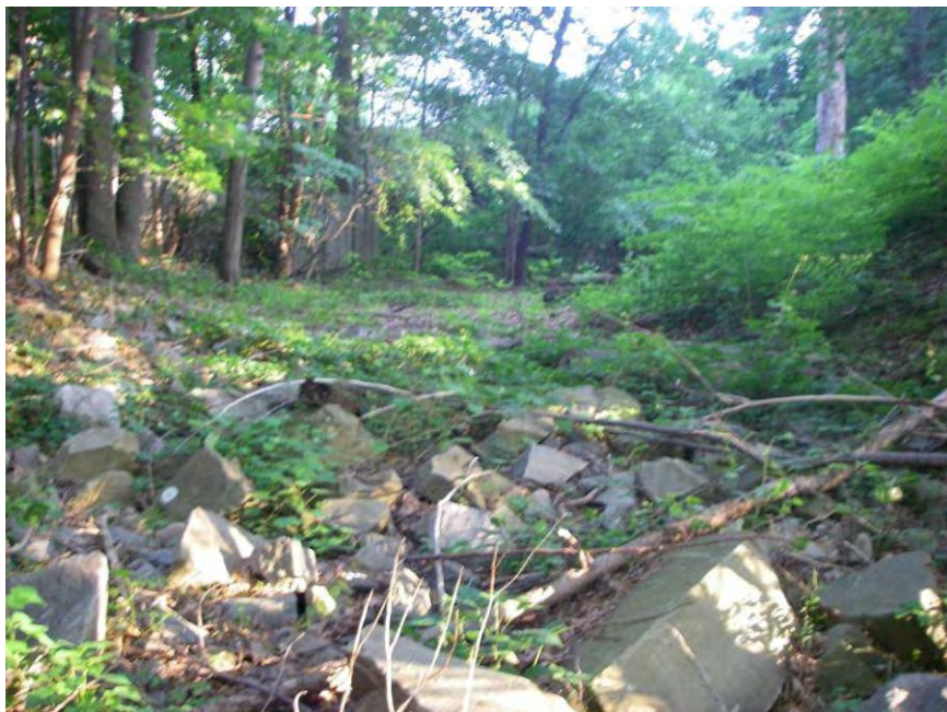
Site Photo: Existing Facility Overview (AC9175B)
