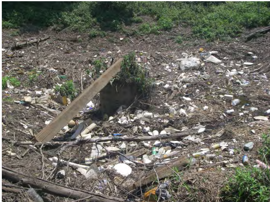
Site Photo: Existing Control Structure
