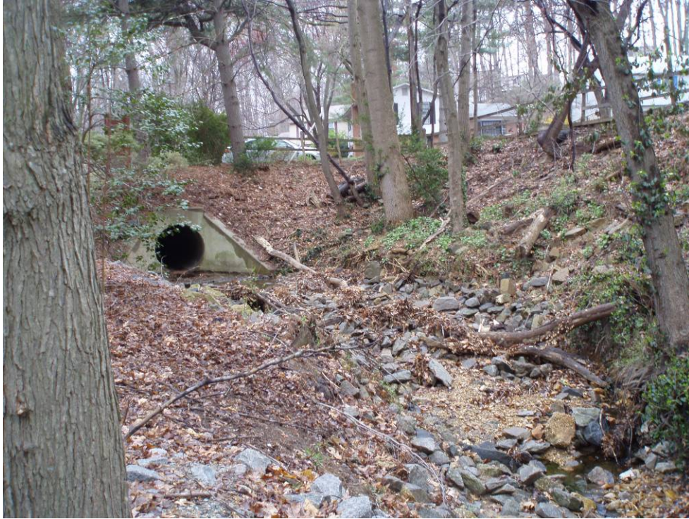
Site Photo: Existing Control Structure
