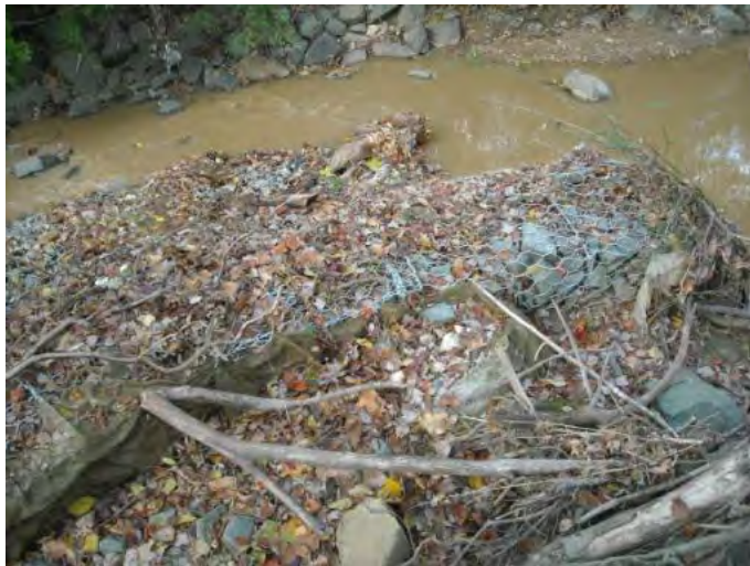
Figure 2: Existing gabion baskets within the channel
