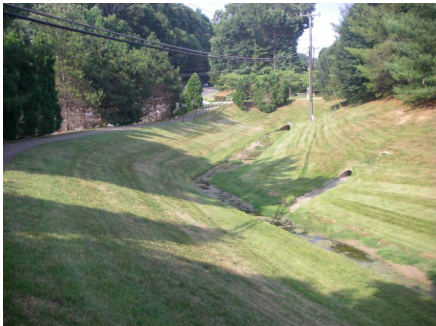
Site Photo: Existing Facility
