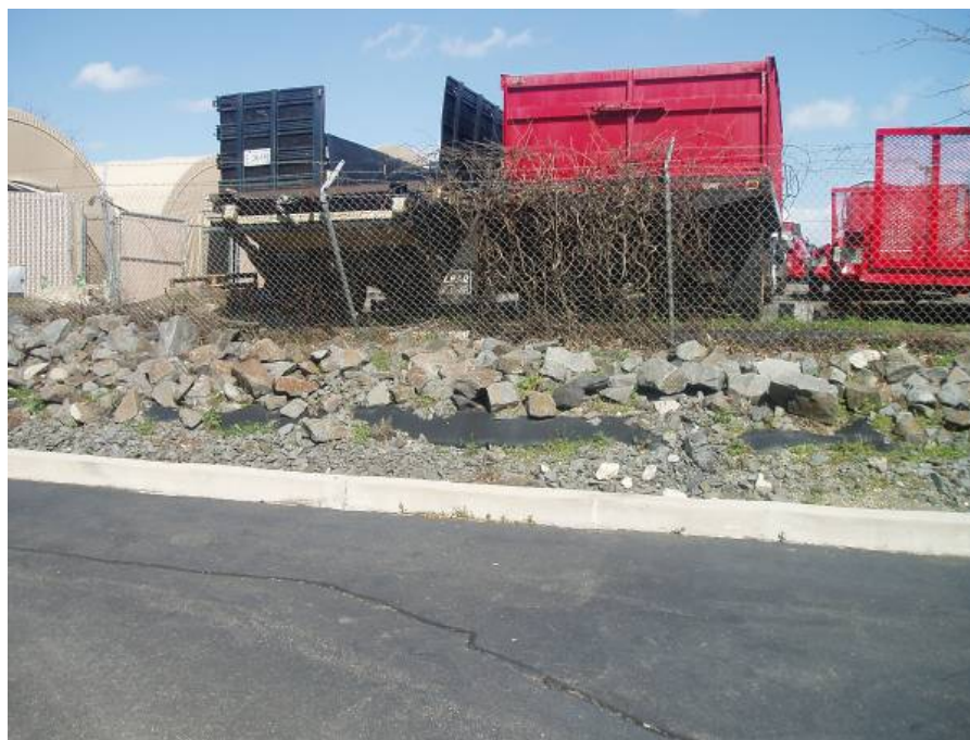
Site photo: AC9550A, near location of proposed sand filter.
