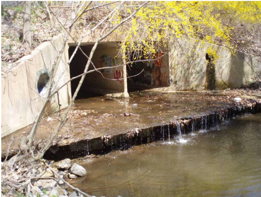
Site Photo: Downstream Side of Existing Culvert Crossing
