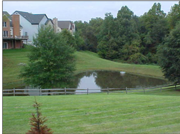
Figure 4-2: Stormwater Management wet pond (Source: Fairfax County)
