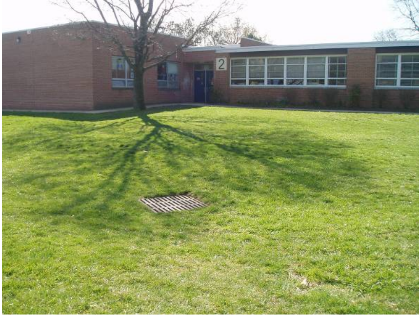
Site photo: Catch basin in field that includes rooftop connections.
