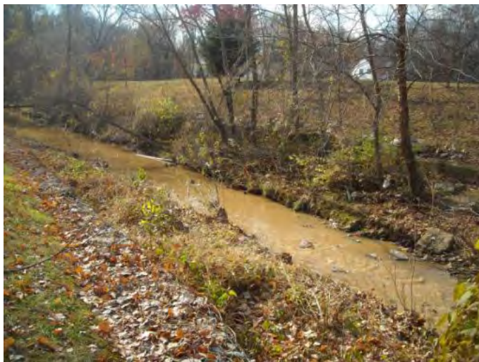
Figure 3: Existing stabilized channel with gabion banks
