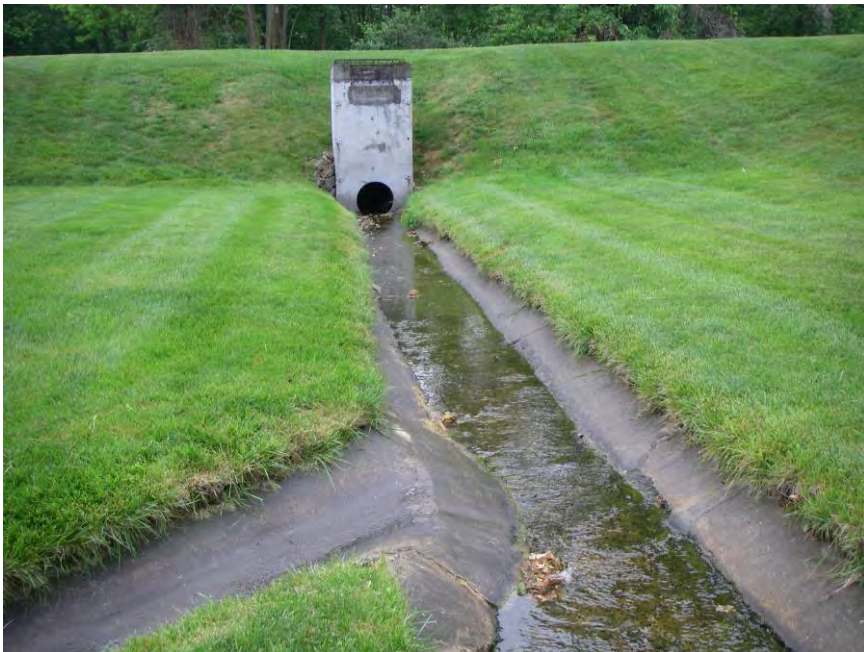
Site Photo: Existing Control Structure and Concrete Low Flow Channels
