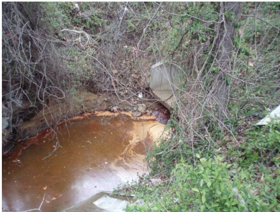
Site photo: Outfall to existing channel
