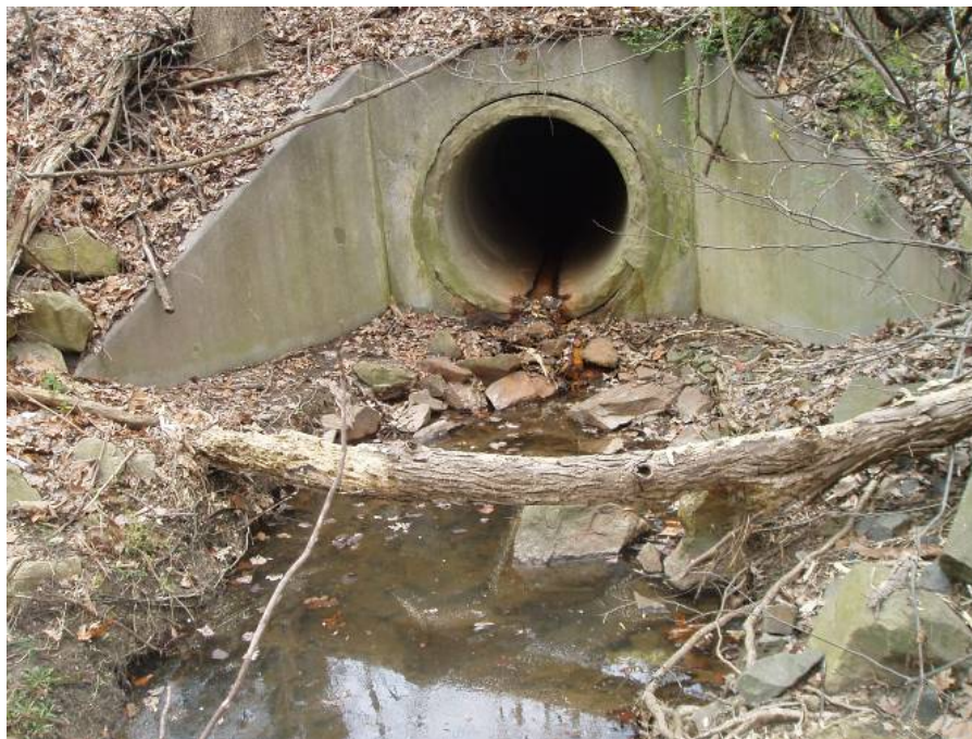
Site photo: Outfall to project area
