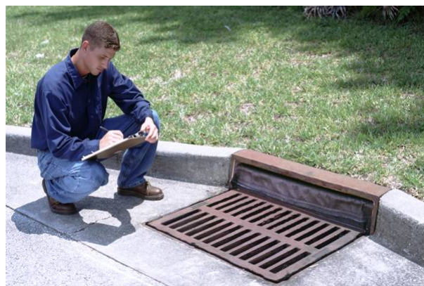
Figure 4-14: Inlet filter (Source: Ultra-Tech Int'l)
