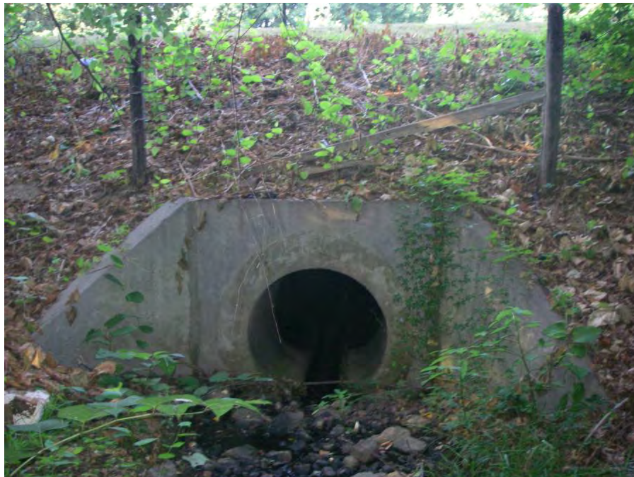
Site Photo: Existing Control Structure
