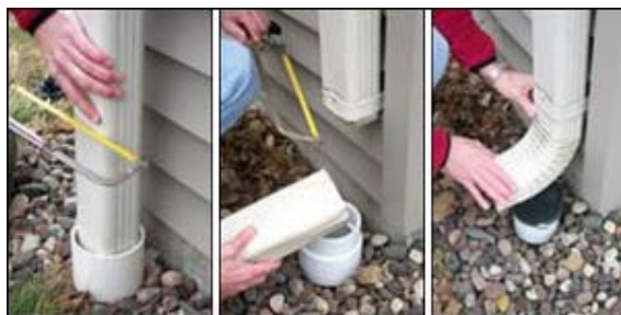
Figure 4-20: Disconnecting a downspout (Source: City of Toronto)
