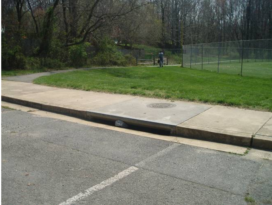
Site photo: Bioretention filter project location for AC9545A.
