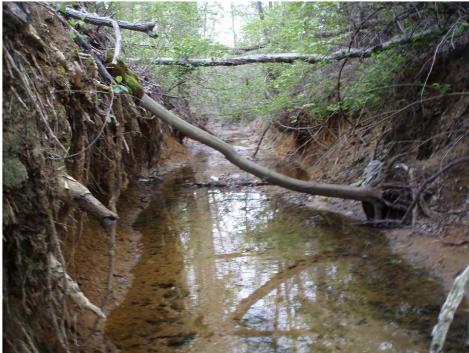
Figure 2: Incised and eroded stream channel along I-66
