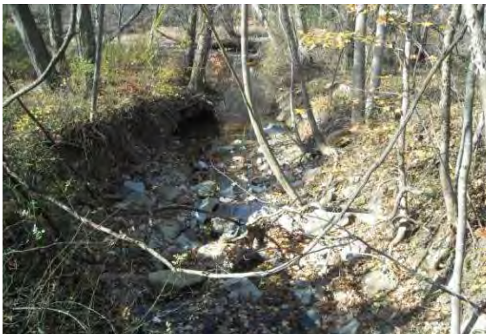
Figure 1: Incised channel with severe bank erosion
