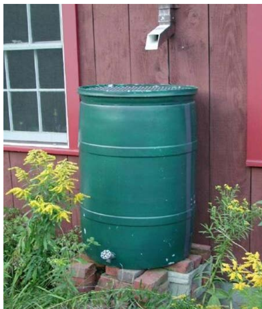
Figure 4-19: Rain barrel (Source: Project Clean Water)
