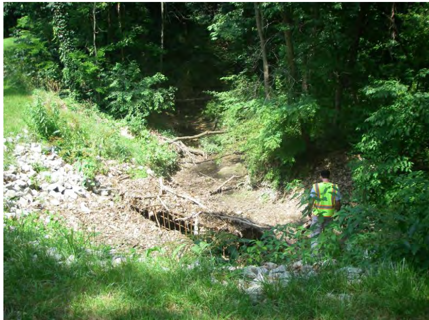
Site Photo: Existing Facility and Control Structure
