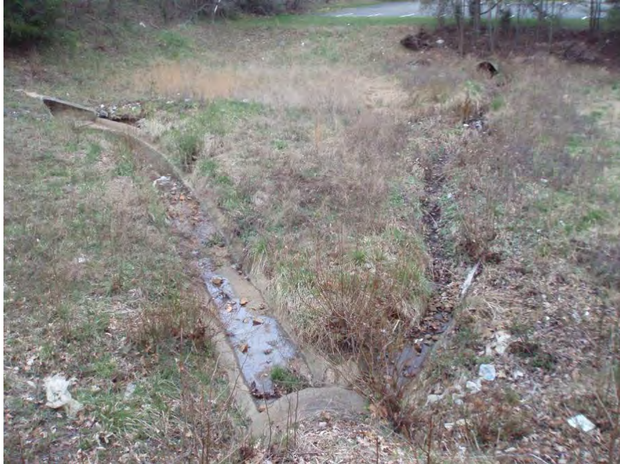
Site Photo: Existing Facility and Concrete Low Flow Channels
