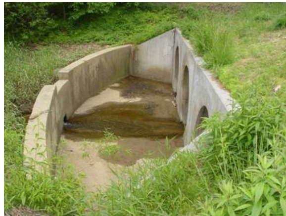
Figure 4-5: Culvert retrofit control structure, flow left to right (Source: KCI)
