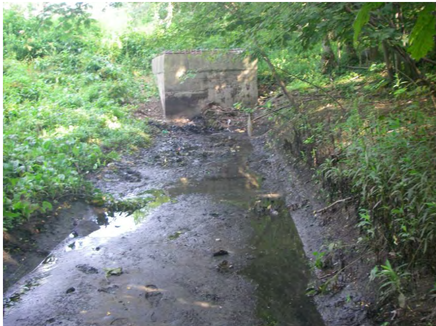
Site Photo: Concrete Low Flow Channel and Control Structure
