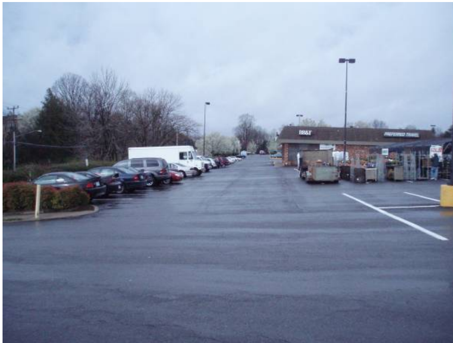
Site photo: Parking lot runoff could be treated by replacing end parking spaces with a bioretention filter.
