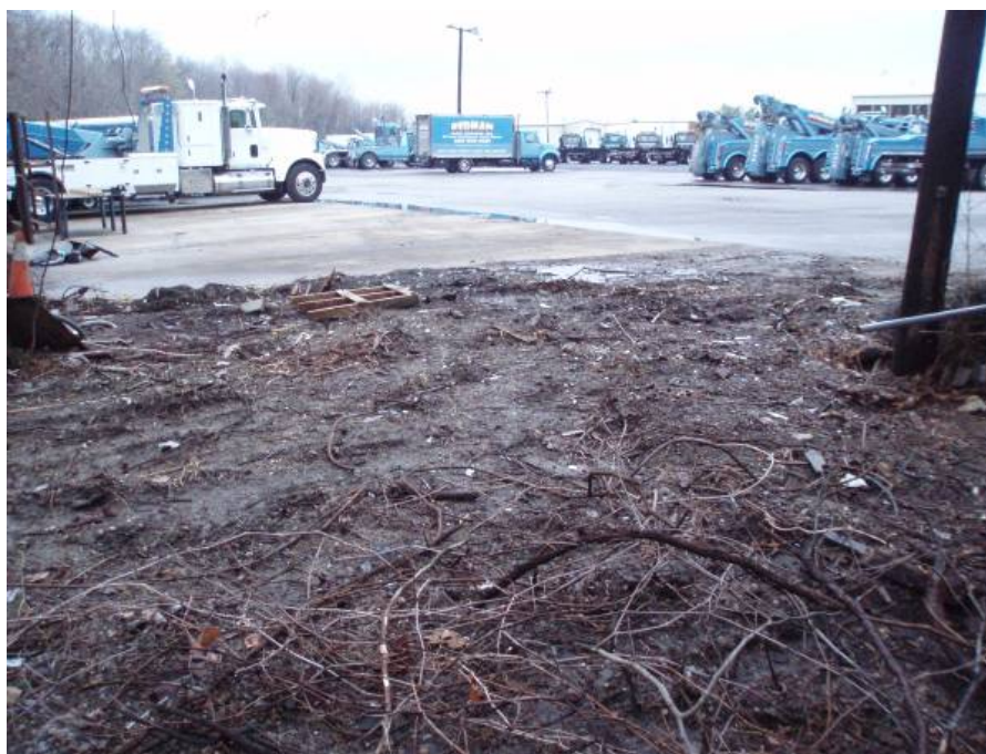
Site photo: Discharge point from parking lot where the bioretention facility could be installed.
