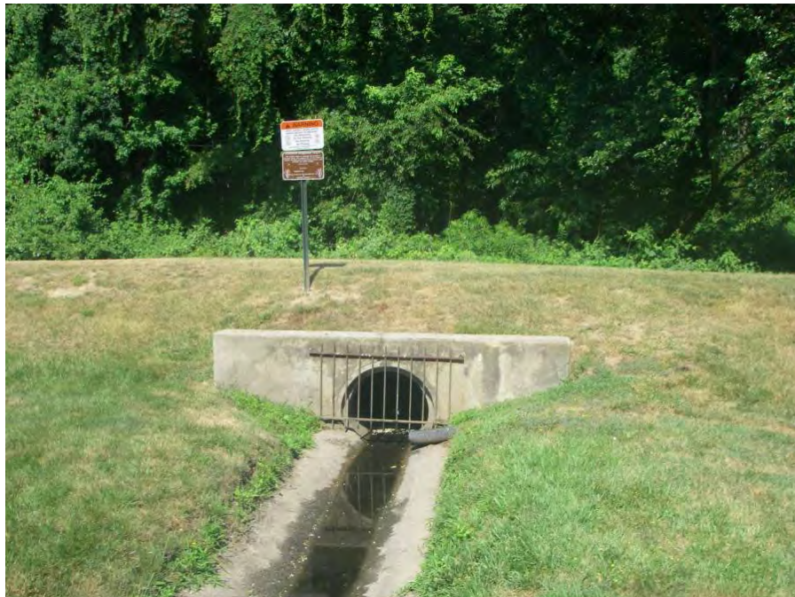
Site Photo: Existing Control Structure
