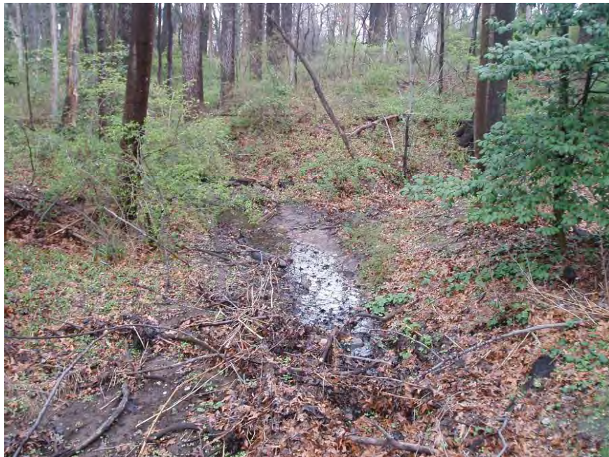
Site Photo: Existing Channel Into Flood Control Structure
