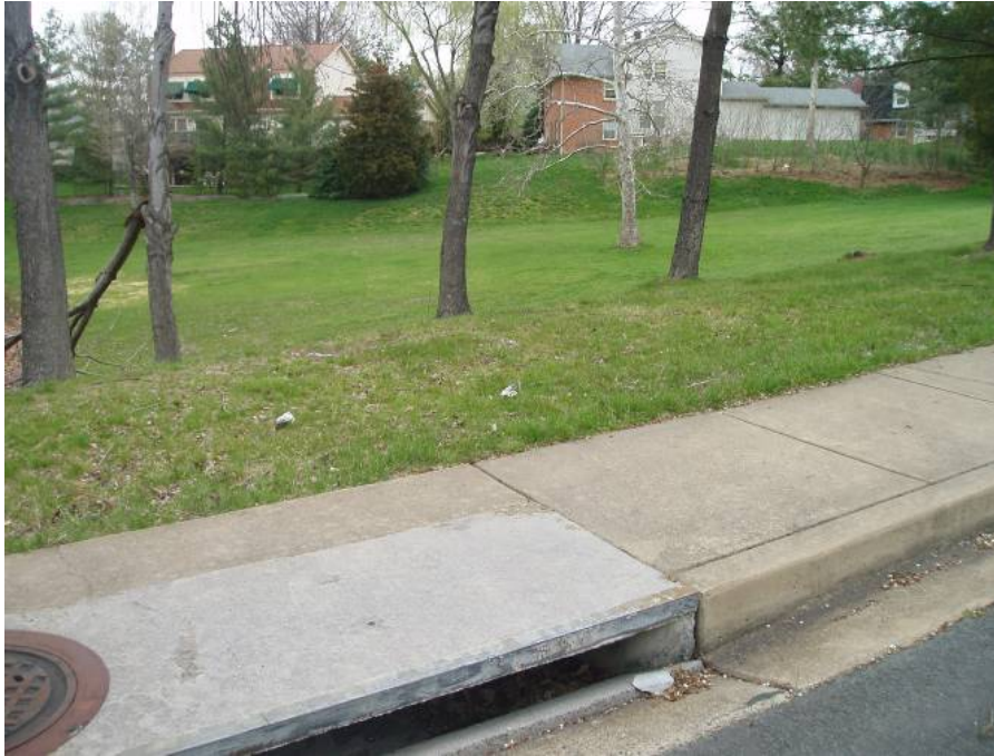
Site photo: Project area viewed from Frontage Road.
