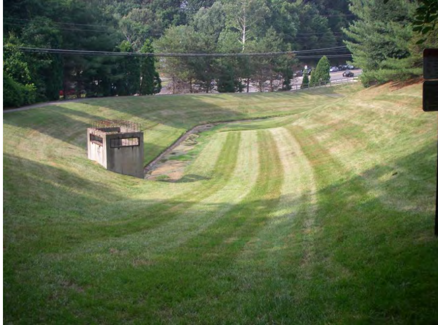
Site Photo: Existing Facility and Control Structure
