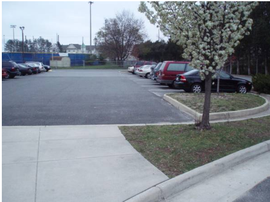
Site photo: Parking spaces to be removed for bioretention facility.
