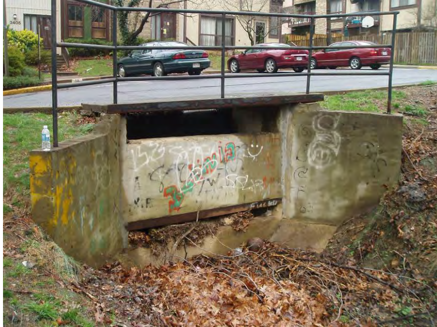
Site Photo: Existing Flood Control Structure
