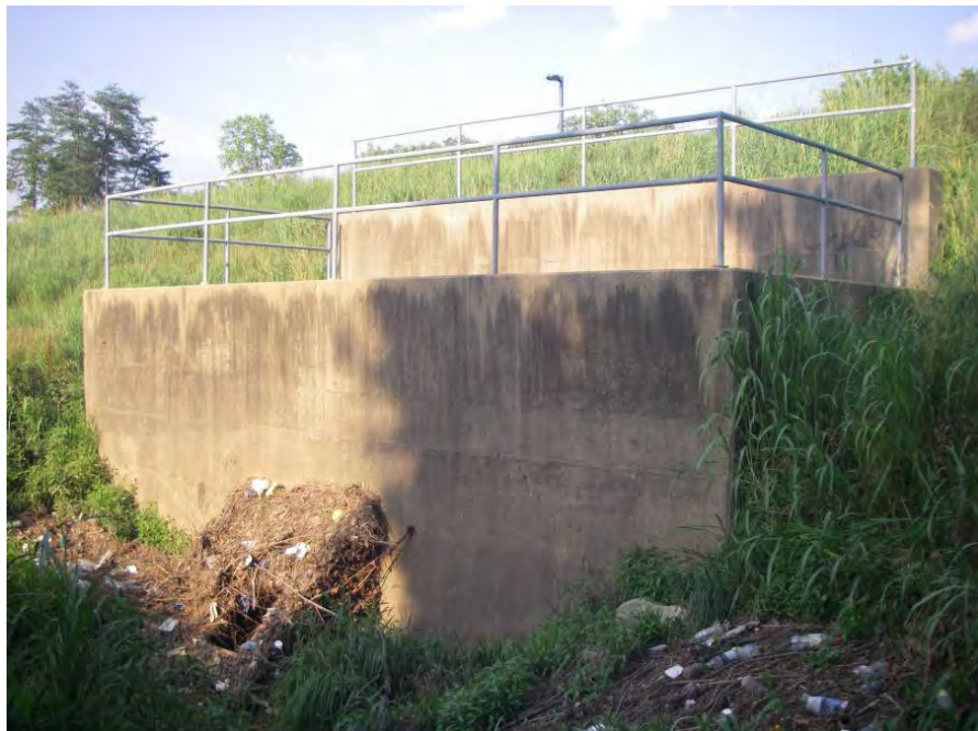
Site Photo: Existing Control Structure
