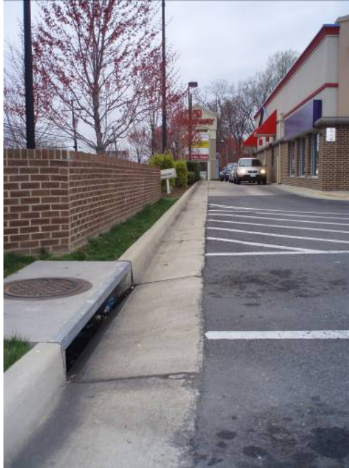
Site photo: Existing storm drain on site.
