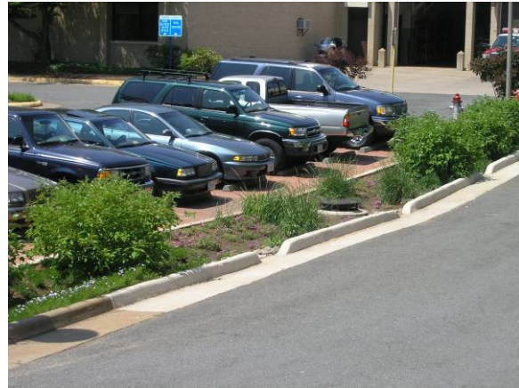
Figure 4-7: Parking lot bioretention (Source: Fairfax County)
