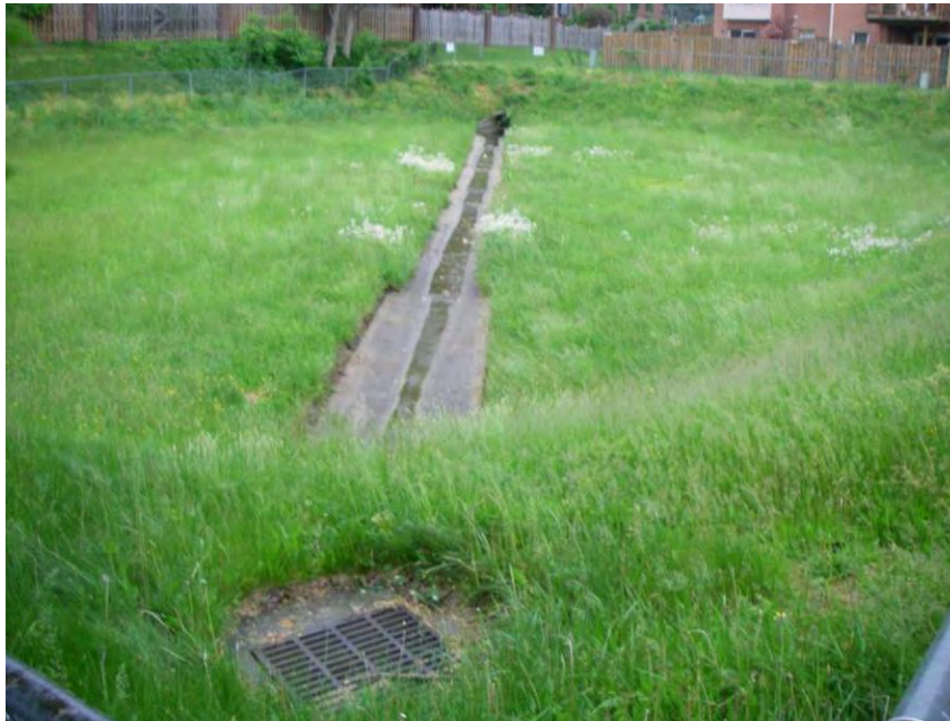
Site Photo: Existing Facility Inflow and Control Structure
