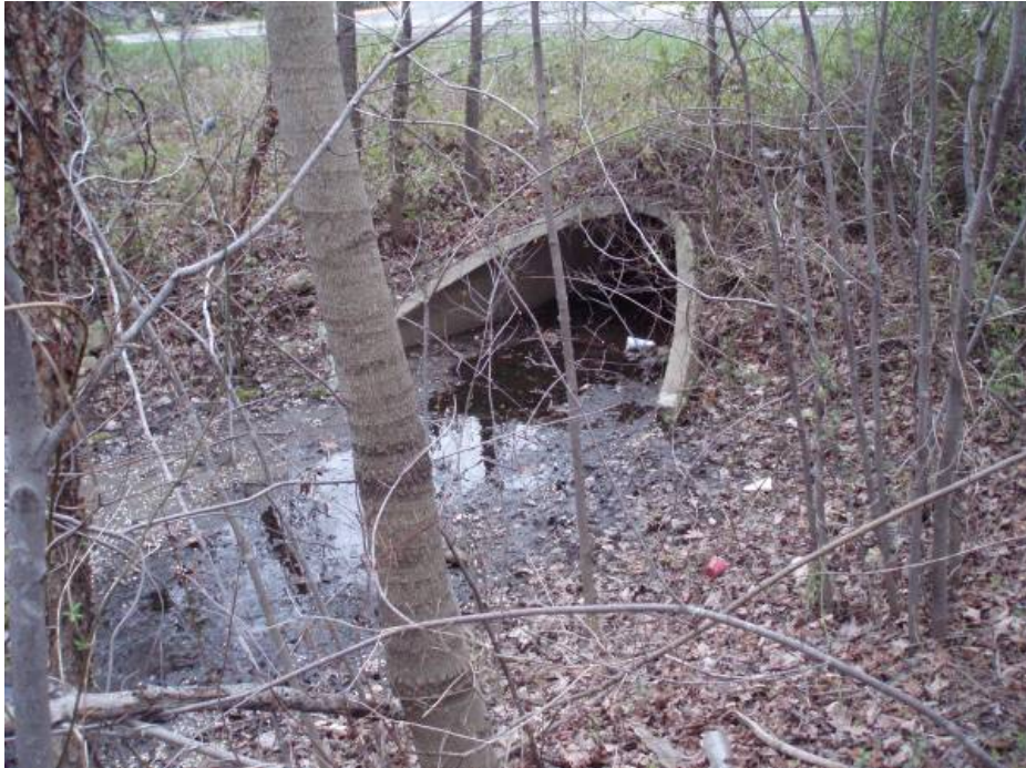
Site photo: Outlet of storm drainage system on east side of Newington Road.
