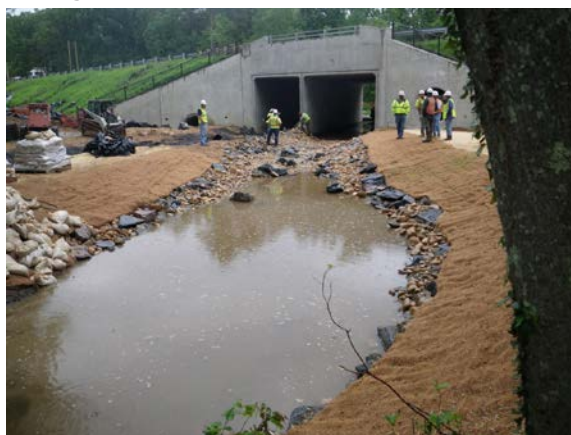
Figure 4-16: New replacement culvert (Source: KCI)
