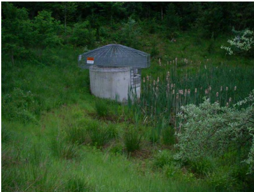
Site Photo: Existing Control Structure
