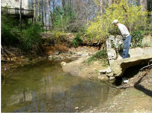
Site Photo: Downstream end with severe erosion and impacts to walking trail/storm drain inflow
