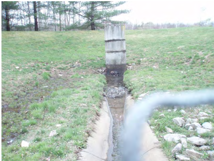
Site Photo: Concrete Low Flow Channel and Embankment
