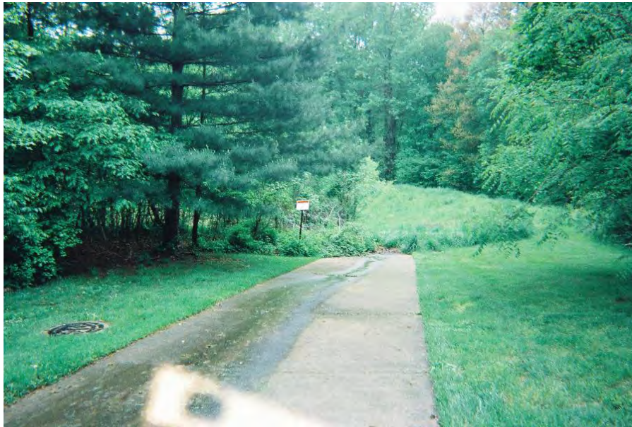
Site Photo: Facility Inflow and Overall Facility
