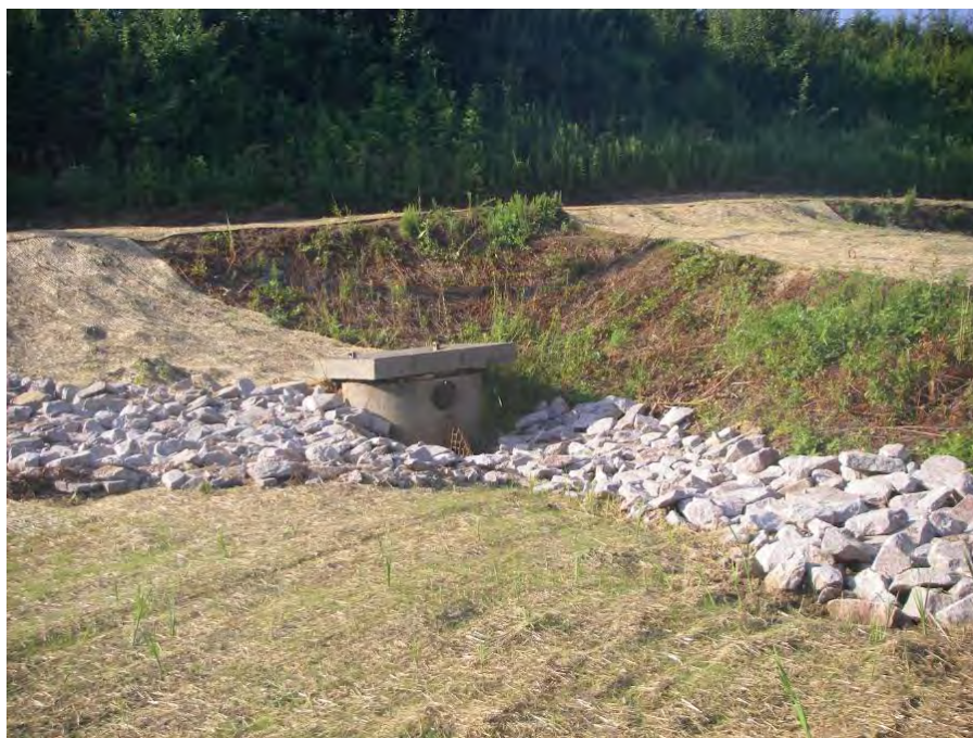
Site Photo: Existing Control Structure
