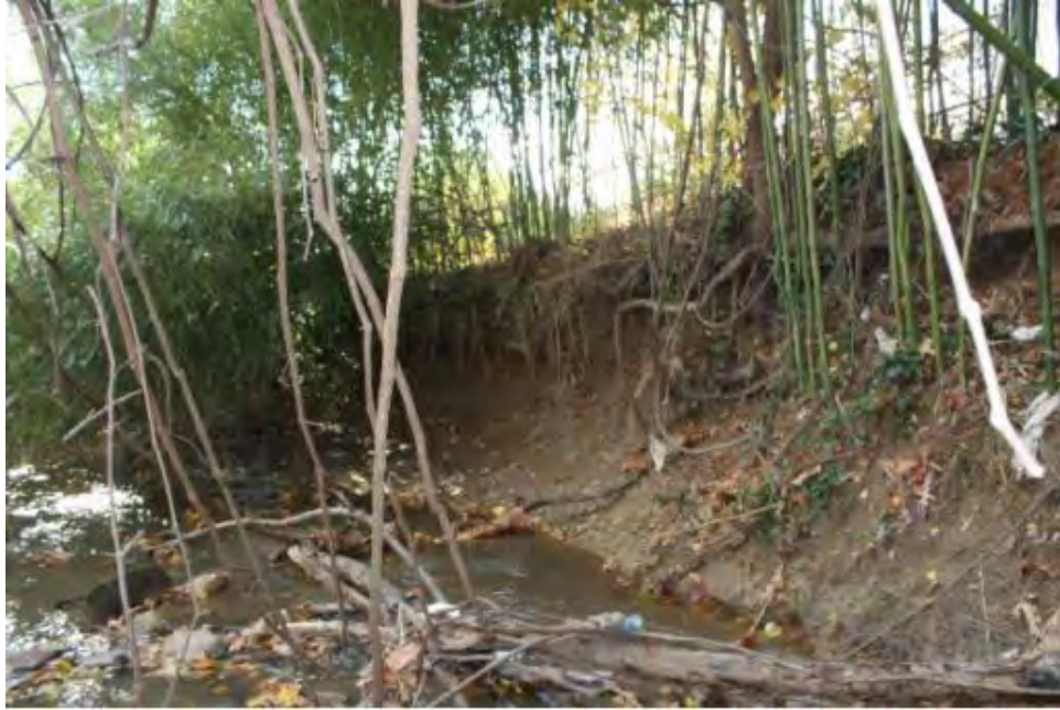
Figure 1: Severly eroded banks with invasive bamboo
