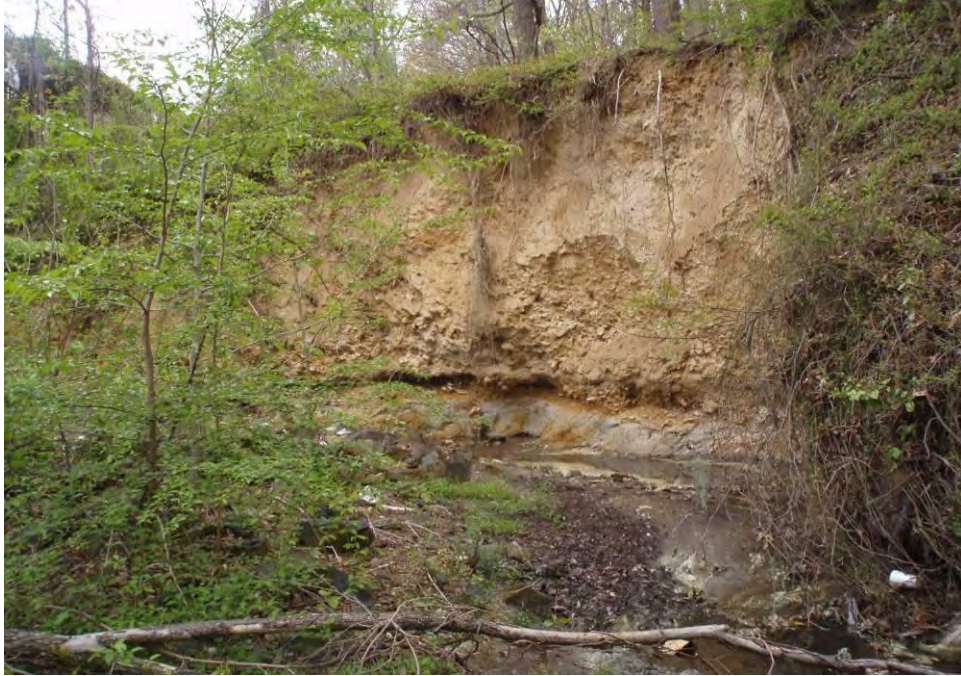
Site Photo: Severe bank erosion in upstream portion
