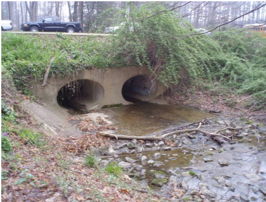
Site Photo: Existing Culvert
