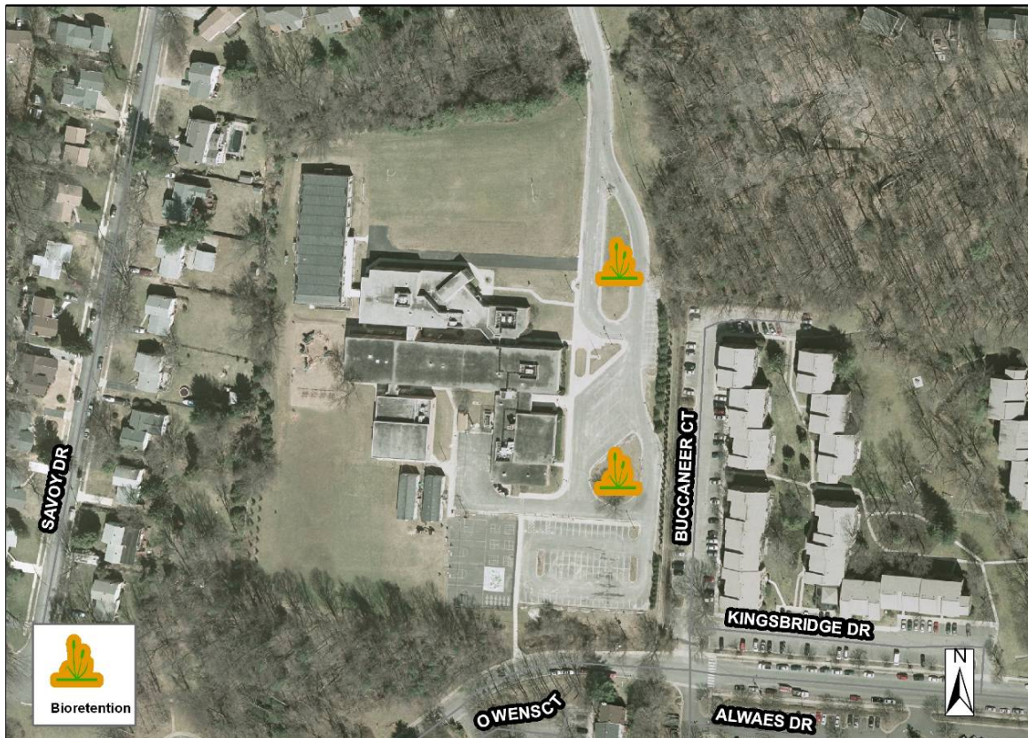
Site Photo: Parking lot island where bioretention facilities can be located.
