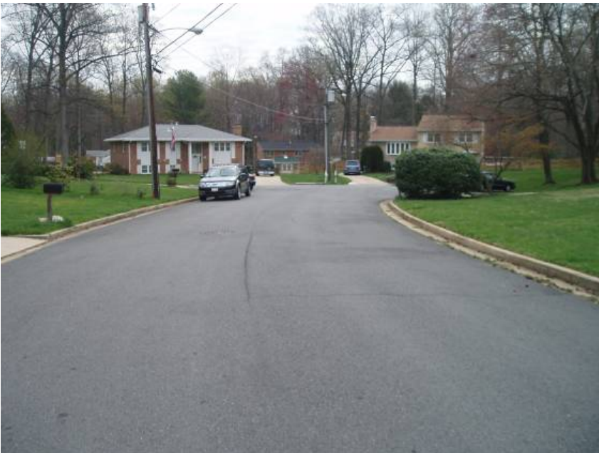
Site photo: Cul-de-sac with space for curb extension at site AC9547B
