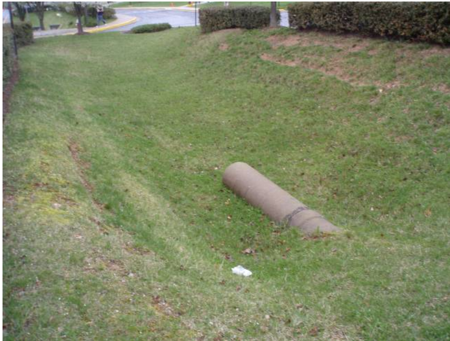
Site photo: Another existing dry pond located in a parking island..
