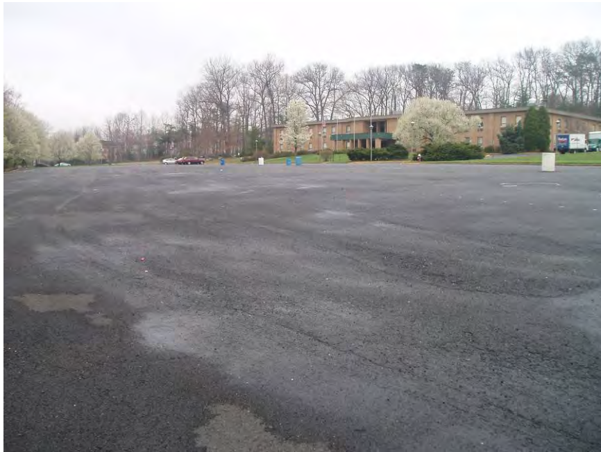
Site Photo: Existing Parking Area
