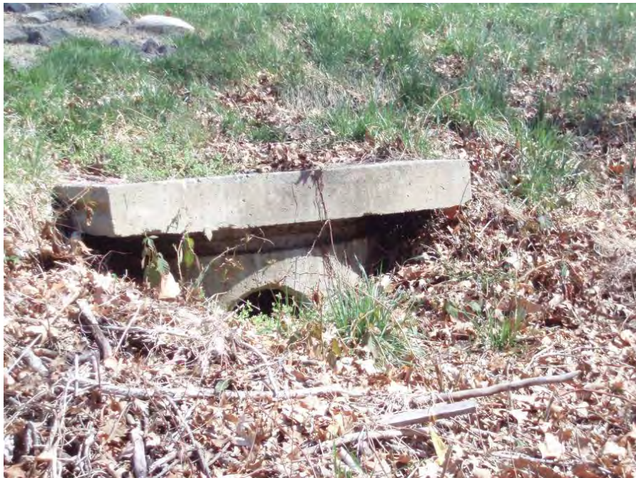
Site Photo: Existing Control Structure
