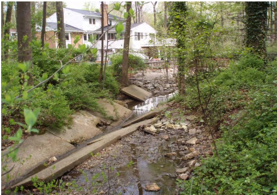
Site Photo: Concrete/rip rap in downstream portion
