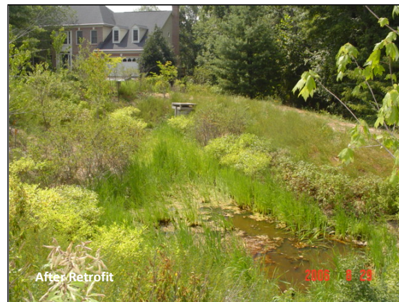
Figure 4-3: Stormwater dry pond retrofit (Source: Fairfax County)
