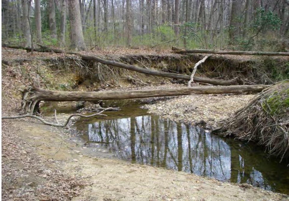
Site Photo: Incised channel with severe meander bank erosion
