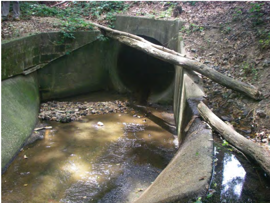
Site Photo: Existing Control Structure
