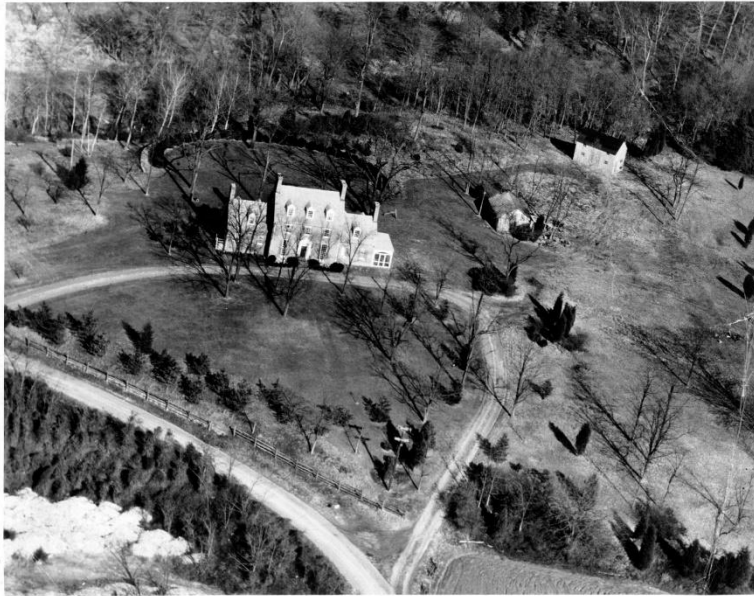
Figure 53: Straight-Era Aerial Photograph Showing Entrance Drive
