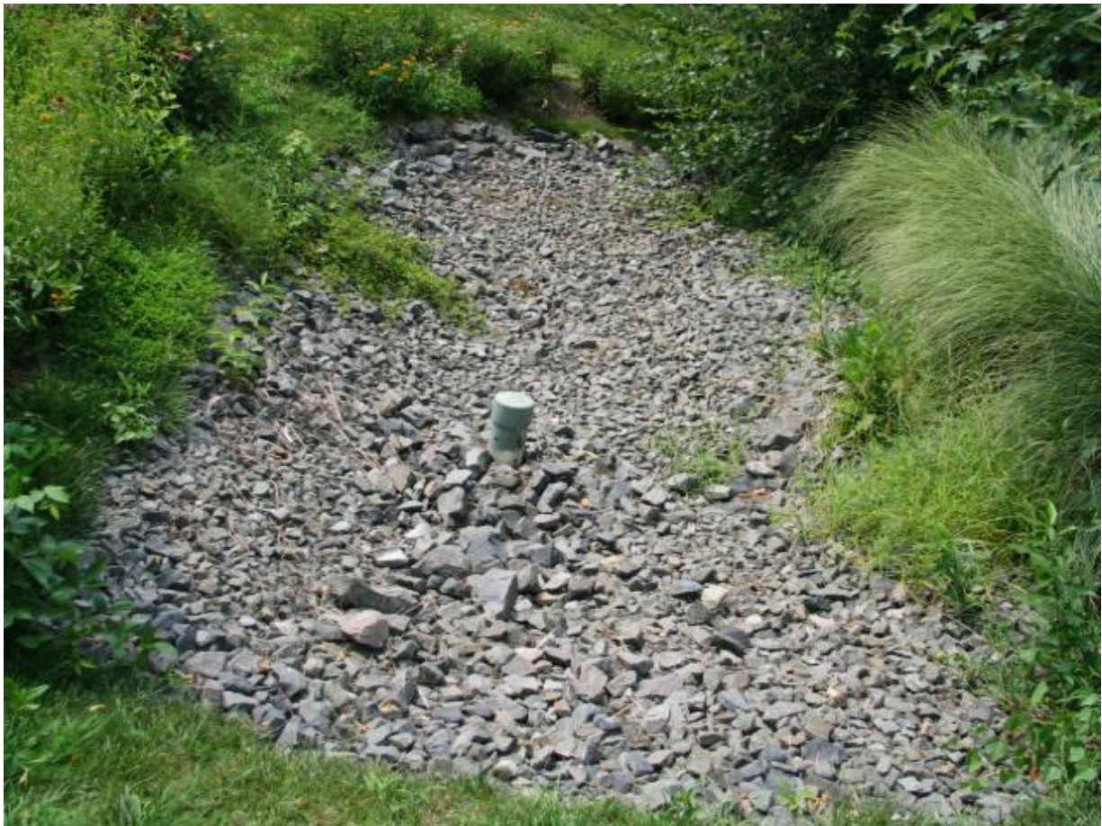
Fig. 8: Example of a modified forebay where a perforated observation well has been added (RG-20)
