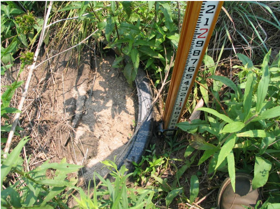
Fig. 7: Example of a modified rain garden where ponding area is directly connected to the gravel sump through a sand column
