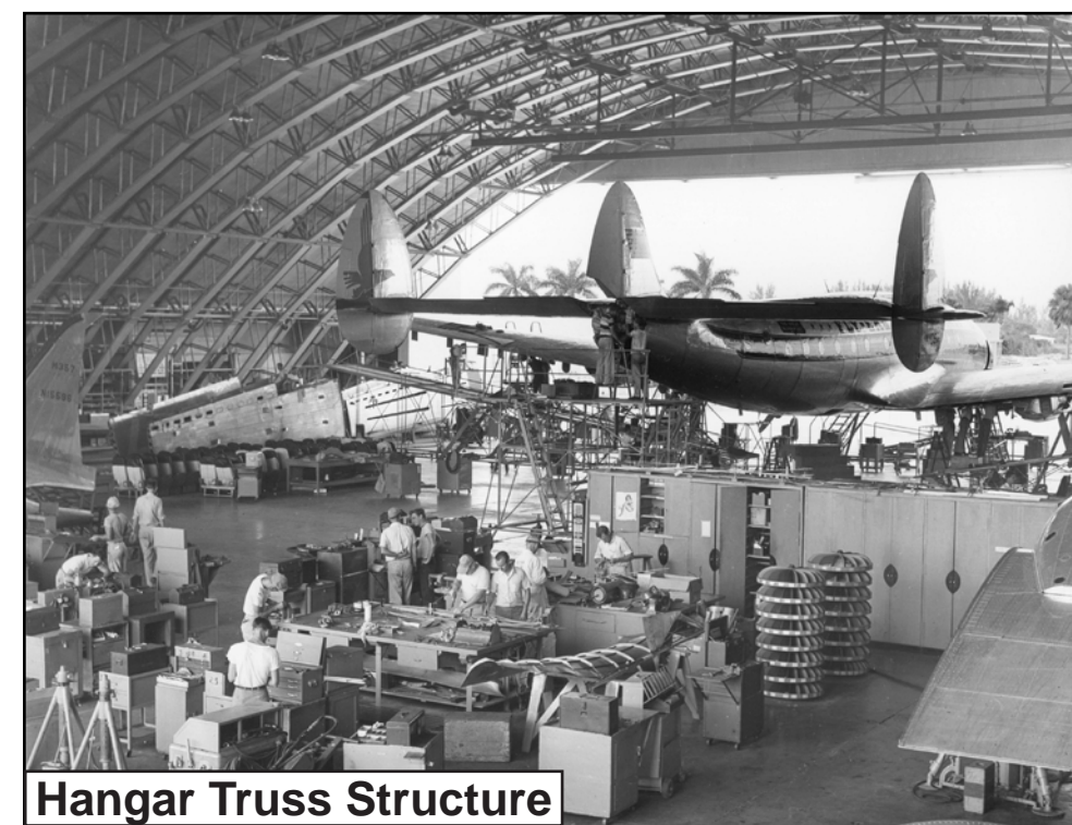
Hangar Truss Structure
